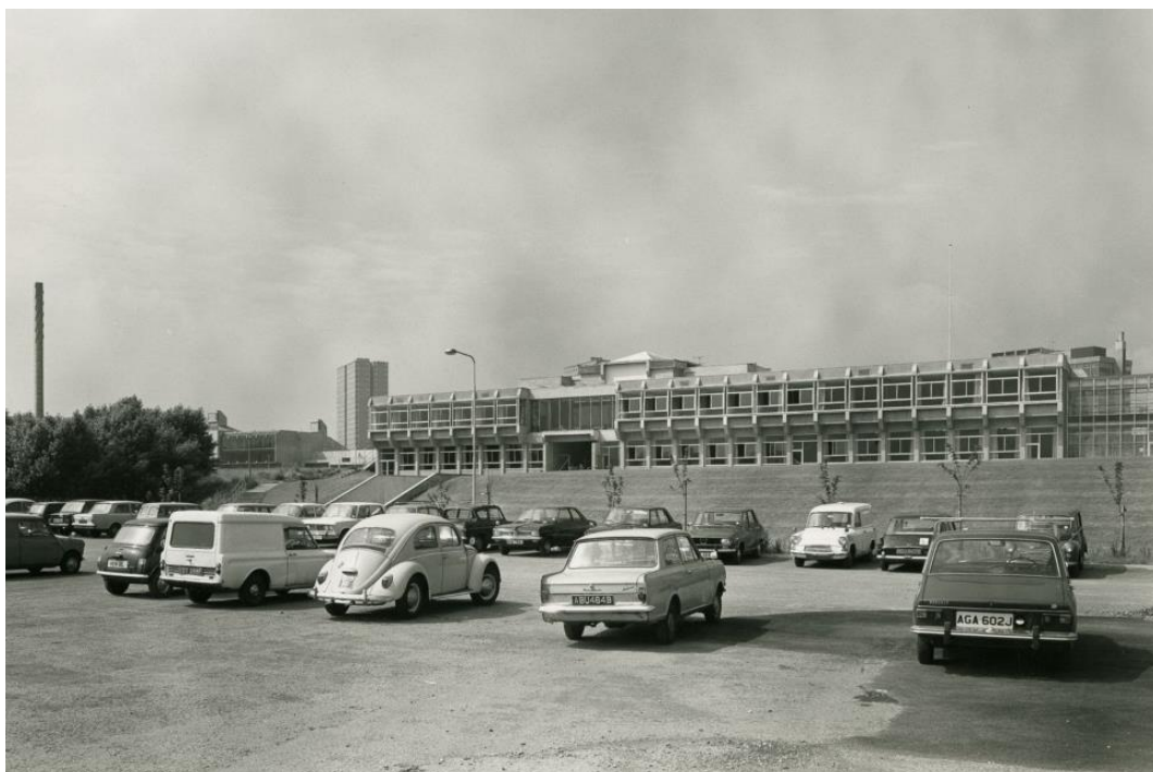
Figure 98: University House (University of Salford, c1970). North car park.
