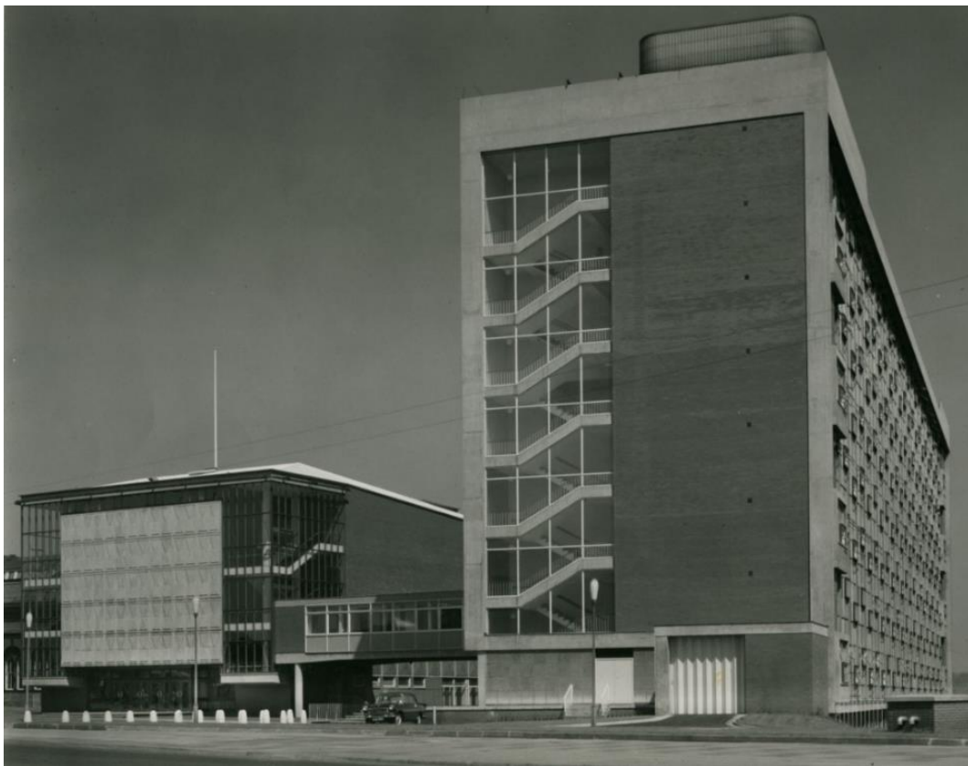
Figure 59: The Maxwell Building and Hall (Royal College of Advanced Technology Salford, c1960c).
