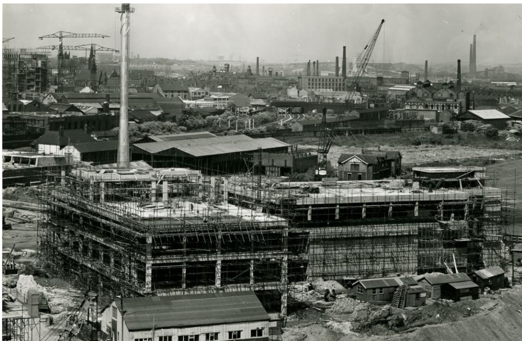
Figure 81: Construction of Cockcroft Building (Royal College of Advanced Technology Salford, 1965). Middle: Central Boiler Plant House. Far left: the Allerton Building under construction.
