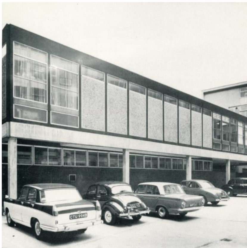
Figure 61: Computer Centre (Digital Salford, c1966). Known today as the Gilbert Rooms, the image is taken from the Maxwell Building's internal service yard and car park.
