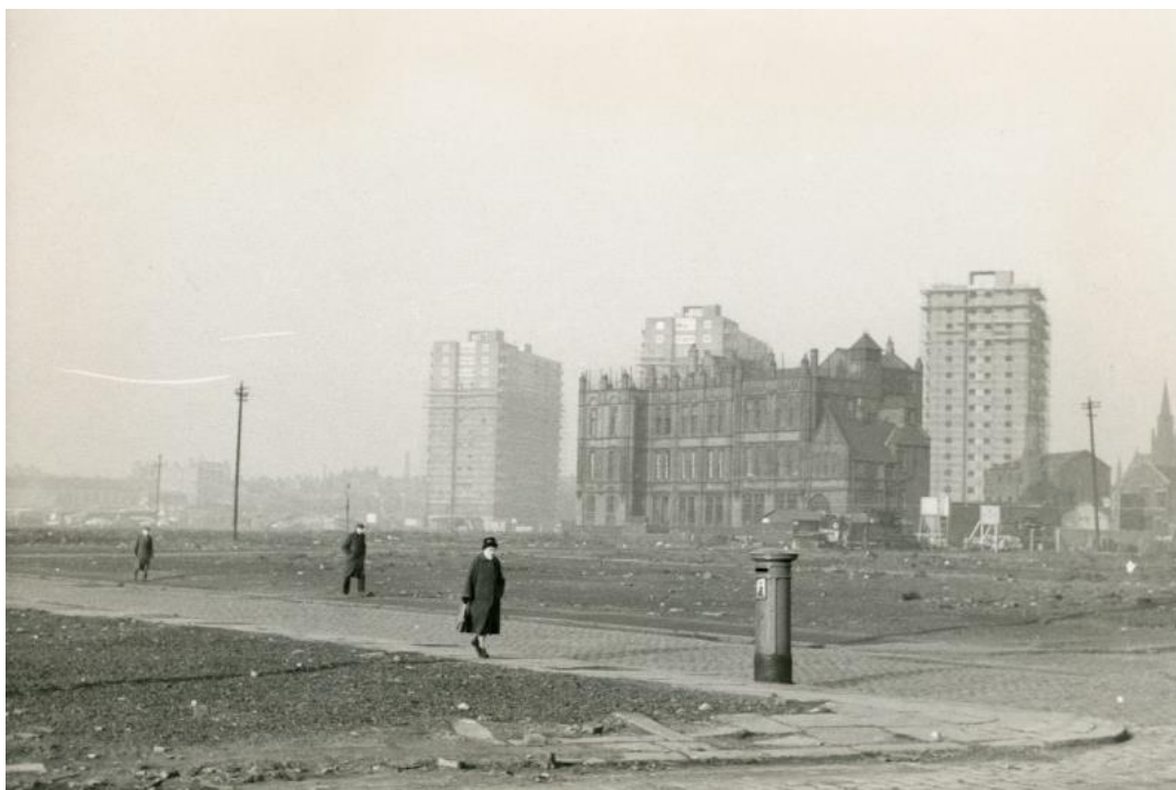
Figure 7: Pendleton (Royal College of Advanced Technology Salford, c1960d). Centre: former John Street Board School.
