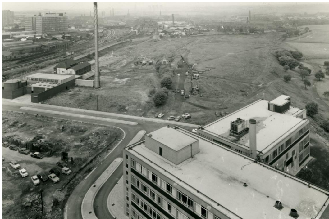
Figure 82: Cockcroft Building (University of Salford, c1970d).
