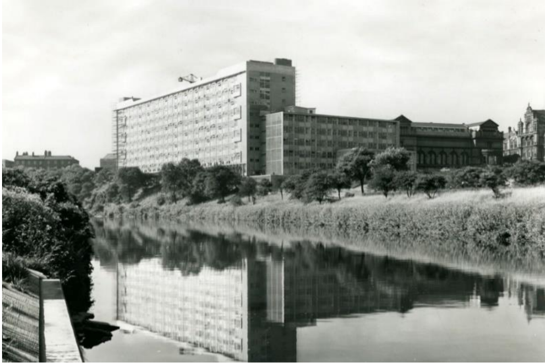
Figure 33: Maxwell Building near completion (Royal College of Advanced Technology Salford, c1959)
