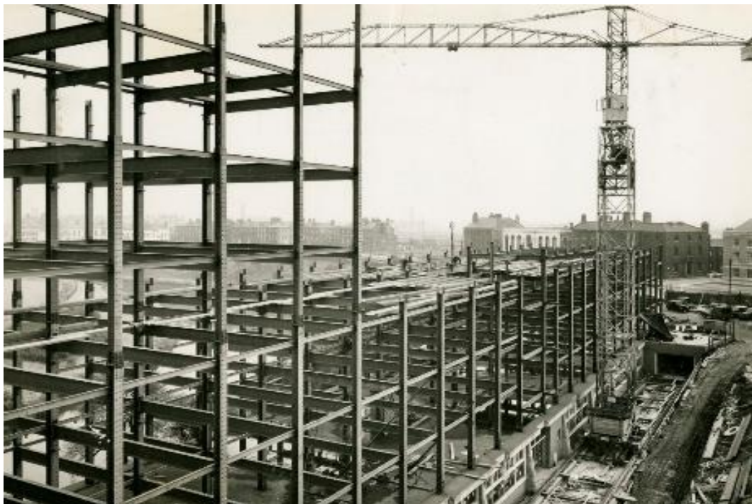
Figure 30: Maxwell Building construction (Royal College of Advanced Technology Salford, c1956). Phase I. Background: Salford Crescent.
