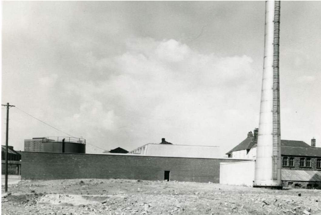
Figure 80: Central Boiler Plant House (Royal College of Advanced Technology Salford, c1963a). East elevation.
