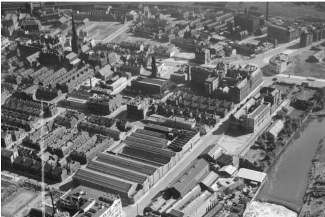
Figure 19: Proposed site (Britain from Above, 1951). Top right, the Council's proposed site. Centre: Adelphi Iron Works; bottom left: Adelphi Building.
