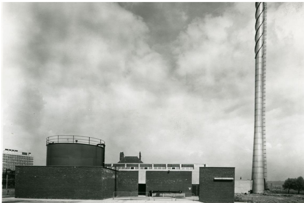
Figure 79: Central Boiler Plant House (University of Salford, c1967).
