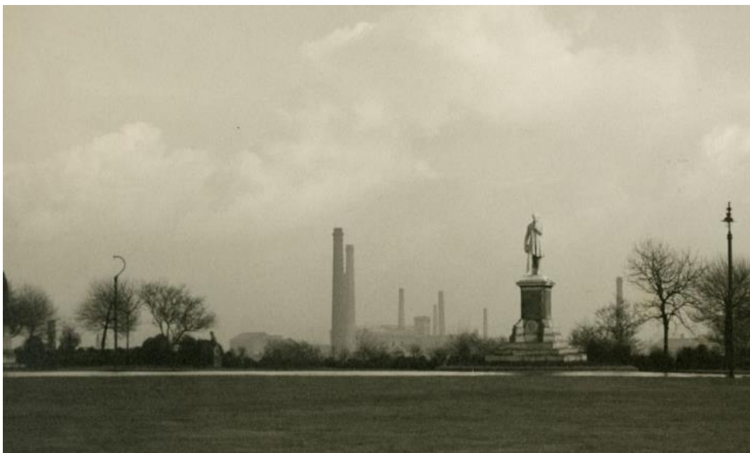
Figure 26: Pre-construction site (Royal Technical College Salford, c1950b).
