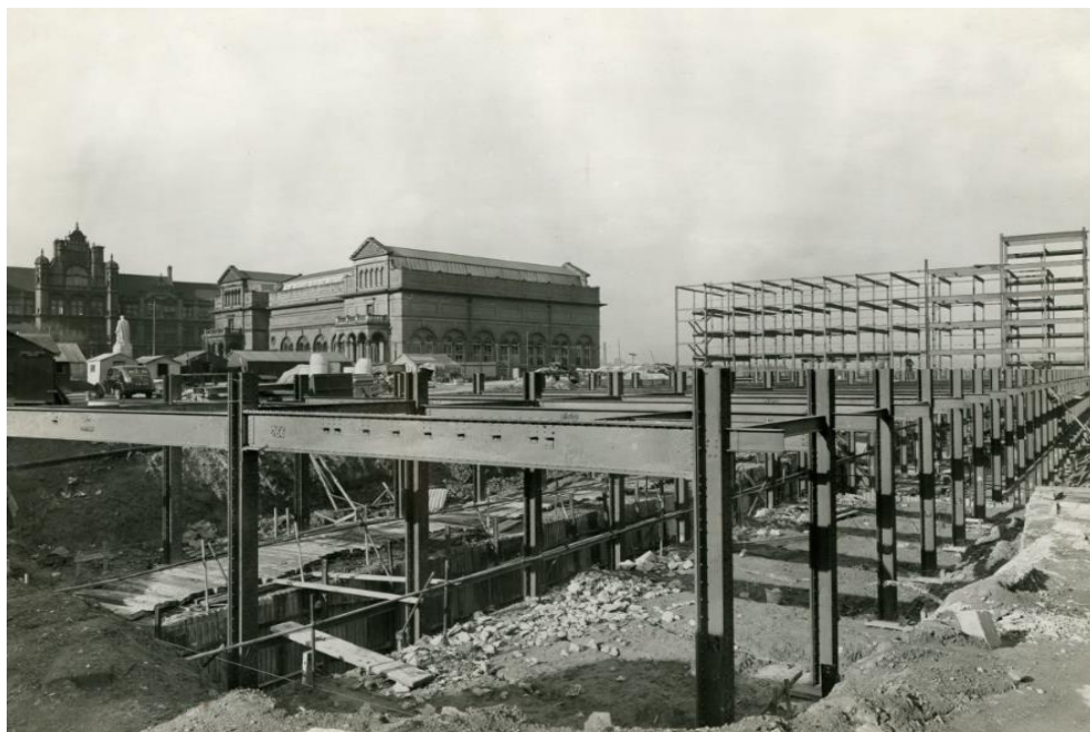
Figure 29: Construction site (Royal Technical College Salford, c1954b). Prior to the pause.
