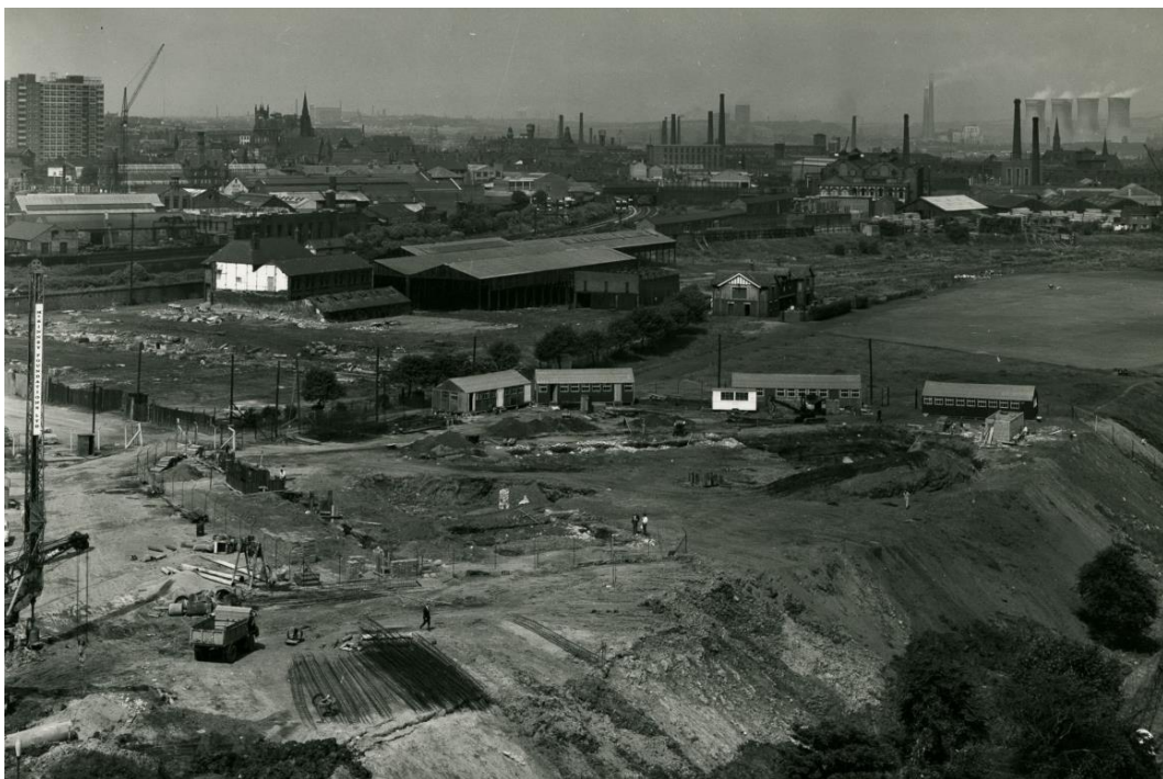
Figure 44: Cockcroft Building site (Royal College of Advanced Technology Salford, c1964a).
