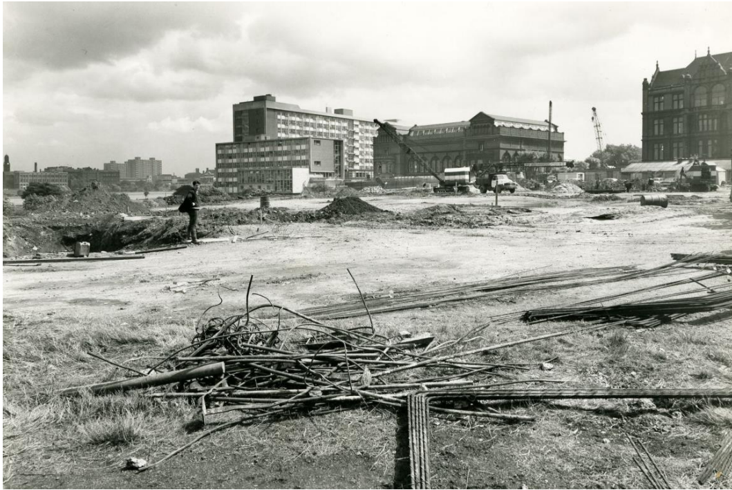
Figure 45: Site clearance ( Royal College of Advanced Technology Salford, c1964b ).
