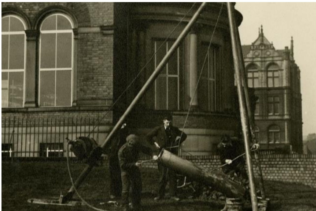
Figure 22: Peel Park site boring (Royal Technical College Salford, 1950e).
