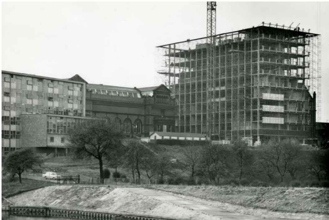
Figure 75: Chemistry Tower (Royal College of Advanced Technology Salford, c1963c). Left: the Maxwell Building smaller five story block.
