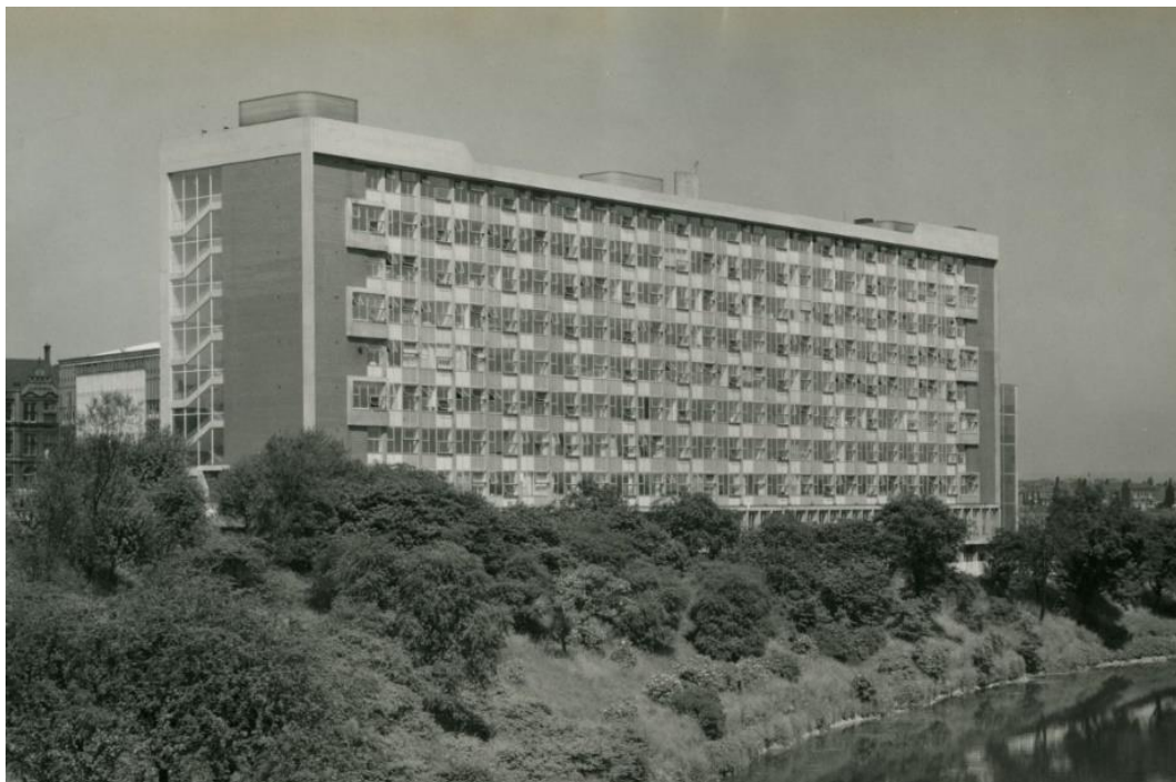
Figure 3: The Maxwell Building and Hall (Royal College of Advanced Technology Salford, c1960e).
