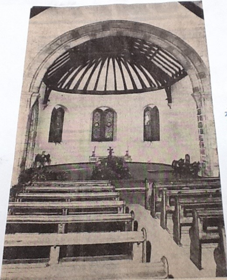
Part of the interior of St Michael's, Lancaster Moor Hospital.—L12
