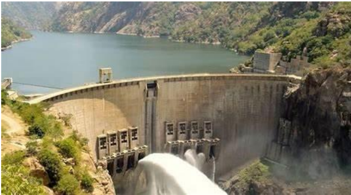
Figure 3. 11 Excess water released from Lagdo dam in Cameroon (Punch, 2022).
