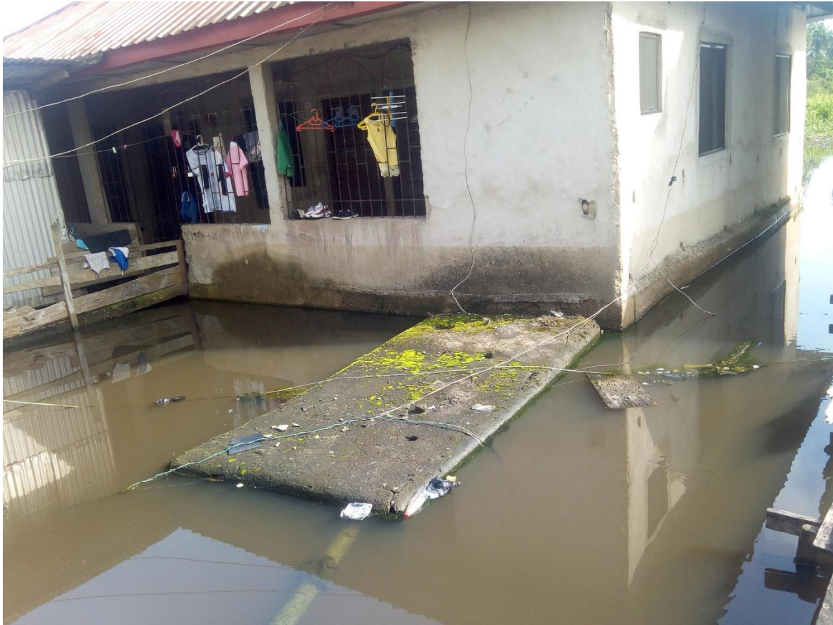
Figure 3. 12: Flood water contamination from soakaway pits.
