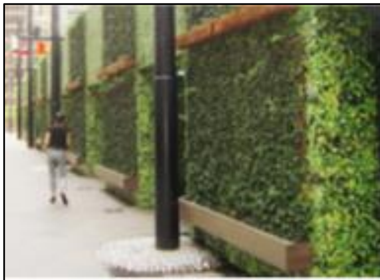
Figure 2-14: Indirect Green Façade (Source:Manso & Castro-Gomes, 2015).
