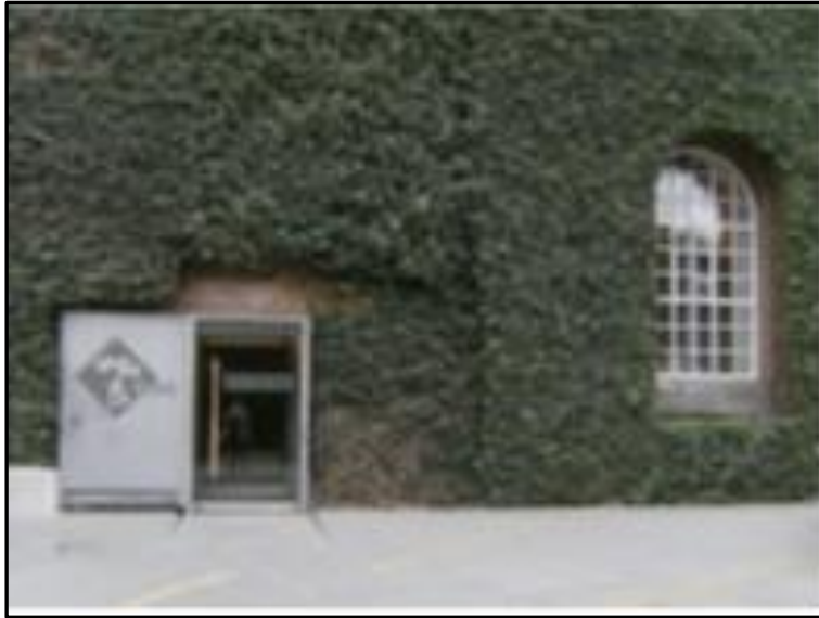
Figure 2-15: Direct Green Façade on a Private House in Golegã, Portugal (Source:Manso & Castro-Gomes 2015).
