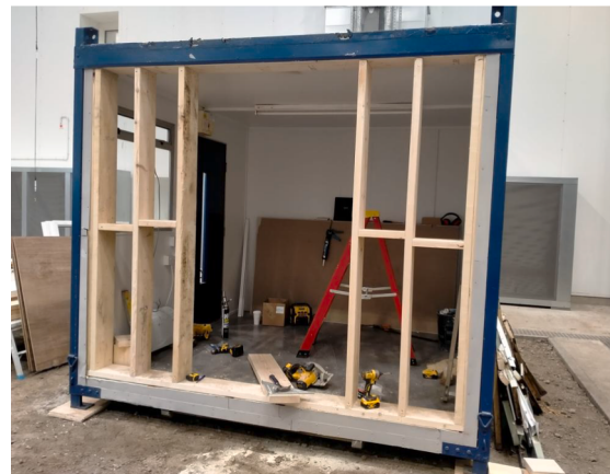
Preparation of the walls (Jan 2023)
