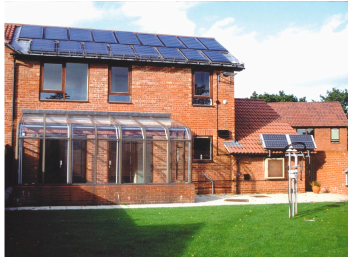
Figure 6. Solar Demonstration House in Bournville, Birmingham (see [3]).
