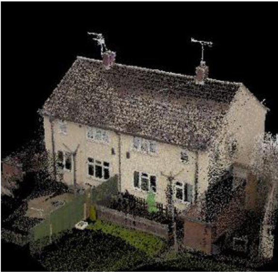
Fig. 5. 3D laser scan of the building used for off-site measurements.
