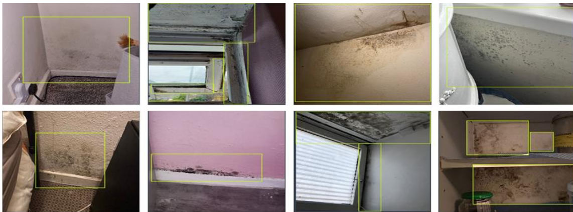
Fig. 8. Annotated and Preprocessed Mould Detection Dataset. This figure displays the result of preprocessing the dataset for training the mould detection model. Bounding boxes (rectangles) are drawn around individual patches of mould (object detection task) within the images. Since some images contain multiple areas of mould, several bounding boxes might be present. It's important to note that the images might have undergone preprocessing steps before this annotation stage.
