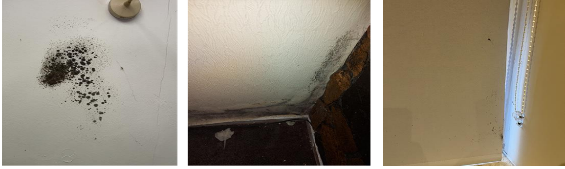
(a) Sample images containing different mould patterns on the wall
