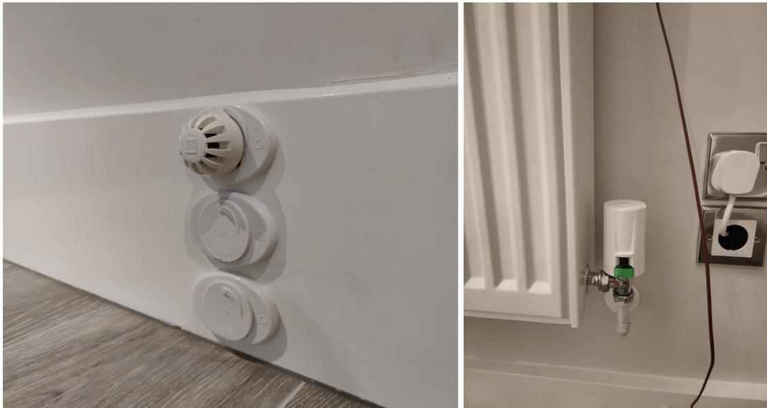
Figure 12. ThermaSkirt control (left) and radiator TRV (right)
