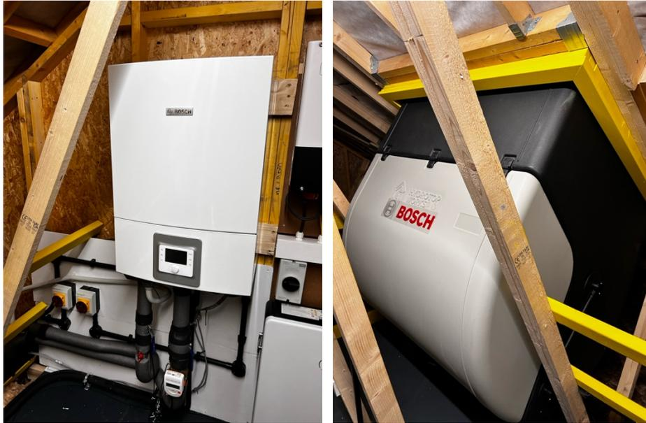
Figure 171. Indoor and outdoor unit located in roof space
