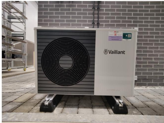
Figure 8. Vaillant ASHP External Unit
