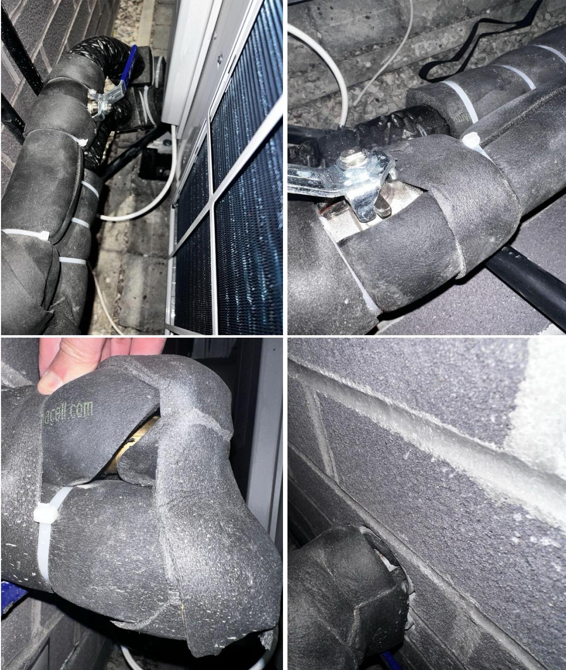
Figure 167. Poor insulation practice externally to the ASHP flow & return pipes
