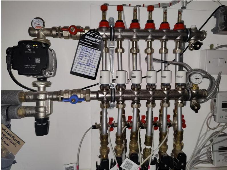
Figure 4. Underfloor heating manifold
