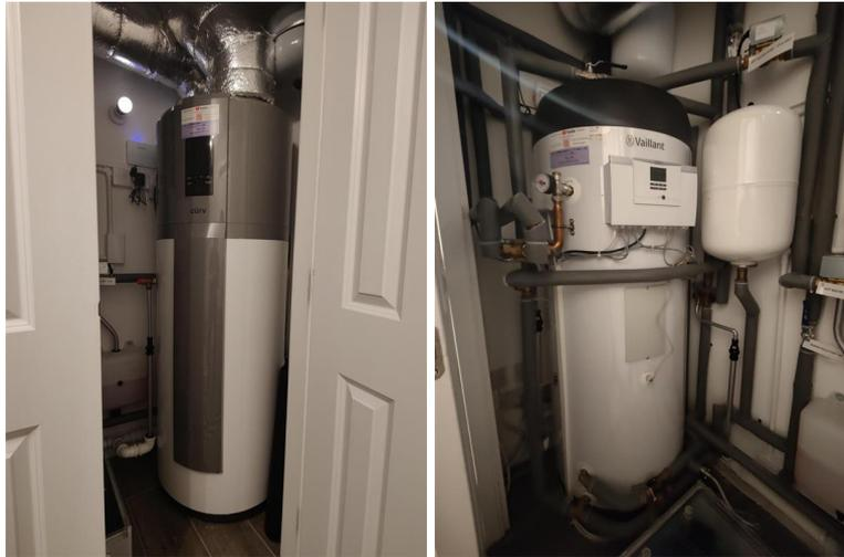
Figure 13. Curv hot water cylinder (left) and Vaillant ASHP cylinder (right)
