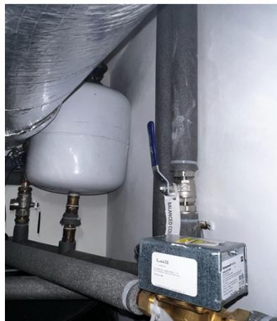
Figure 170. Uninsulated volumizer/solar safety vessel
