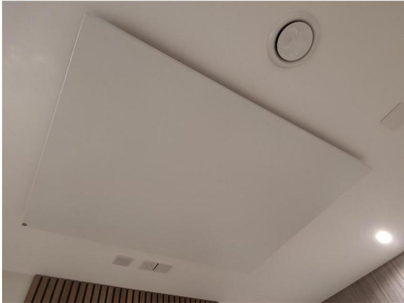
Figure 5. Wondrwall infrared panel
