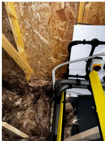
Figure 175. Waste pipe to dispose condensate located in the roof space
