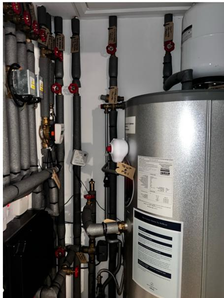
Figure 172. Cylinder without TMV protection
