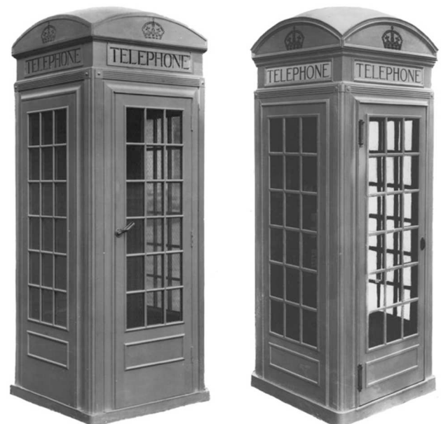
Figure 7. Differences between Sir Giles Gilbert Scott's original design (left) and the finalised design (right) adopted by the GPO as the K2 (courtesy of BT Group Archives images TCB 417/E 3092 and E 3363).
