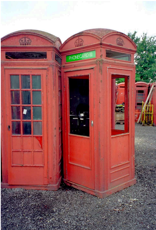
Figure 12. Two K2s located at Unicorn Restorations showing the extreme anti-vandal modifications that had been carried out prior to their ultimate demise (photograph taken 29 September 1999).
