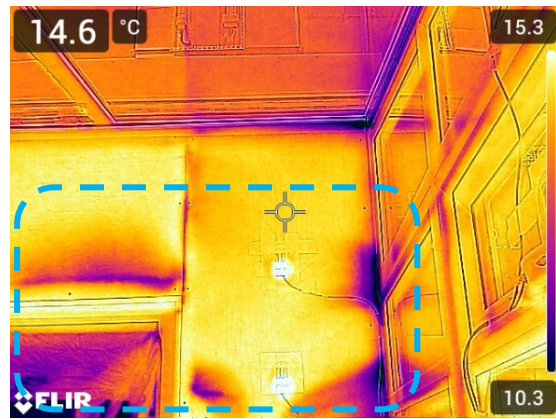
Figure 16 Insulation Under Depressurisation Test
