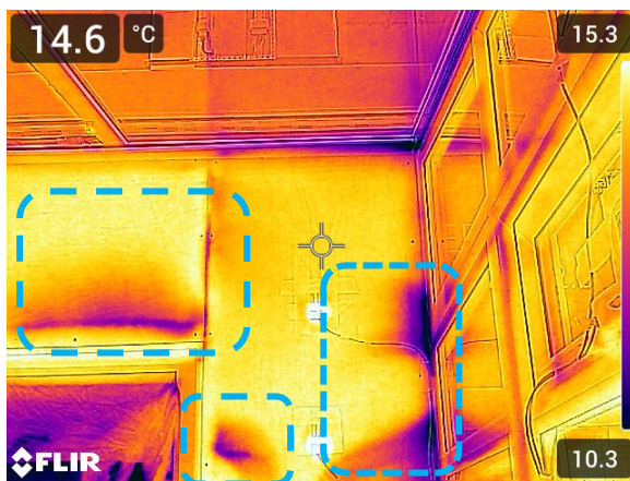
Figure 11 Insulation Under Depressurisation Test-Interior View
