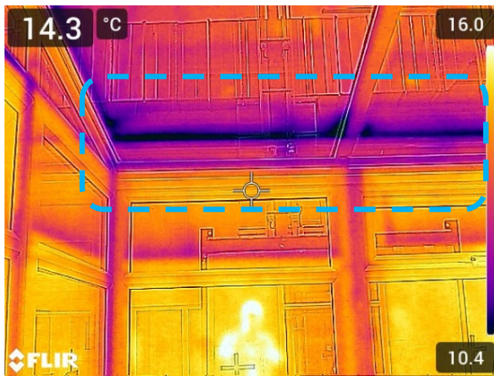
Figure 15 Ceiling Under Depressurisation Test
