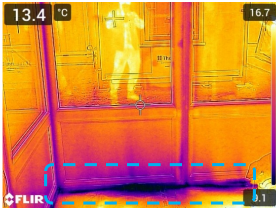
Figure 13 Floor Under Depressurisation Test
