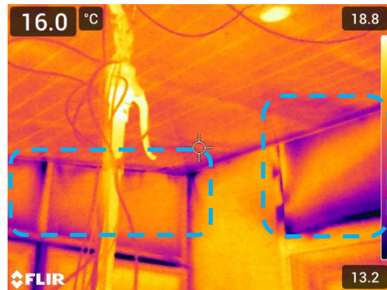
Figure 24 Interior View of the Ceiling (Front)- De-pressure Test
