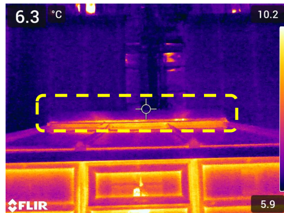
Figure 26 Exterior View of the Ceiling- Pressure Test
