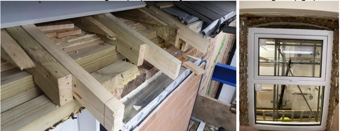
**Figure 4: Whole house approach retrofit works. Eaves being extended over EWI at Stage 6c (left) and window moved in line with EWI at Stage 6d (right)**
