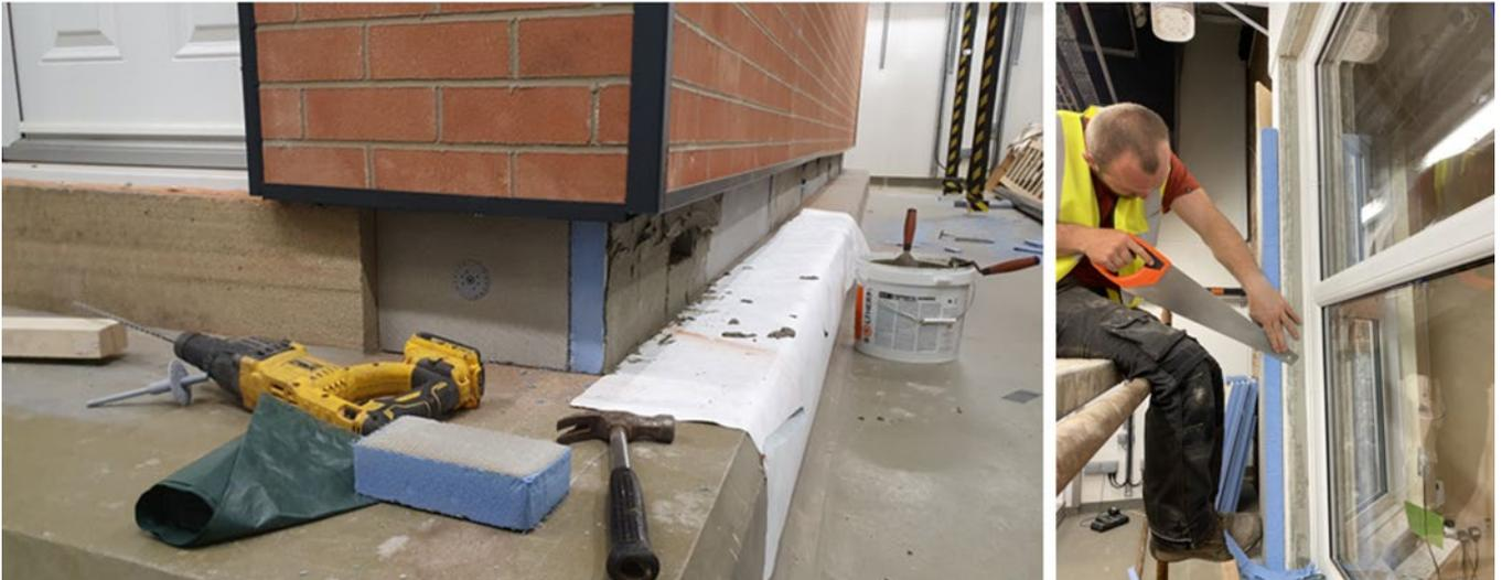
**Figure 3: Whole house approach retrofit works. Extruded polystyrene (XPS) being applied to walls below DPC level at Stage 6a (left) and to bay window mullions at Stage 6b (right)**
