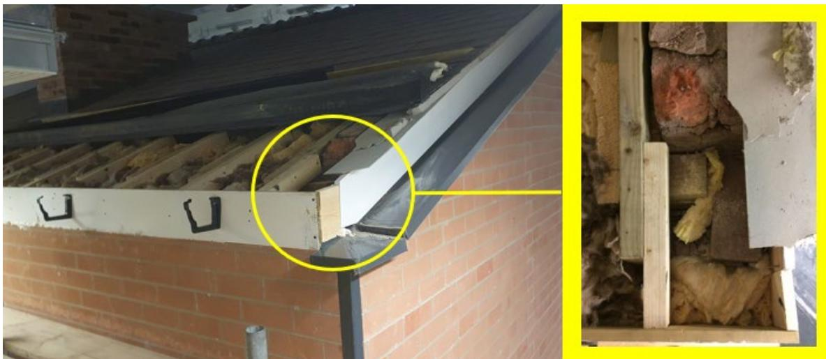
**Figure 32: Hard-to-treat detail at eaves/gable interface at verge resulting in residual risk of surface condensation and mould growth following the whole house approach retrofit**
