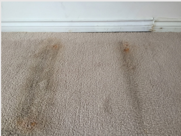
E Stain, rot or mould on floors, carpets or furniture
