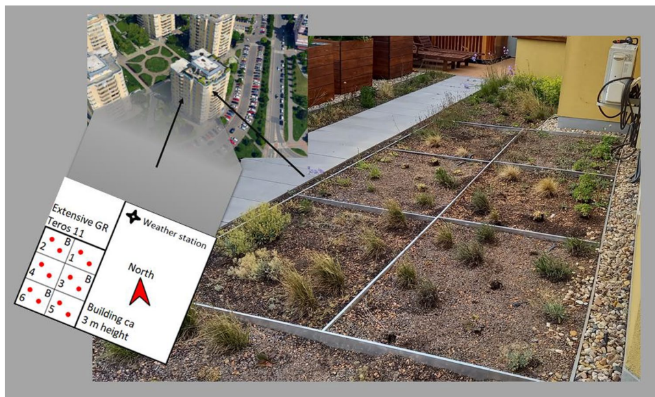
Fig. 1 The layout of experimental green roof plots on the roof of the building (foto June 2022). B = plot with substrate amended with biochar (ROOFChar ® ), other plots with SSE substrate. Red dot = TEROS sensors position in experiental plots
