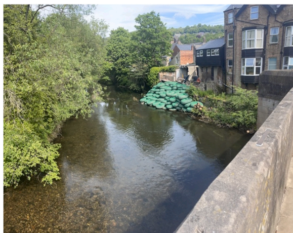
Fig. 1. This image is taken from 2021 showing the main bridge connecting the two parts of Matlock with businesses located to the right-hand side. Sandbags are acting as provisional flood prevention measures, before reconstruction took place in 2022/2023. This area is prone to significant flooding and is at the highest risk level.
