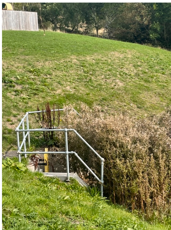
Fig. 4. Attenuation pond around a housing development in Matlock.
