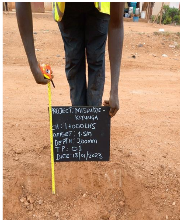
Figure 7.3: Excavated Trial Pit (TP01) at Km 1+000
