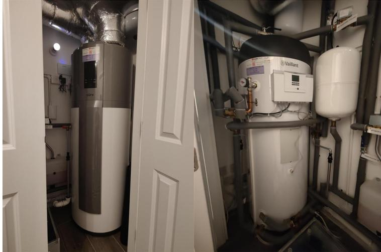
Figure 3. Curv hot water cylinder (left) and Vaillant ASHP cylinder (right)
