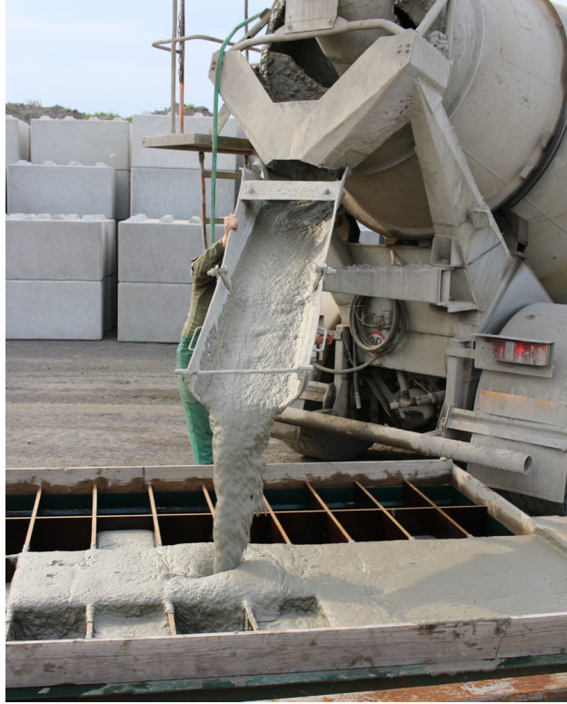
Figure 7: Pouring of the industrially produced mixture (4/6 SP4 B) into large-scale molds.
