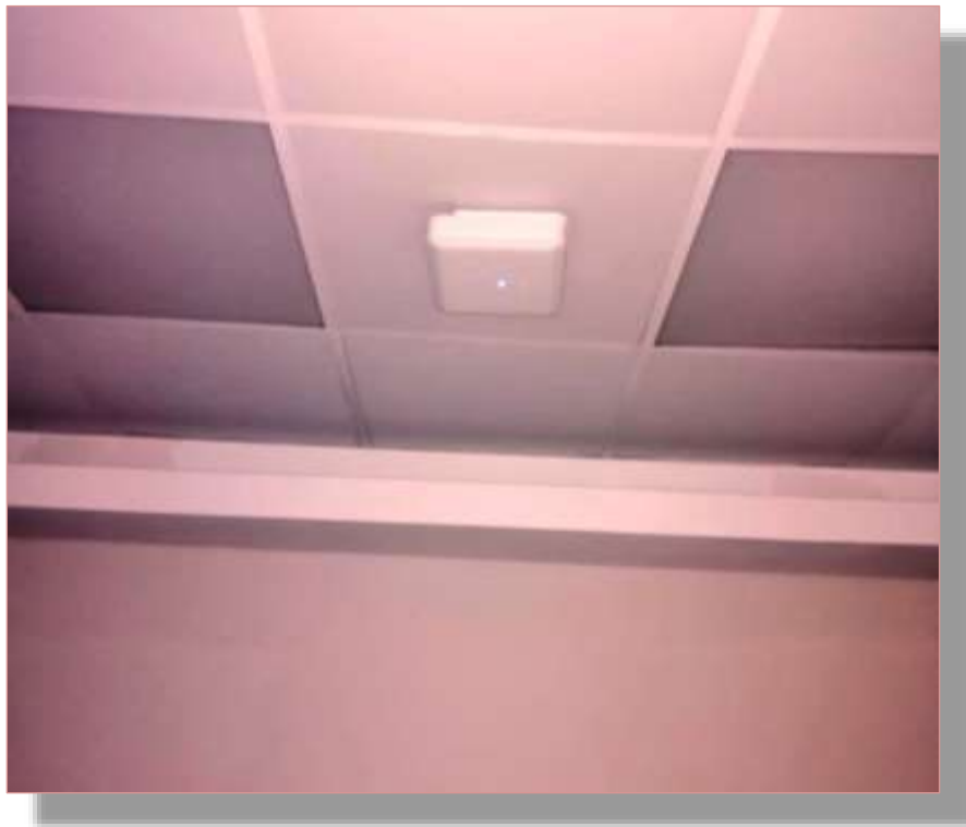
Figure 5.2: Wi-Fi Antenna operating at 5.8 GHz is mounted on the ceil of the room and directed downwards.
