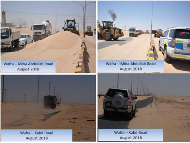
Figure 3.3: Severe sand encroachment along Wafra Roads (August 2018) Source: Misak et al. (2019).
