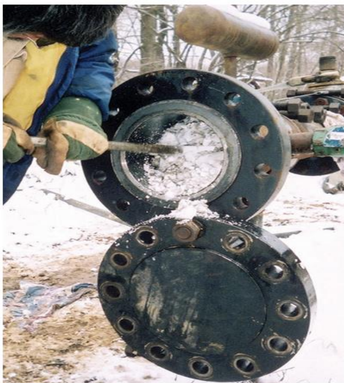
Figure 2.13 Gas hydrate plug in a pipeline (Boschee, 2012)
