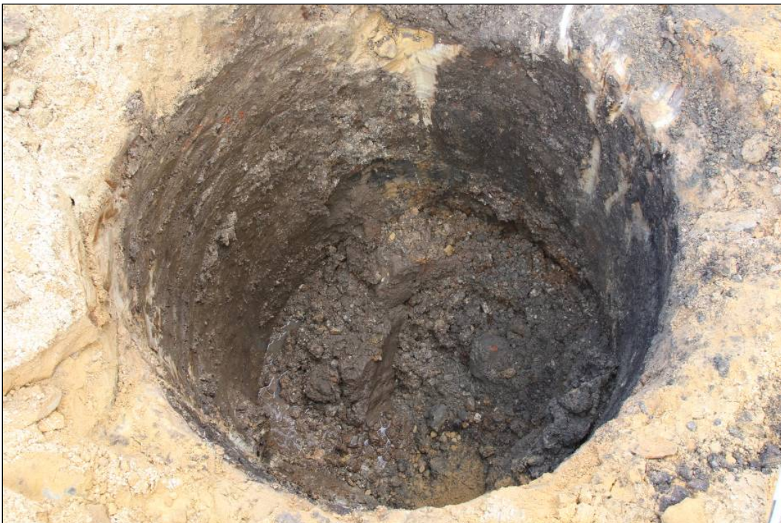
Plate 2: Lower excavated 1.5m depth (to 3m) of the well looking north-west
