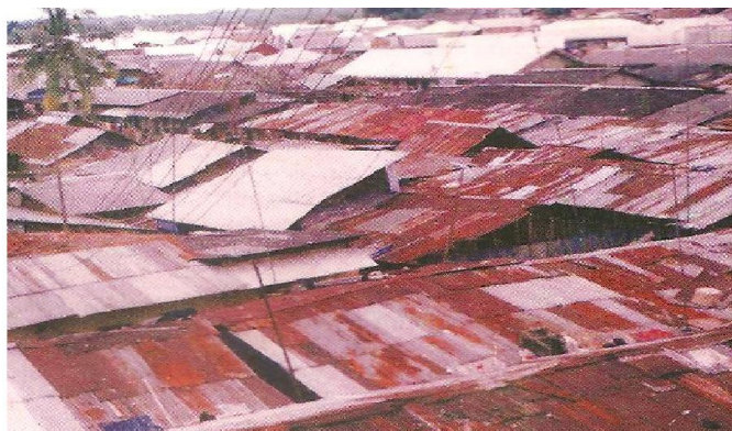
Figure 2. Corroded Roof in the Niger Delta Area of Nigeria
