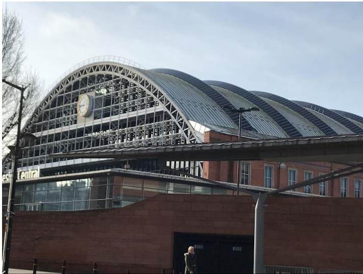
Figure 6.1.15 Manchester Central view from side illustrating a series of trussed arches.
