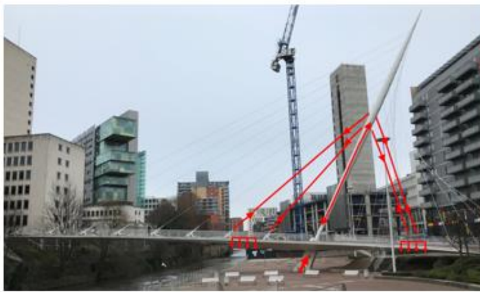
Figure 6.1.11 Screenshots of A.R. video before and after animations describing structural load paths.
