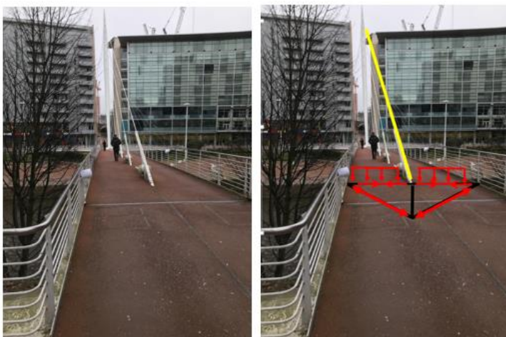
Figure 6.1.12 shows how the triangular box girder supports the weight of the footpath is discussed with tension and compression arrows and the significance of the box girder being a closed (rather than open) section shape.
