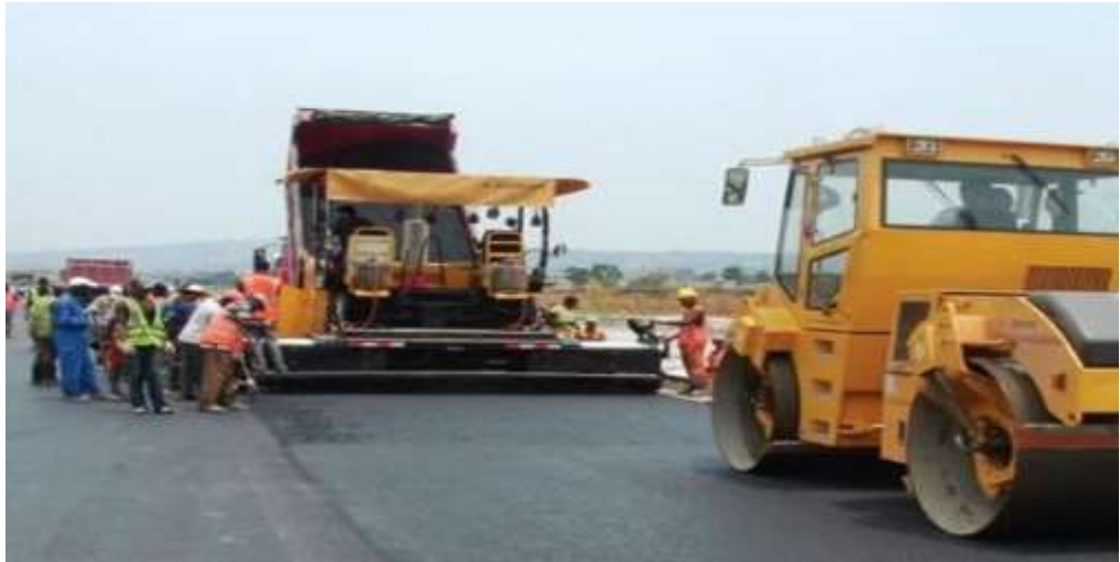
Figure 2.8: Muritala Muhammed airport Road's Reconstruction
