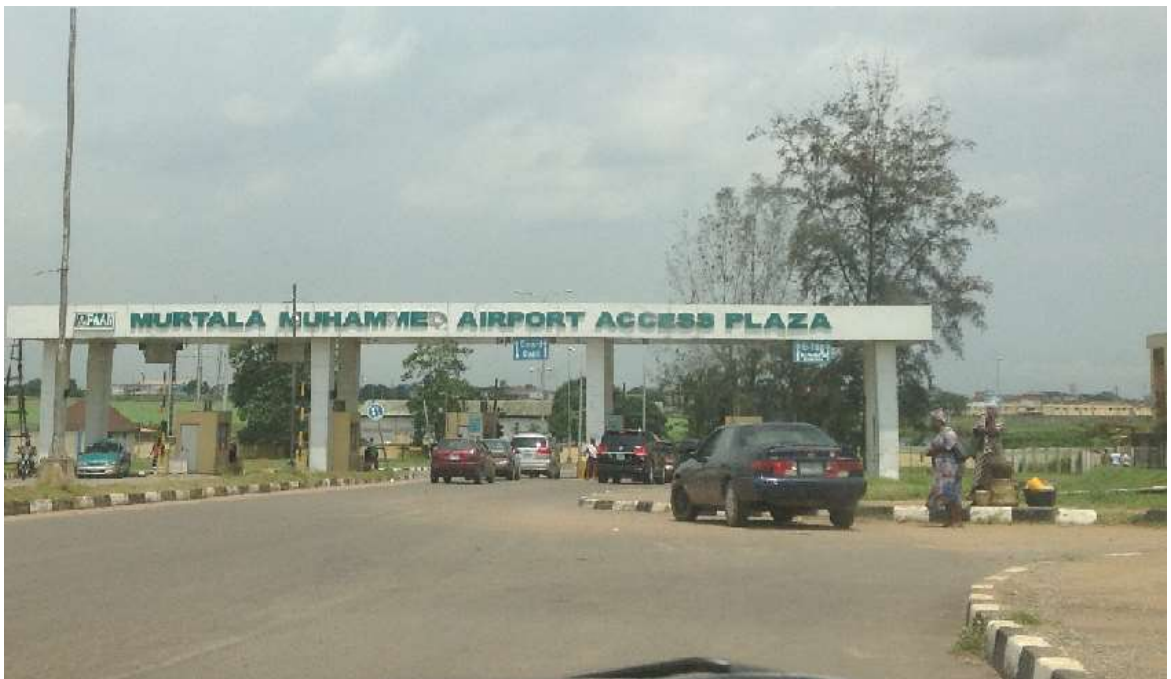
Figure 2.7: Muritala Muhammed Toll road
