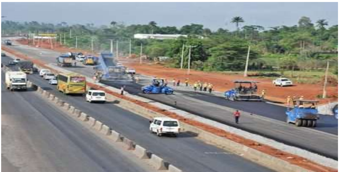
Figure 2.9: Reconstruction of Lagos-Ibadan expressway
