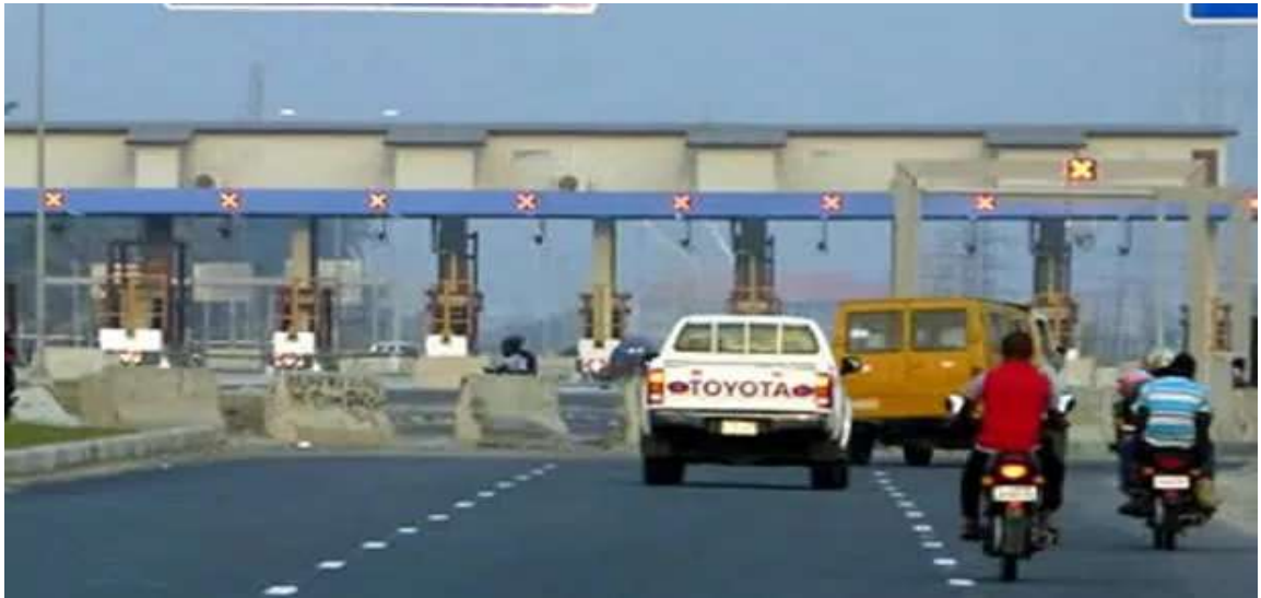
Figure 2.5: Lekki-Epe Toll Road
