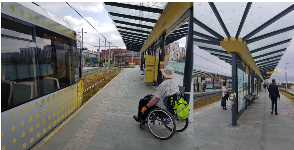
Figure 28: Metrolink station showing sheltered tram stops and tactile paving
