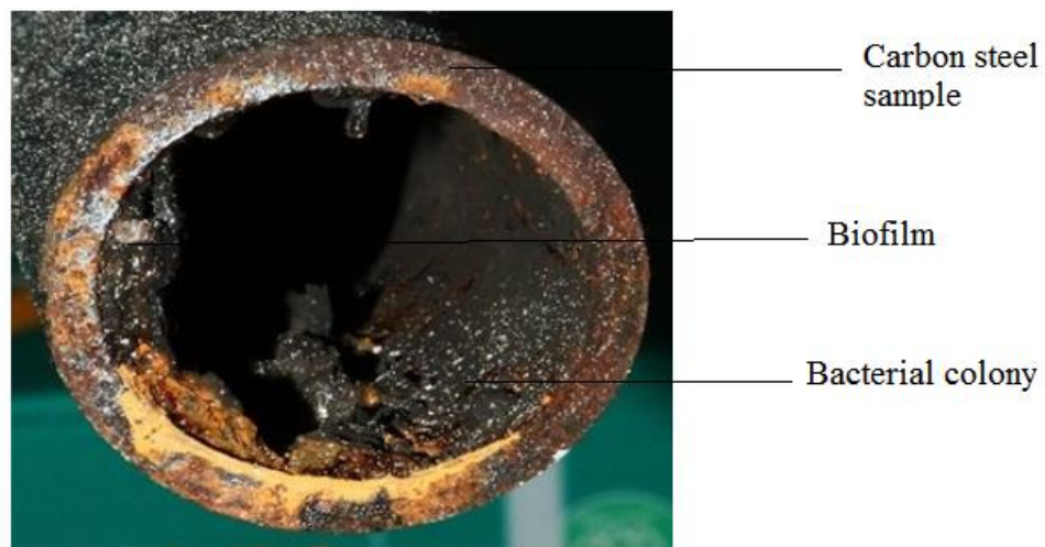
Figure 2-12: Microbiologically induced corrosion in a carbon steel weld
