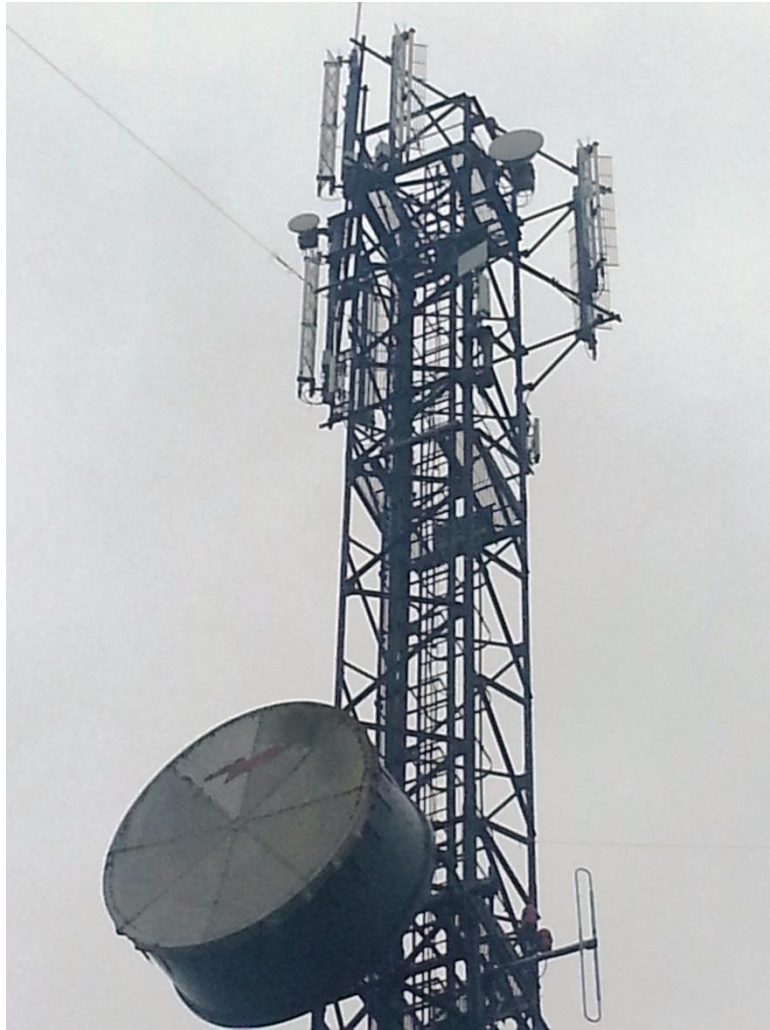
Figure 5: Early cellular antennas, as deployed for the analogue network, being reused to support GSM signals (2014).
