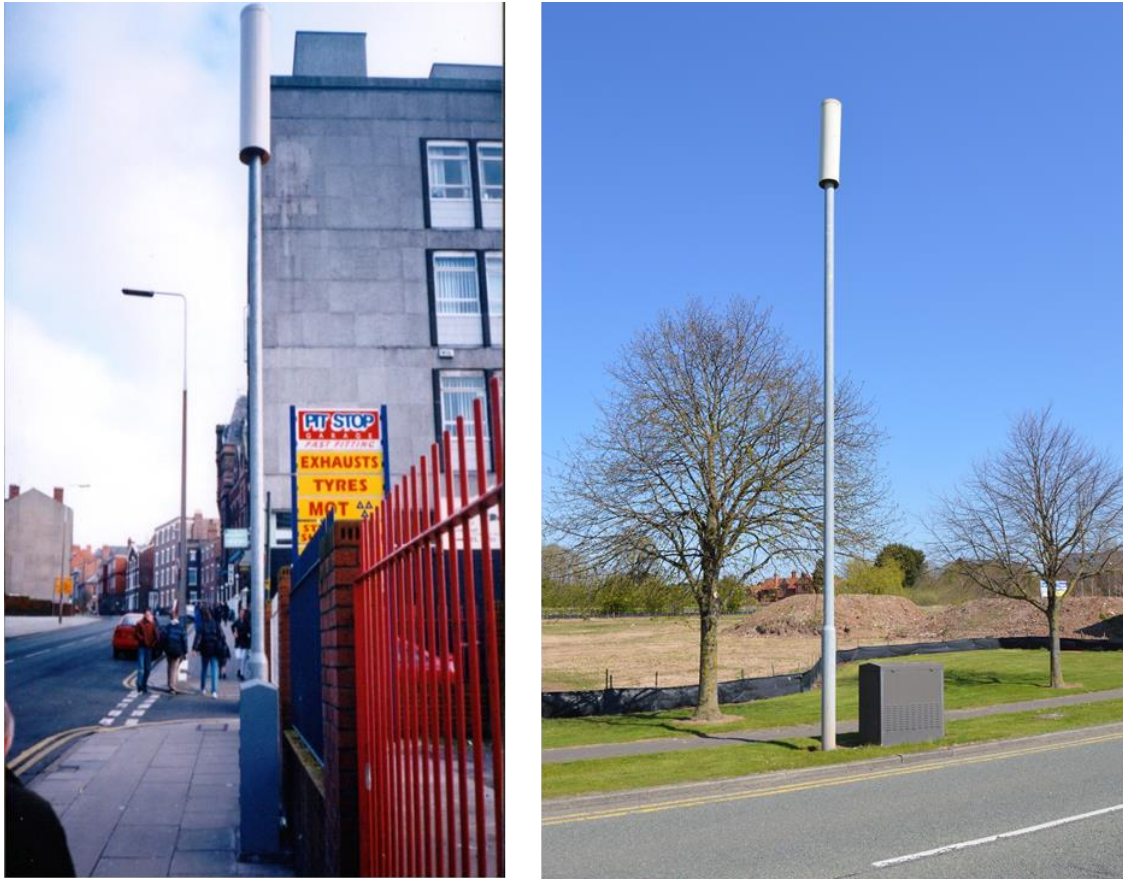
Figure 22: Micro-cell installations with lamppost like columns (left image 1999, right 2015)
