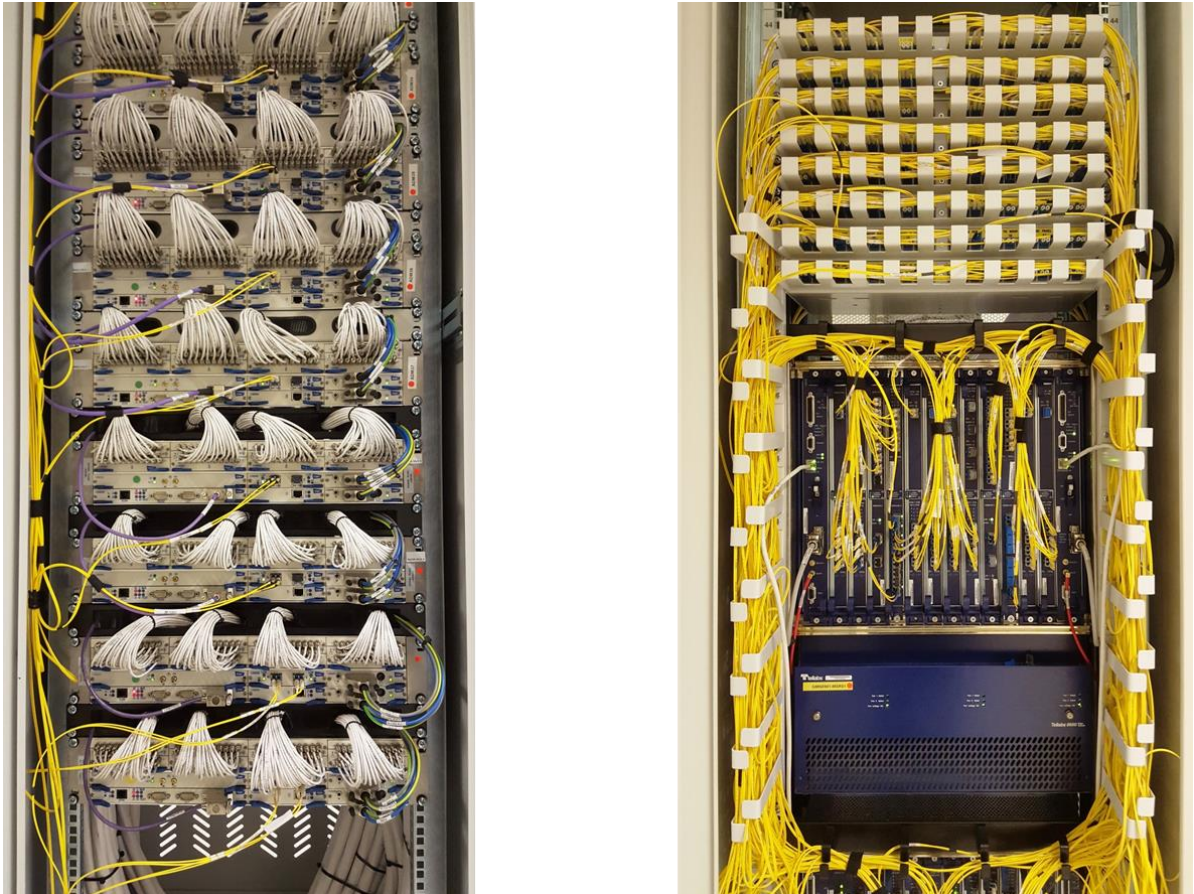
Figure 78: Siae STM-1 ADMs (left) and core site Tellabs MSSR (right) (2016)
