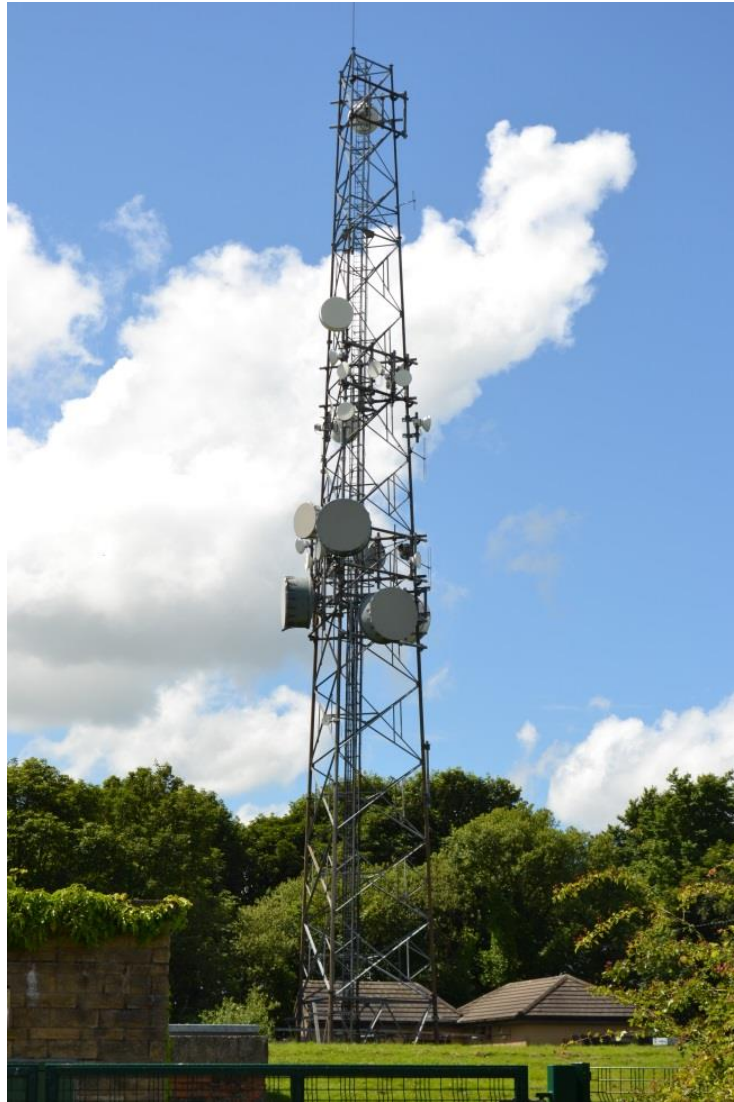
Figure 21: BSC site with point to point microwave connectivity for Abis and Ater interface circuits (2014)
