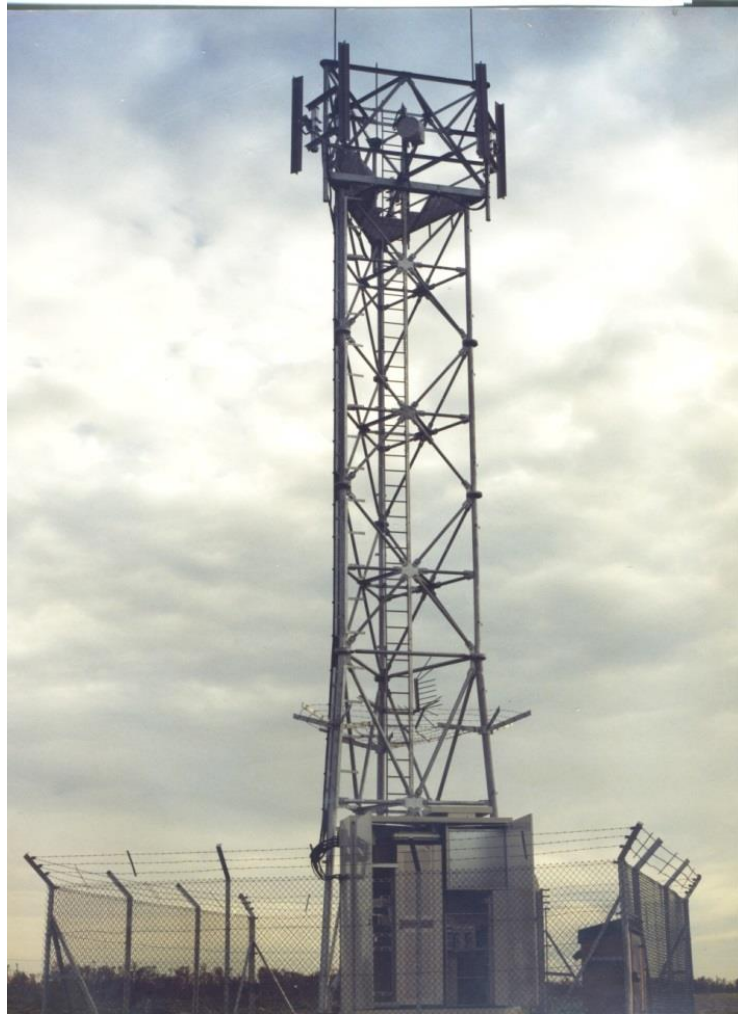
Figure 14: Early Orange cell site with Marconi antennas but no LNAs (1993) Source: Orange UK
