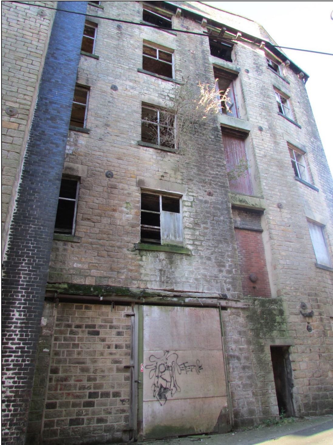
Plate 5 Eastern elevation with taking-in doors and modified ground-floor entrance
