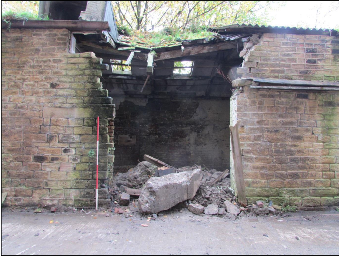
Plate 78 There appears to have been an entrance located here into the east shed, however roof collapse has damaged this area
