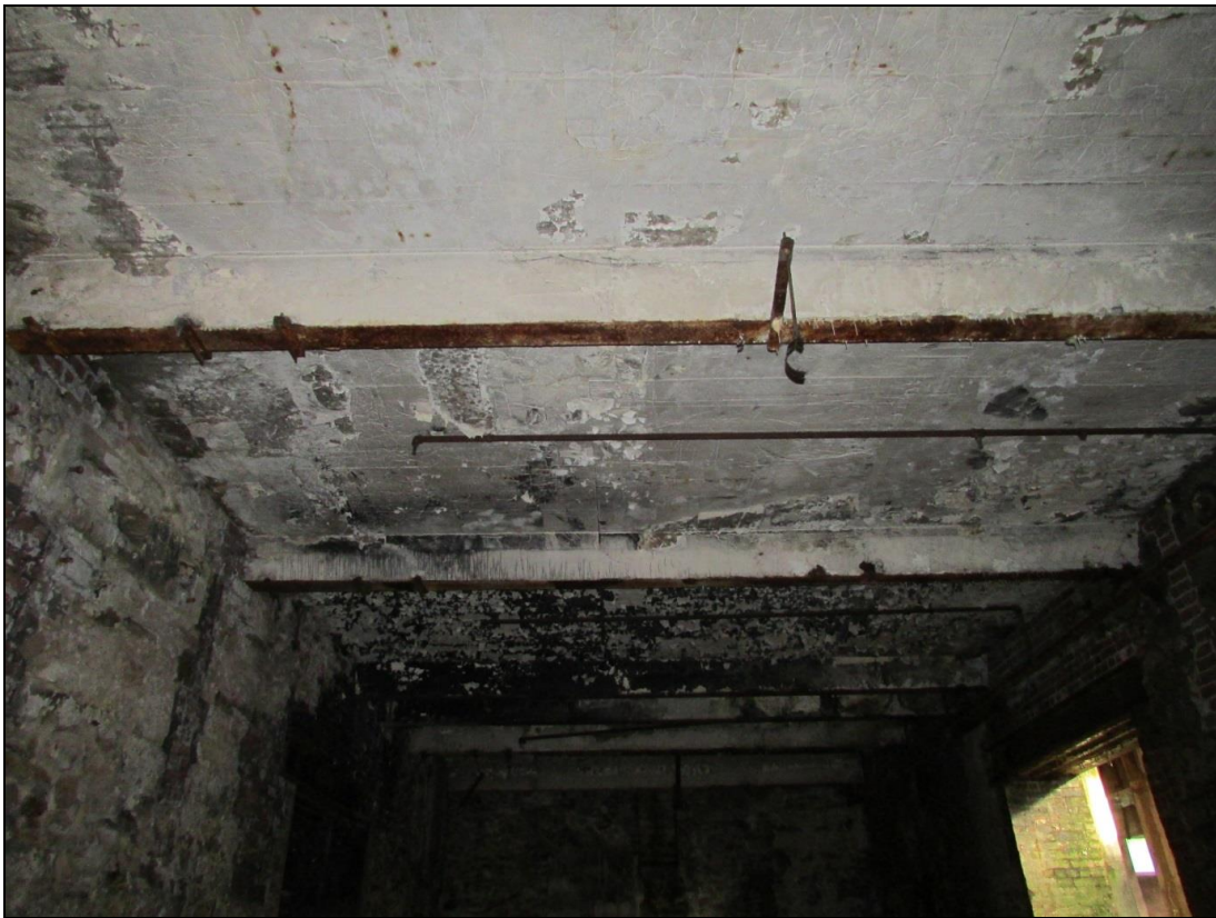
Plate 41 The flat ceiling of the engine house ground-floor, which is probably later in date
