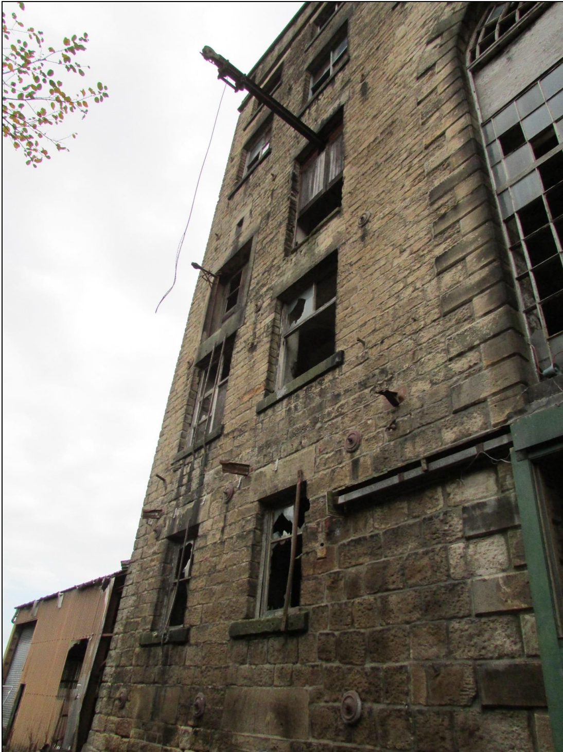
Plate 37 The western part of the engine house has taking- indoors on the third-floor including in situ cat head and swivelling crane jib
