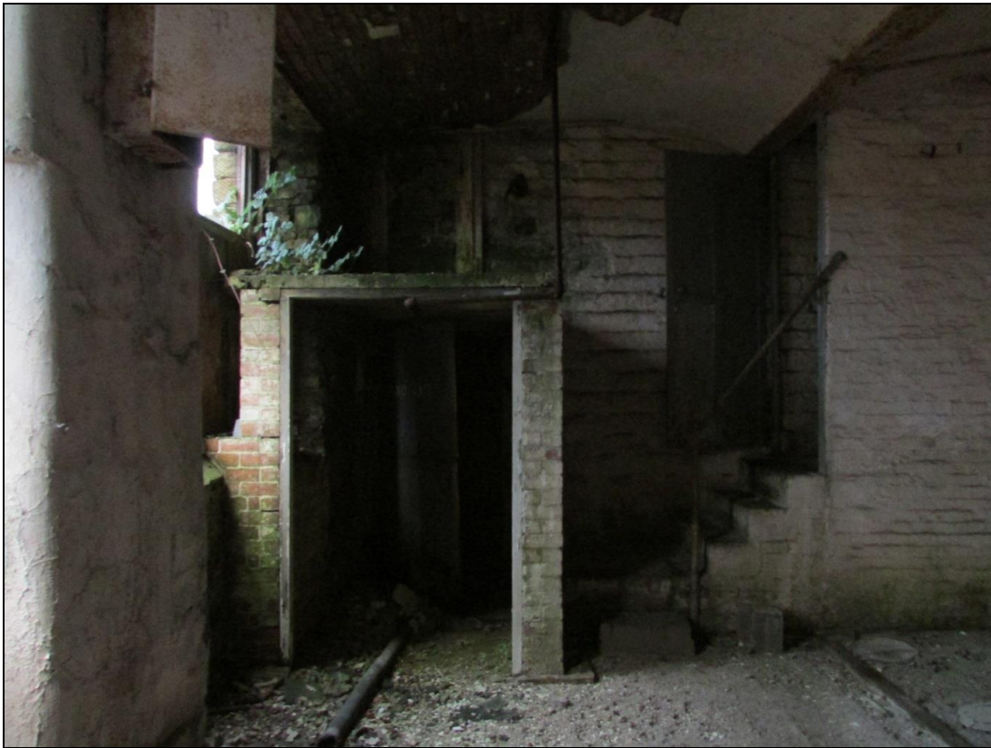
Plate 47 Later machine made brick divisions (including the stairs to the right) within the first-floor of the engine house
