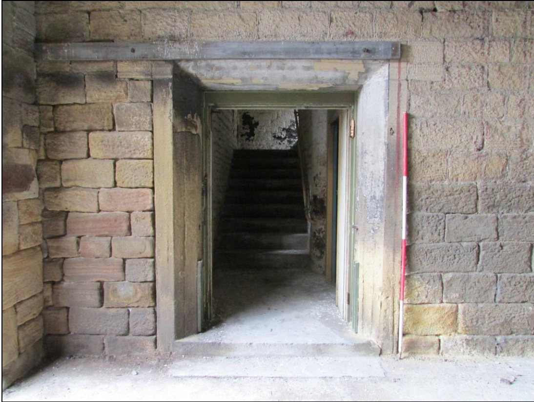
Plate 4 Original entrance into the mill, via the stair tower
