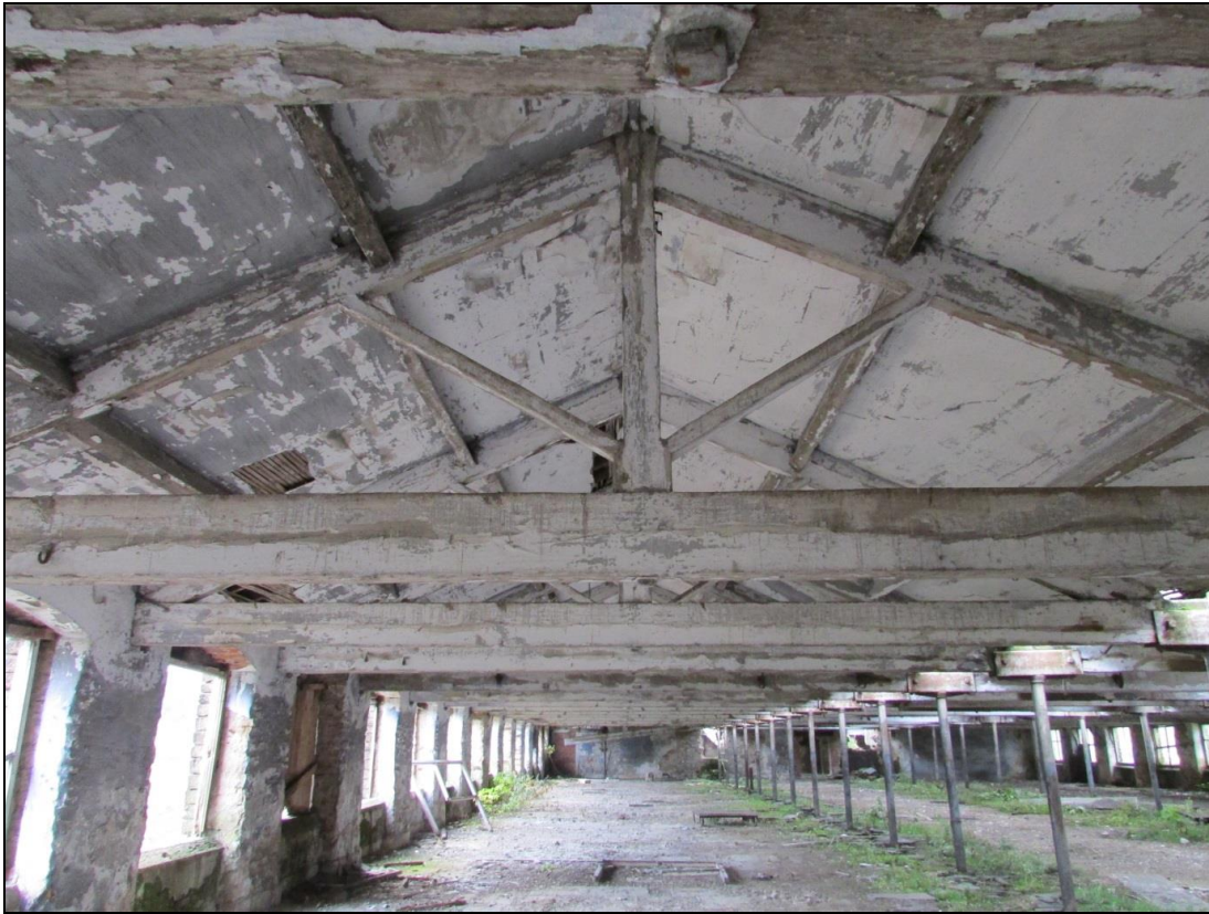
Plate 29 One of the three pitches spanning the roof showing the king post style structure
