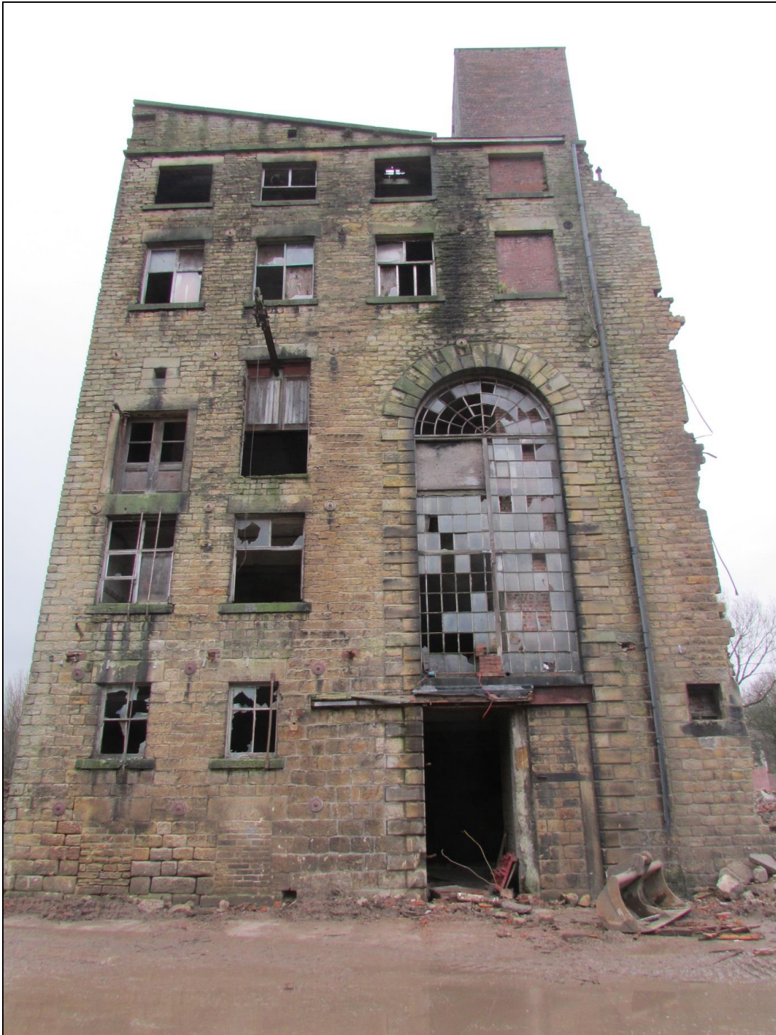
Plate 35 Southern elevation of the engine house
