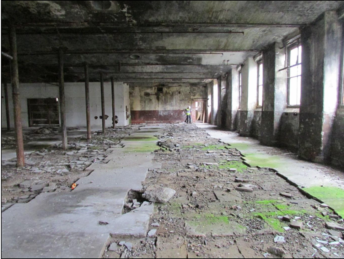
Plate 13 Robbed out flagged flooring on the first-floor
