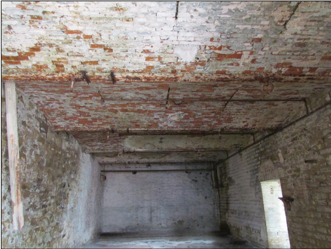
Plate 58 Metal fixtures, including hoist rings, would have been used to lift components vital to maintaining the engine
