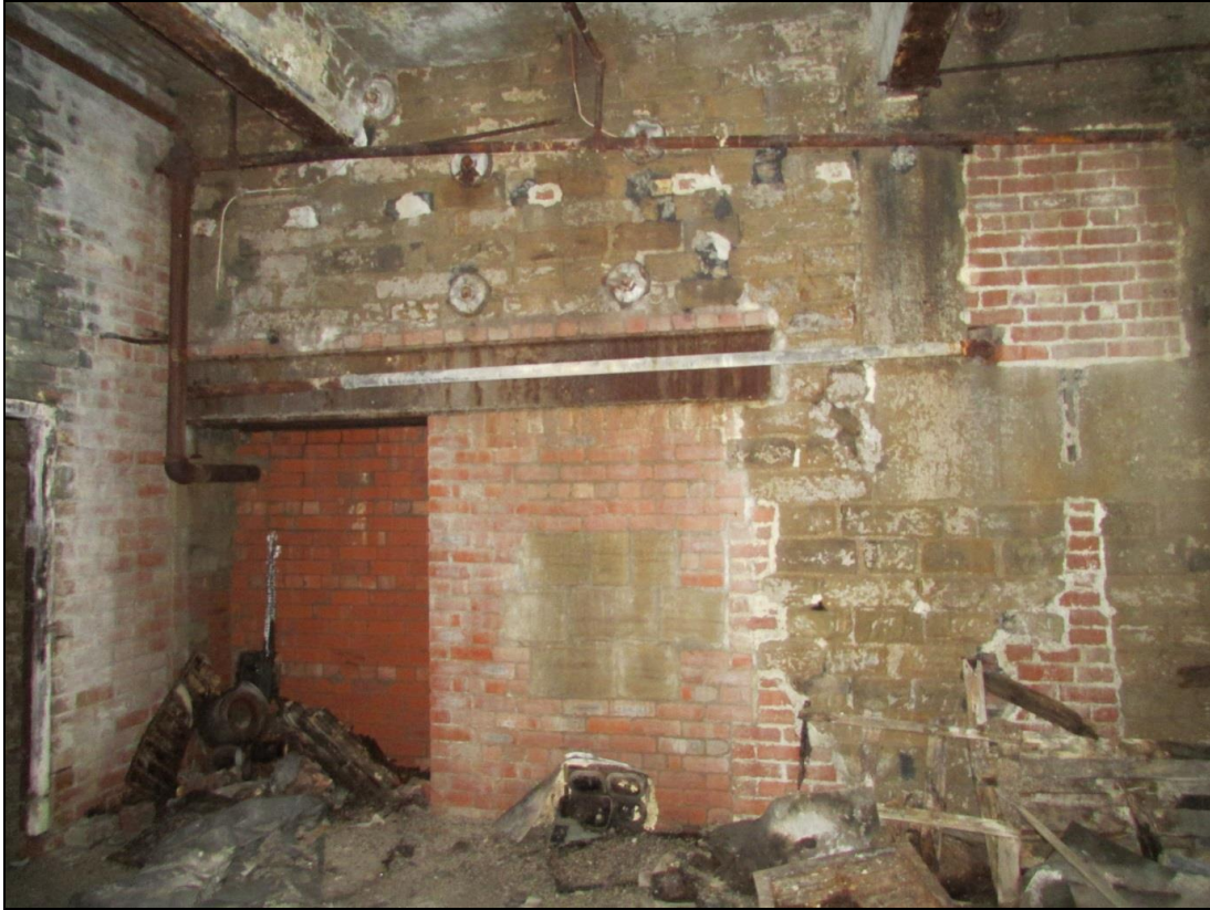
Plate 48 Later inserted doorway, which was then blocked and a blocked footstep bearing for another upright shaft (see also Plate 16 for the bracket on the other side of the gearing wall)
