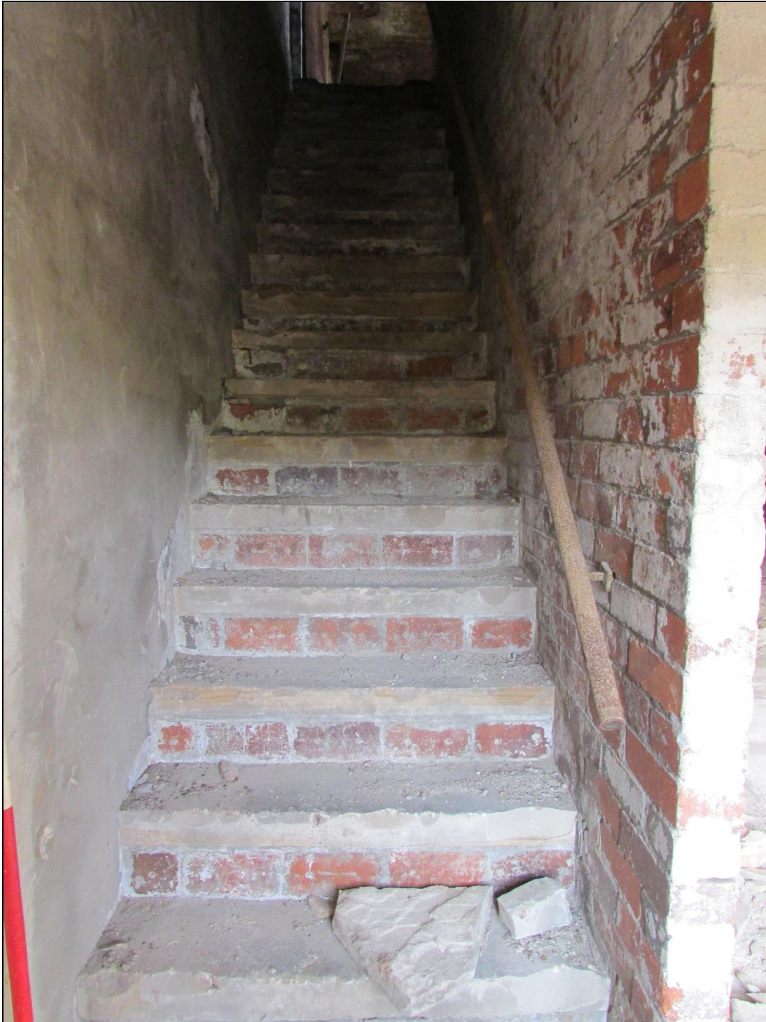
Plate 53 Later steps leading from the second to the third-floor of the engine house
