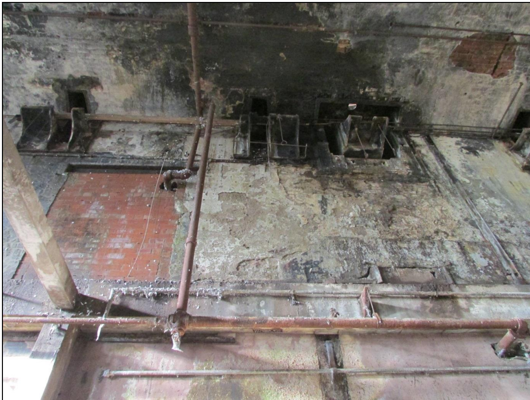
Plate 16 The bracket and aperture for the driveshaft is located to the right; a blocked entrance and two more brackets are shown to the left
