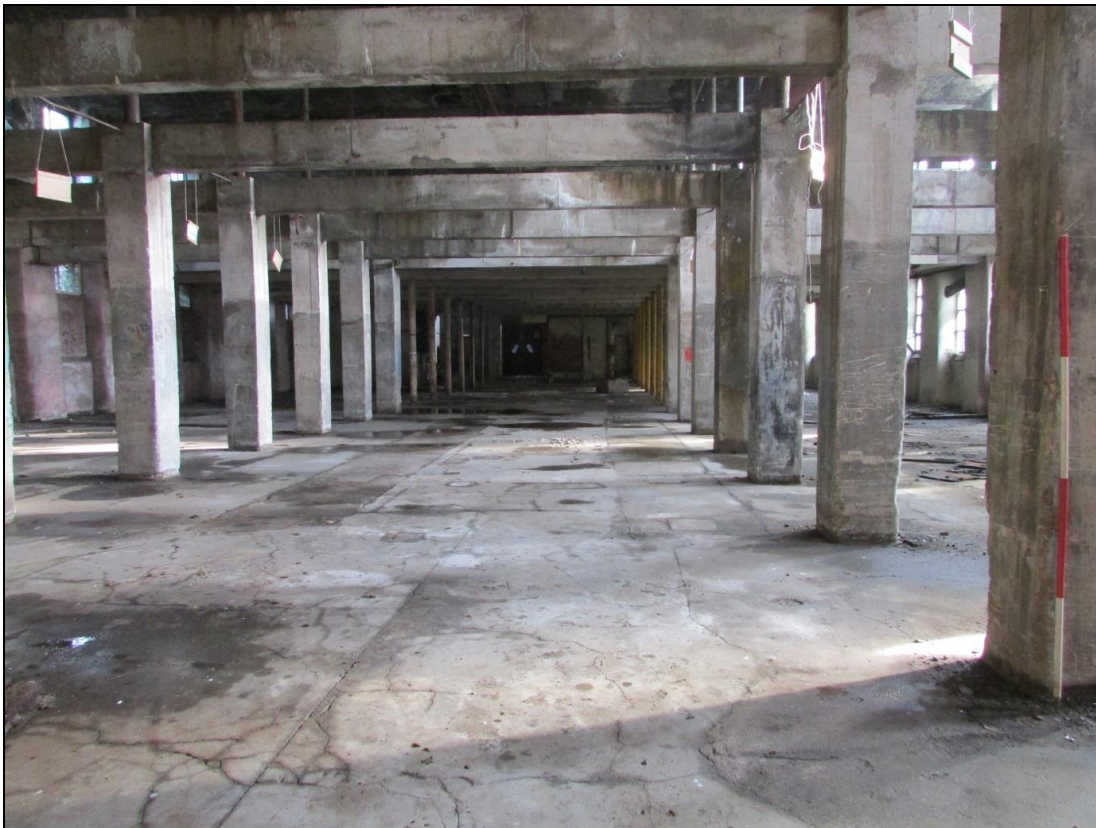
Plate 7 The iron columns at the western end of the mill were encased in concrete
