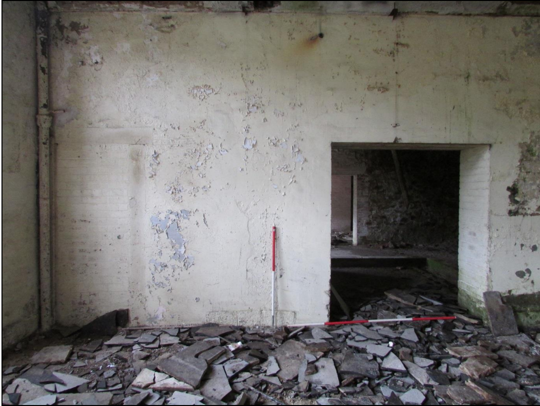
Plate 23 On the second-floor, the entrance on the right has been inserted at a later date, whilst the entrance to the left has been blocked
