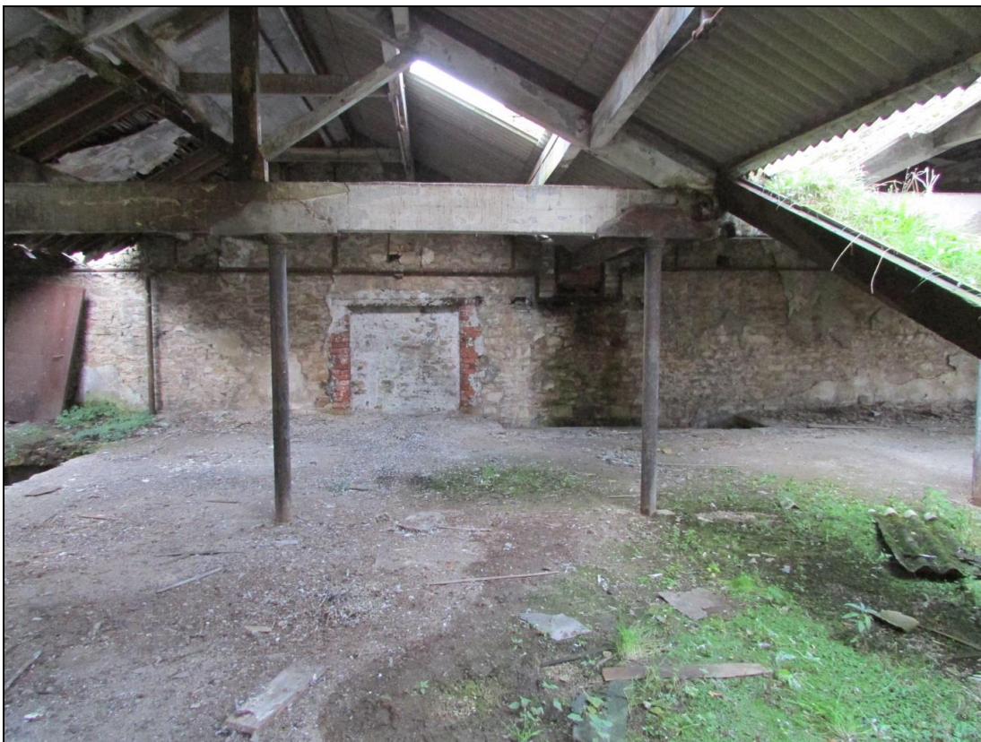
Plate 63 General view of the fourth-floor of the engine house
