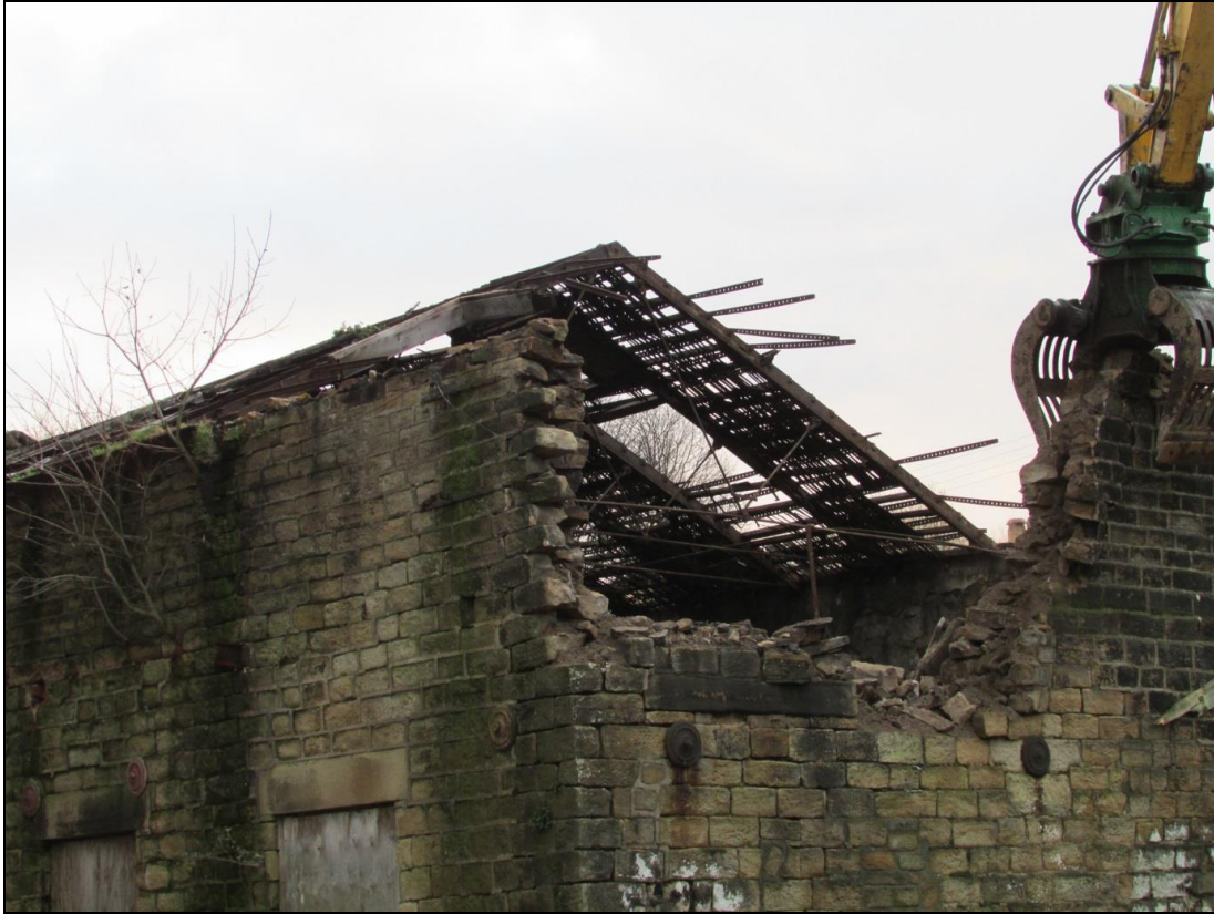
Plate 89 The west shed during demolition. The roof was constructed entirely from iron
