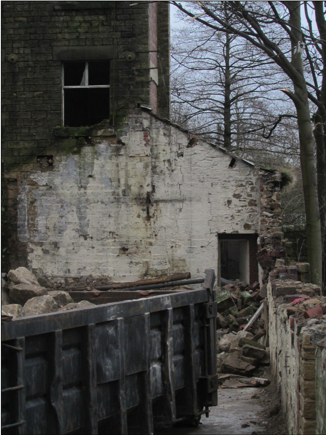
Plate 68 Close up of the western elevation of the office block
