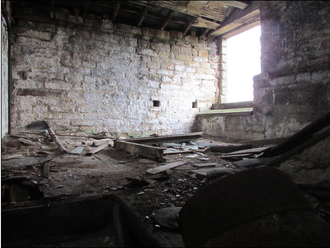
Plate 31 A small attic space located in the stair tower and accessed from the fourth-floor
