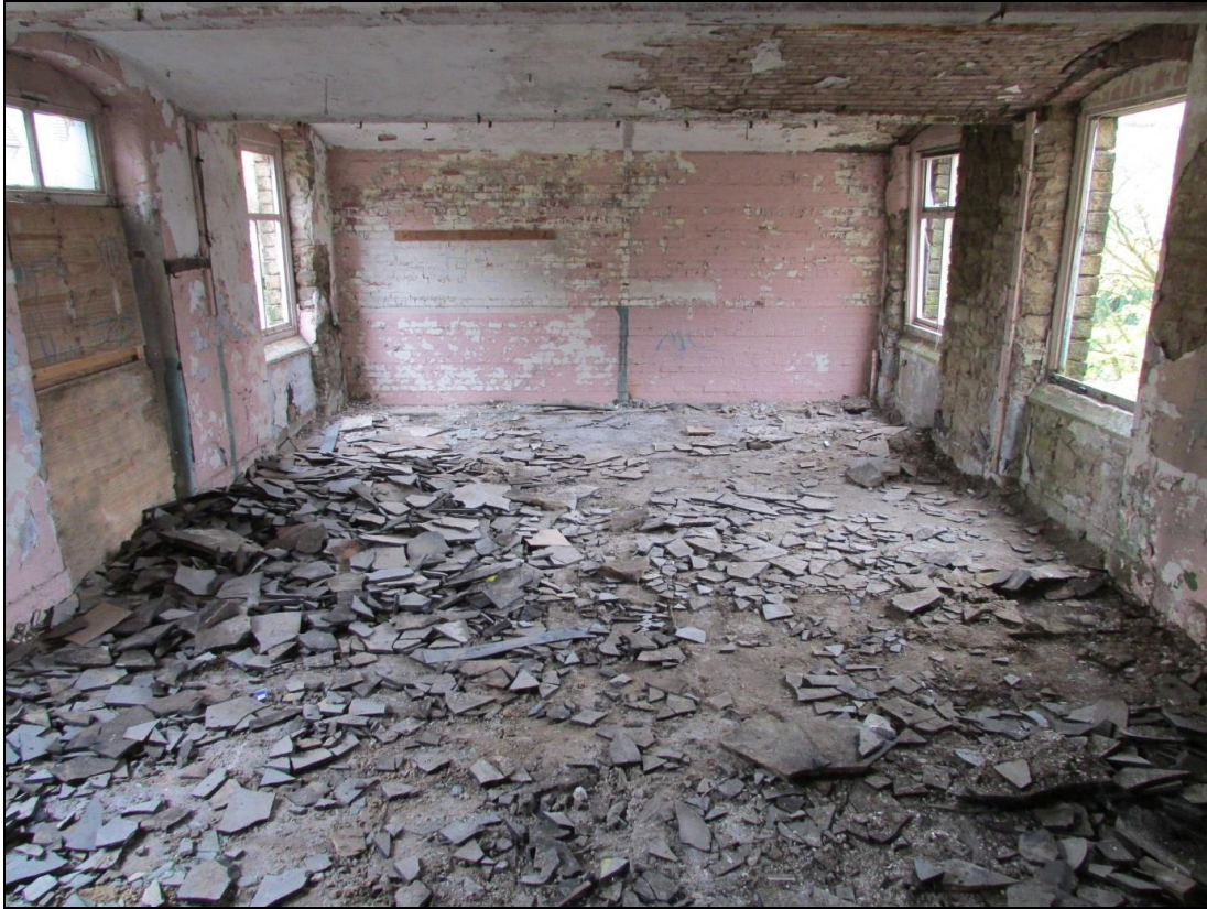
Plate 72 General shot of the Office Block-second floor
