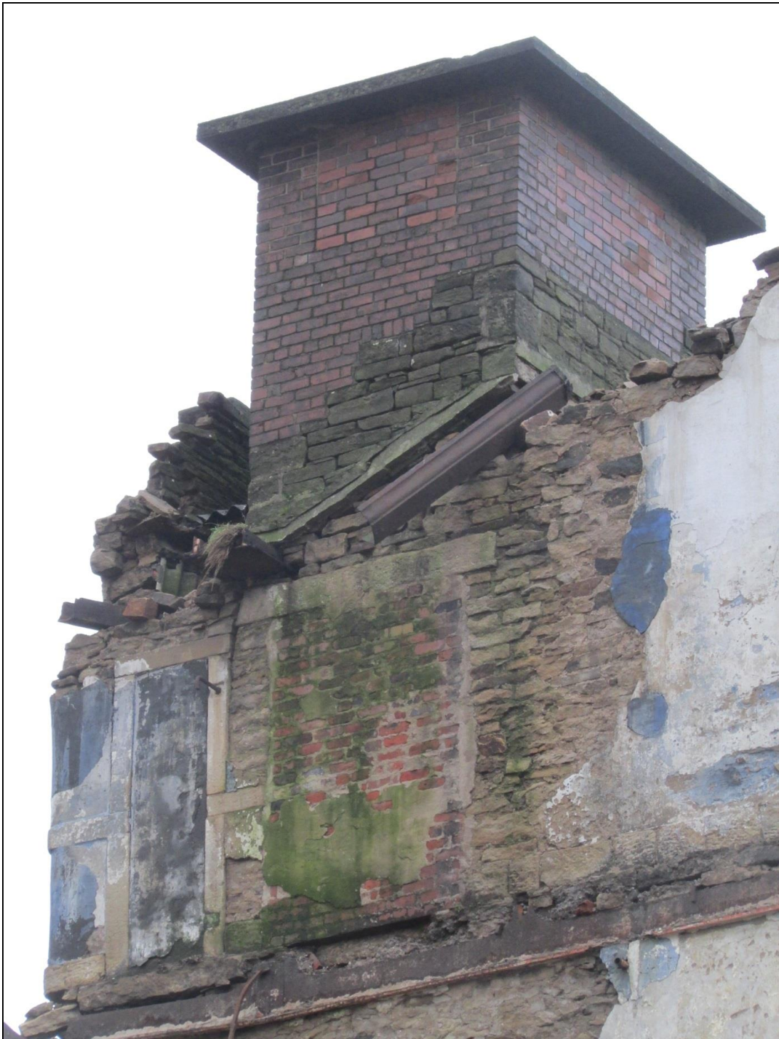
Plate 6 Close-up of the eastern lift shaft headgear shows the partial reconstruction in brick, as well as subsequent blocking of apertures
