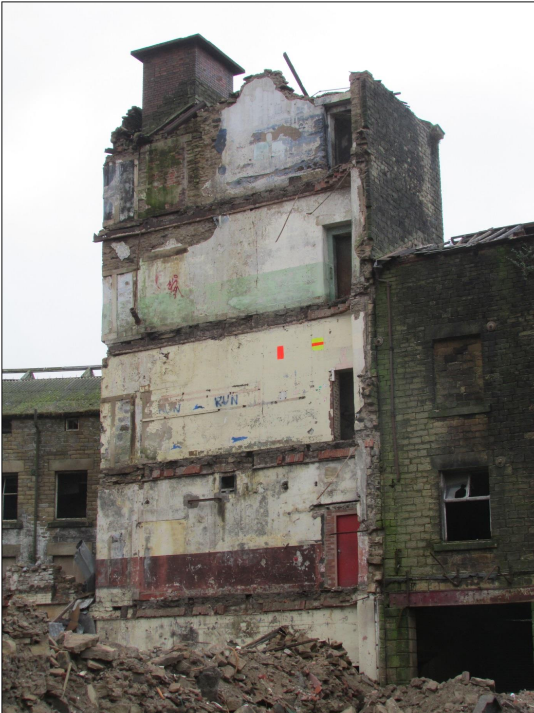
Plate 91 The demolition of the central part of the mill revealed the phasing of the lift shaft
