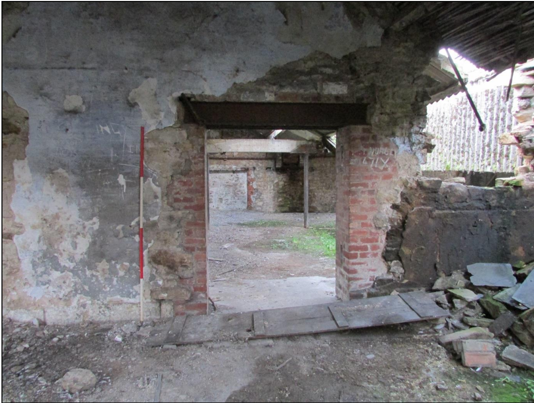
Plate 30 An inserted entrance into the engine house and position of robbed out top steady bracket (to the right)
