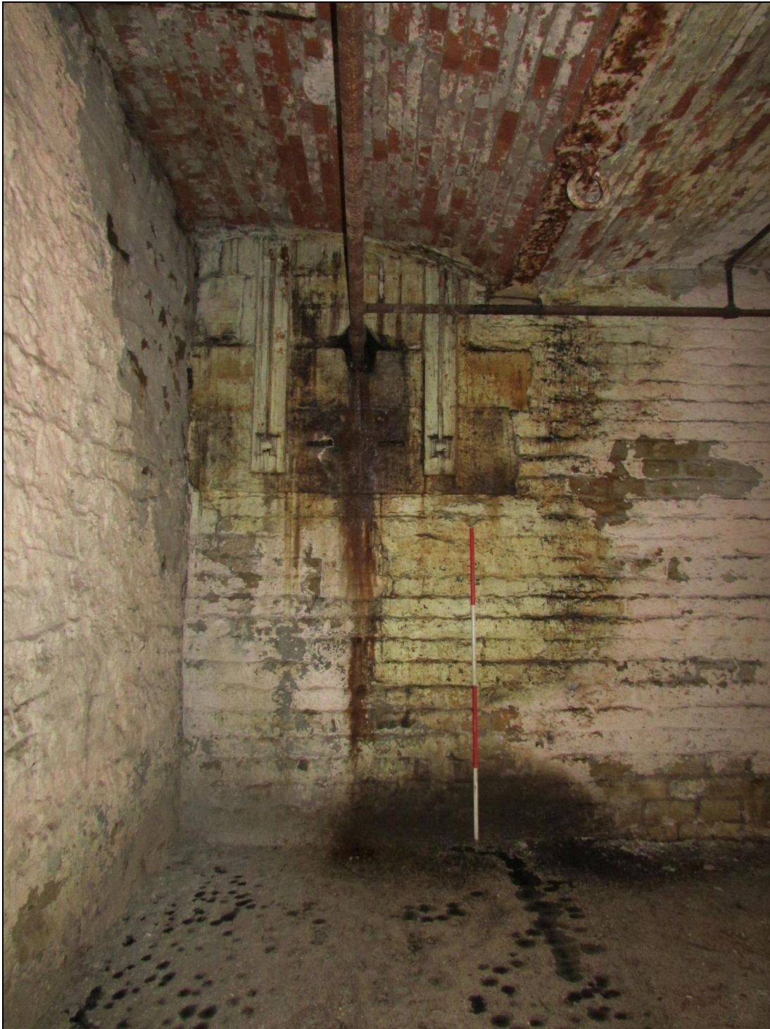
Plate 57 Original metal brackets supporting the power transmission system, later adapted for a sprinkler system.
