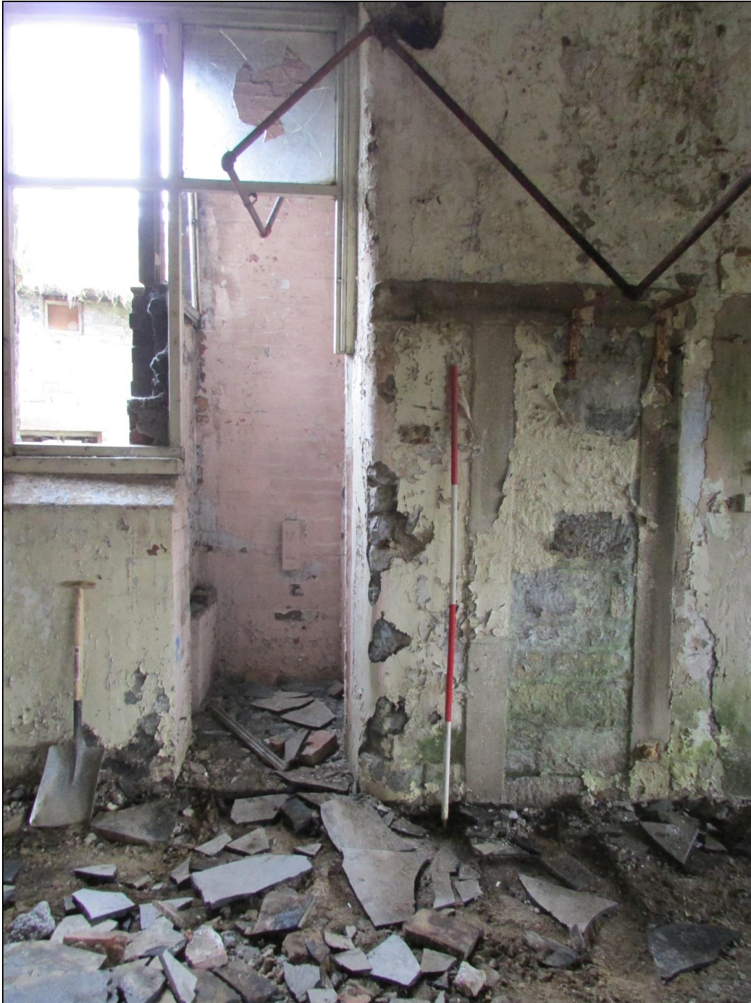
Plate 21 The entrance on the left leads into the privy tower extension and the blocked entrance led originally into the privy tower
