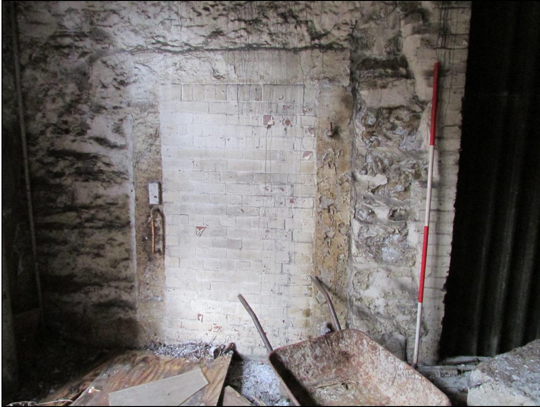
Plate 39 Blocked entrance located within the engine house dividing wall
