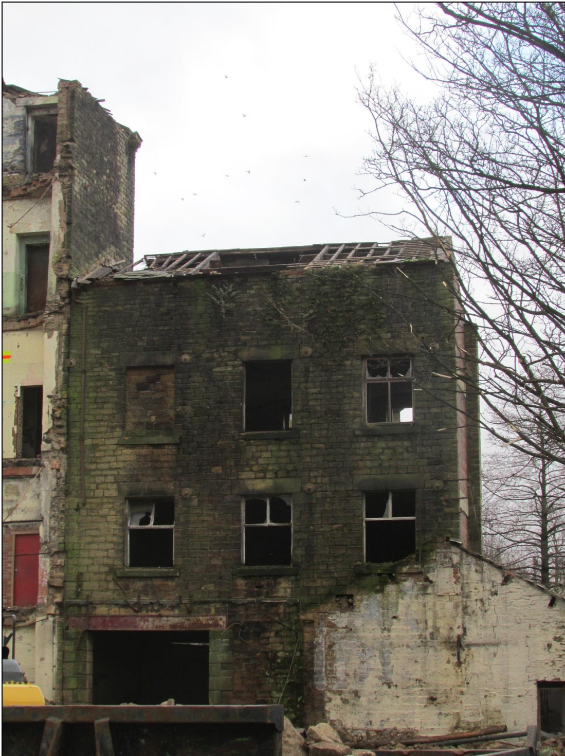
Plate 67 Western elevation of the office block, after the demolition of the sheds
