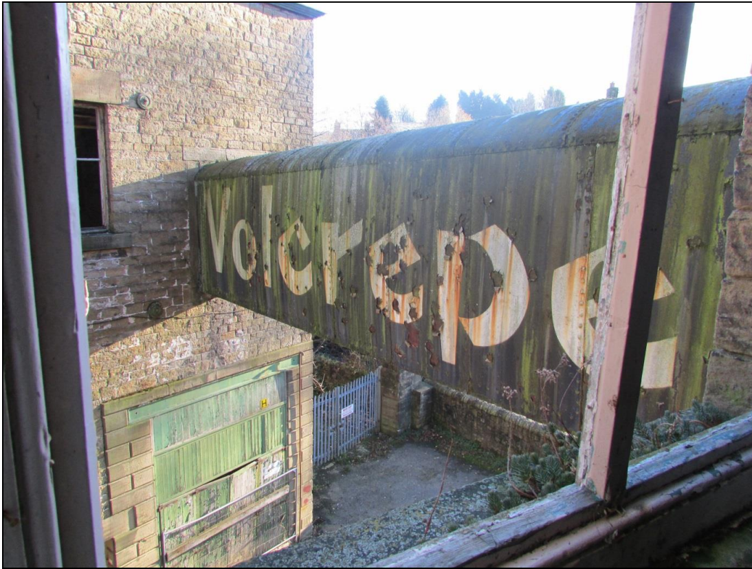
Plate 65 Metal walkway with the Volcrepe logo still in good condition
