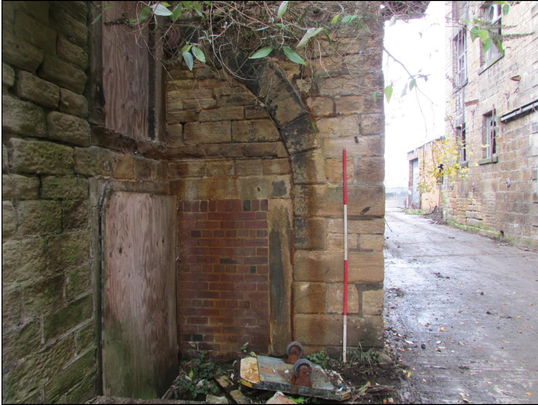
Plate 88 The eastern elevation of the west shed, with a former arched entrance with two phases of blocking evident
