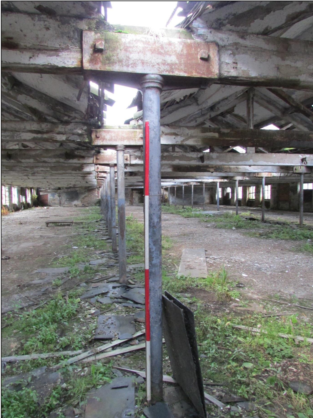
Plate 28 Detailed shot showing how the roof was supported using the cast iron columns
