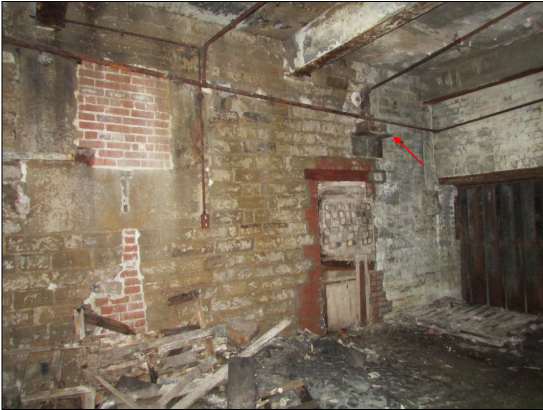
Plate 49 Another inserted doorway had been blocked subsequently with a mixture of unknown materials. An original engine fitting is visible above (arrowed)
