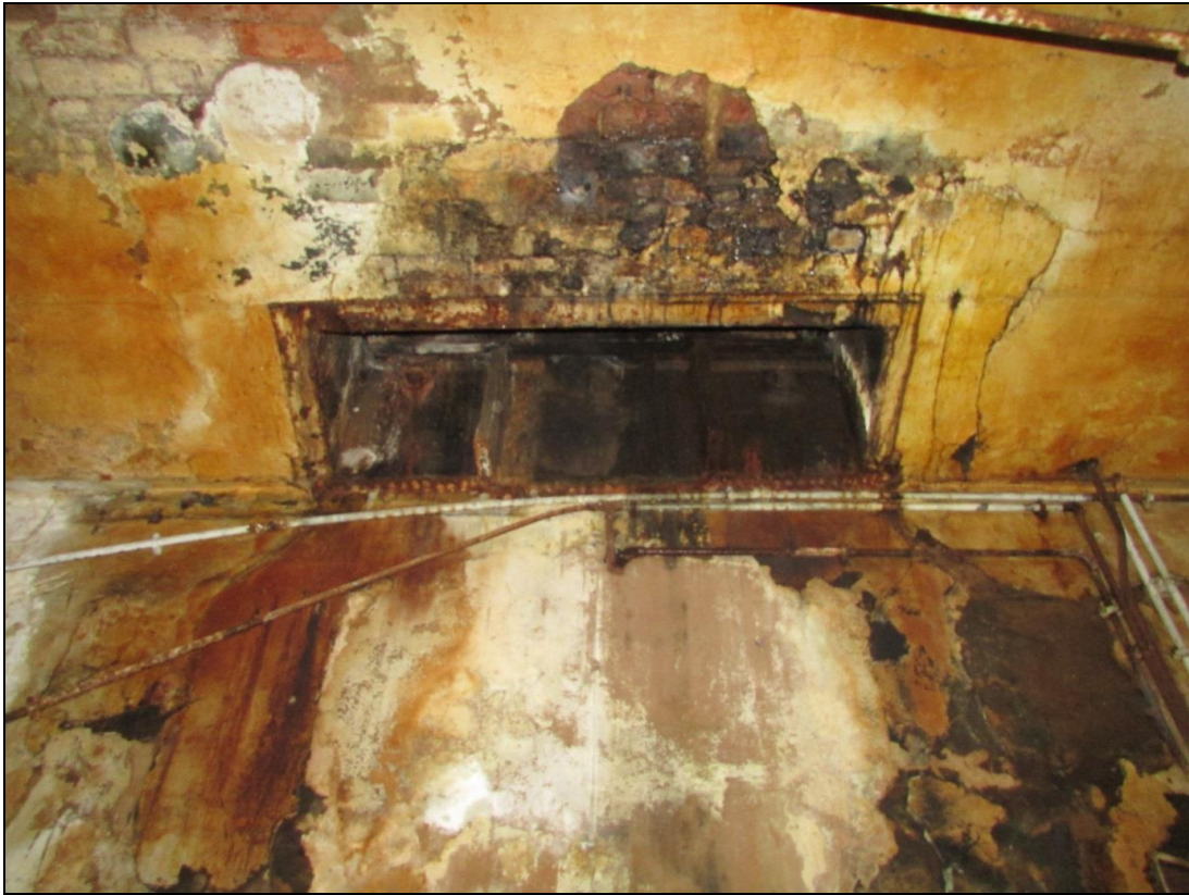
Plate 26 A metal lined aperture inserted into the ceiling on the third-floor
