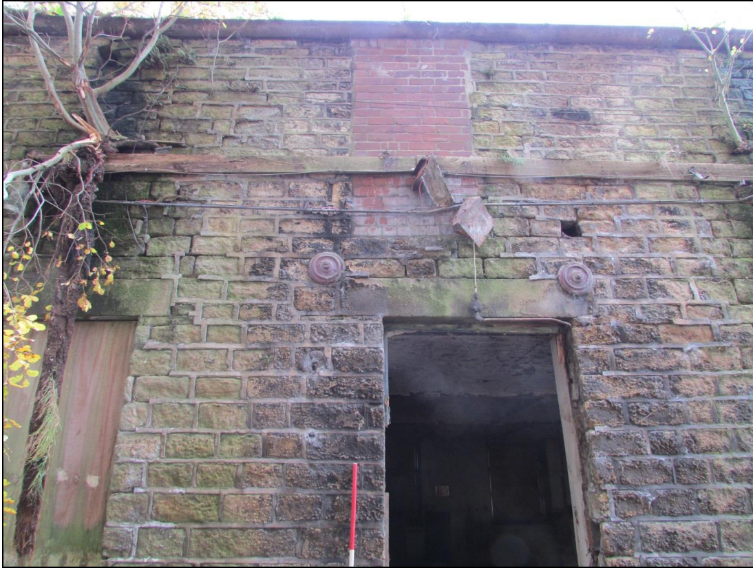
Plate 87 A possible blocked window is visible above the entrance to the west shed
