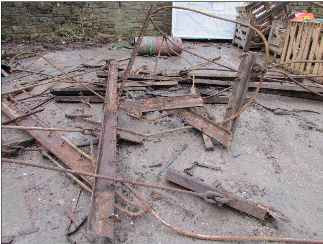
Plate 90 Remnants of the iron roof of the west shed
