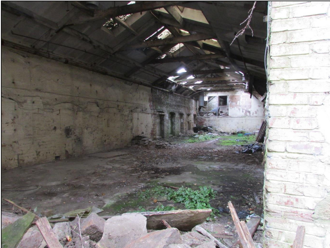
Plate 80 General view of the interior of the eastern and middle sheds. A machine made brick and timber division is visible in the background. Also visible are the former windows which were blocked subsequently
