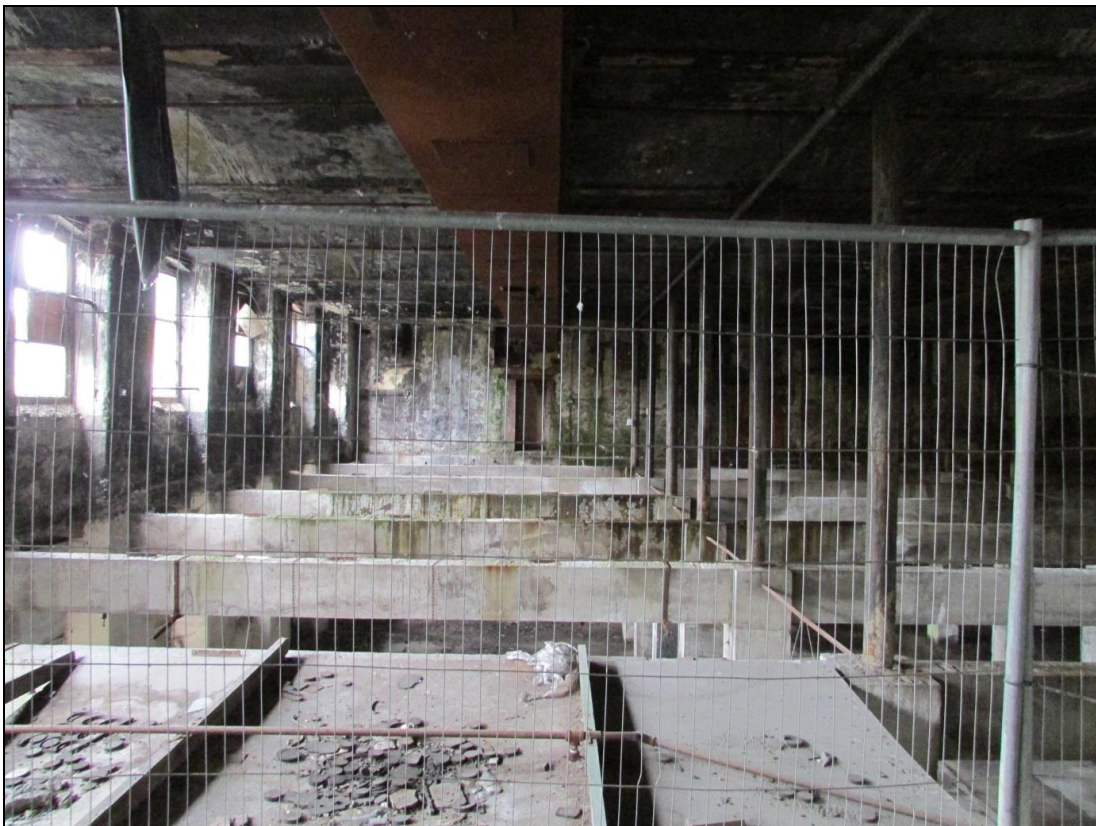
Plate 14 The first-floor in the western half of the mill was removed at a later stage
