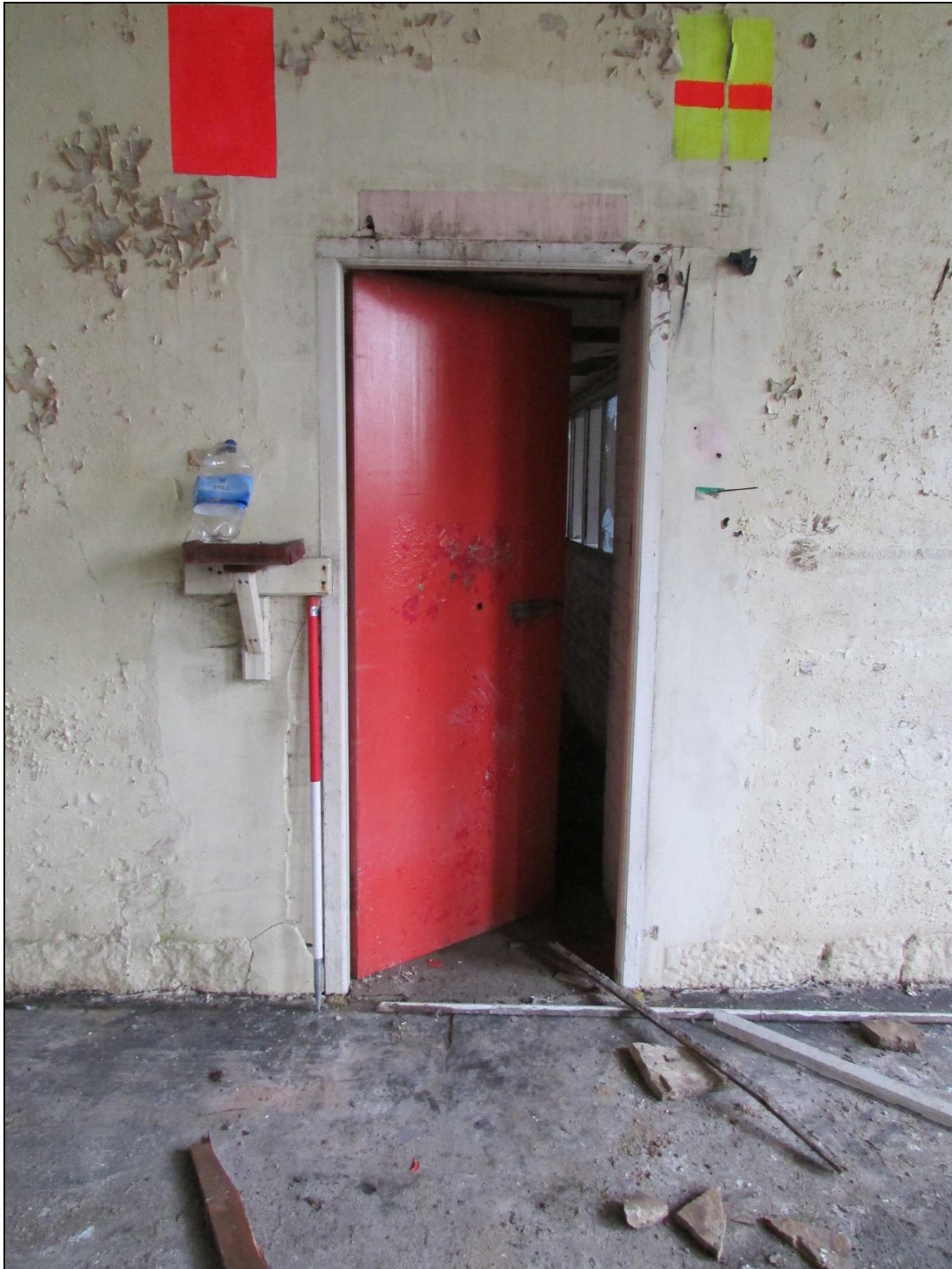
Plate 24 Later inserted entrance into the northern part of the engine house on the second-floor
