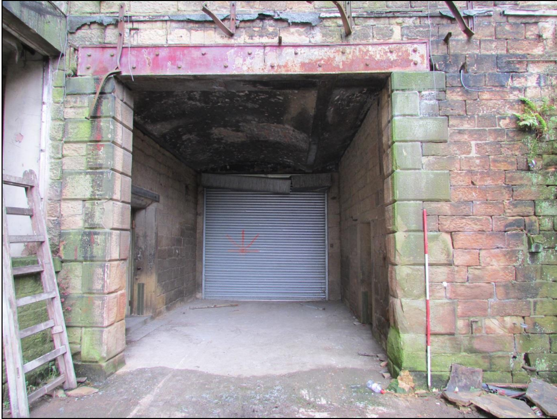
Plate 69 Entrance to covered walkway between the spinning mill and the office block, also showing a later RSJ and fixtures for a possible canopy above
