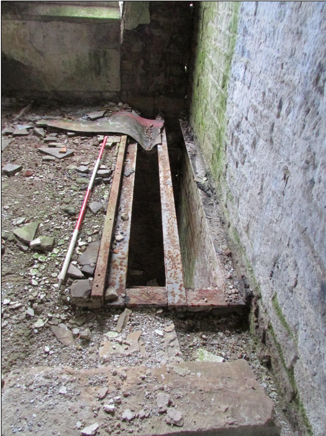
Plate 62 Cast iron lined aperture within the engine house
