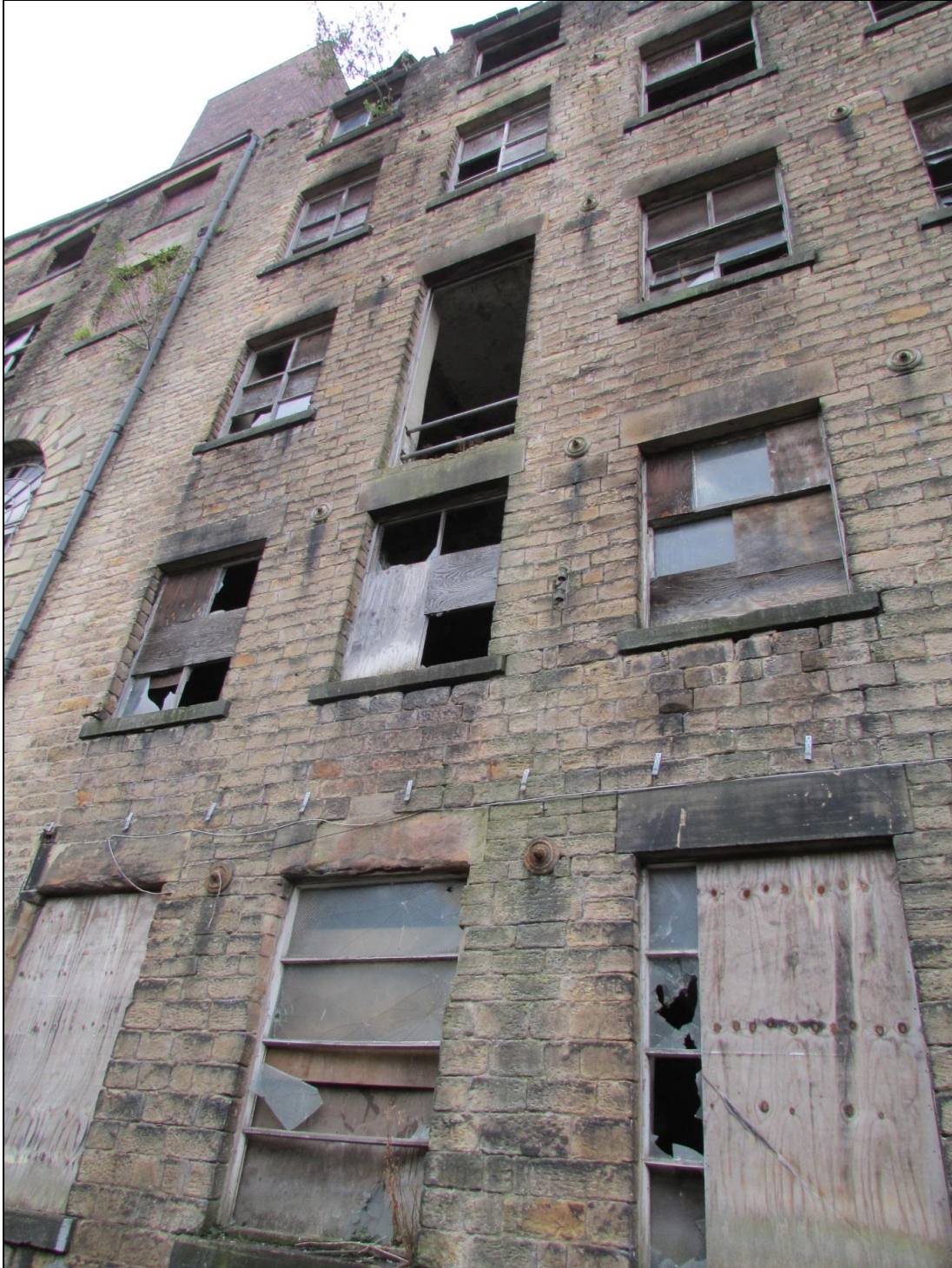
Plate 2 The modified second-floor window (in the middle)
