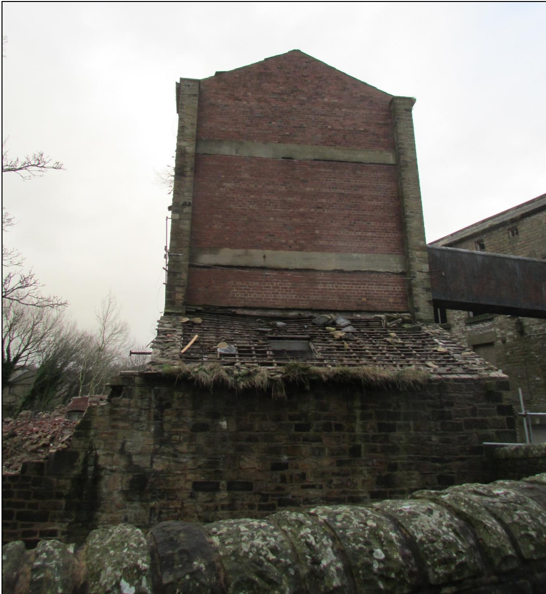
Plate 66 South elevation of the office block, which appears to have been rebuilt along with the stone lean-to on the ground-floor level
