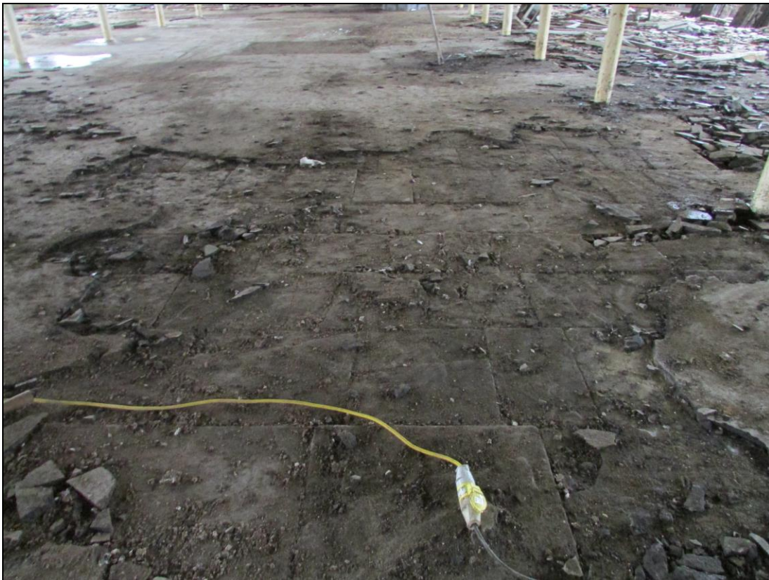
Plate 19 Original stone flagged floor sealed below concrete skim
