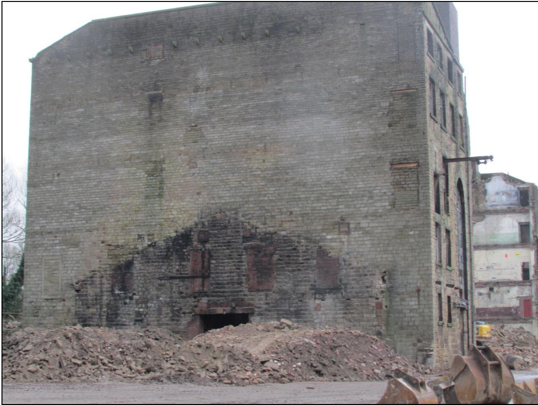
Plate 32 General view of the Engine House western elevation, after removal of the 20th century warehouse (its former position still visible)
