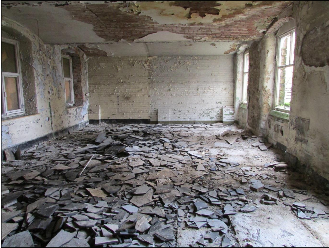
Plate 71 General shot of the Office Block first-floor
