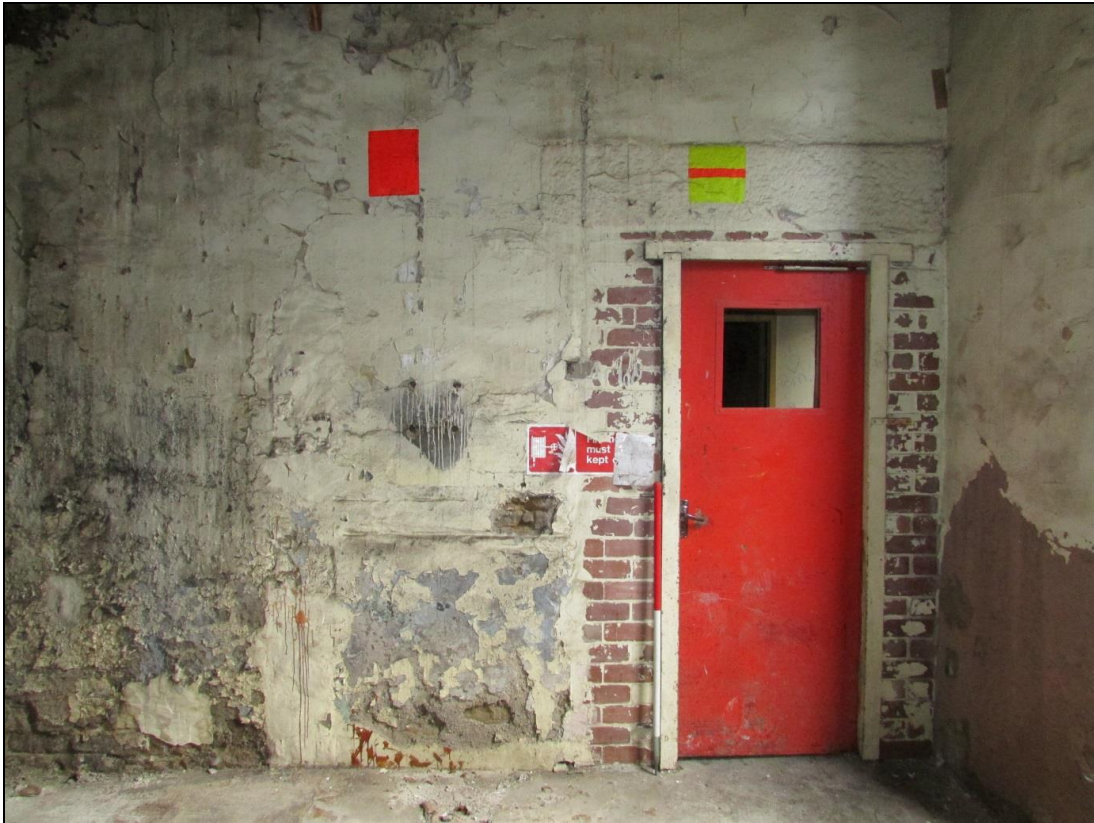
Plate 92 The entrance into the spinning mill from the stair tower, modified and made smaller
