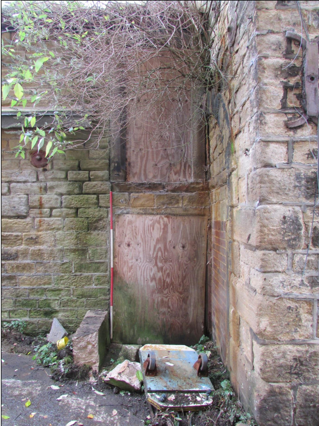
Plate 84 Boarded entrances into the middle shed
