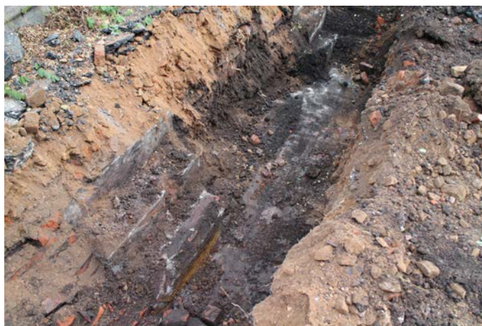
Plate 17: Concrete bases 903 and 904, concrete floor 902 and brick floor 905, looking north
