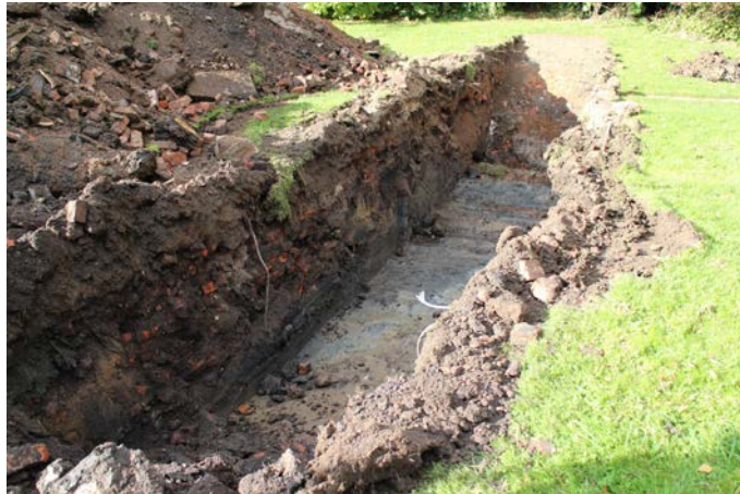
Plate 14: Trench 7, depth of natural clay, looking west
