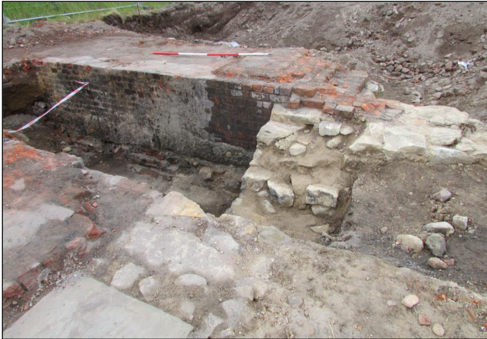
Fig. 7. Wall (019) in foreground with brick structure (009) to rear. Looking west.
