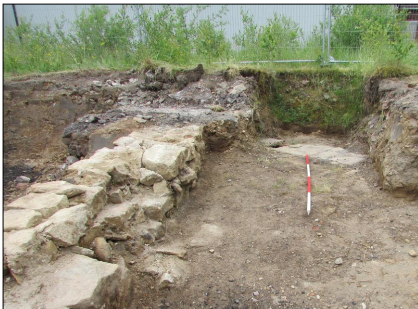
Fig. 5. Eastern side of Room 1 showing culvert found during the evaluation works. Looking east.
