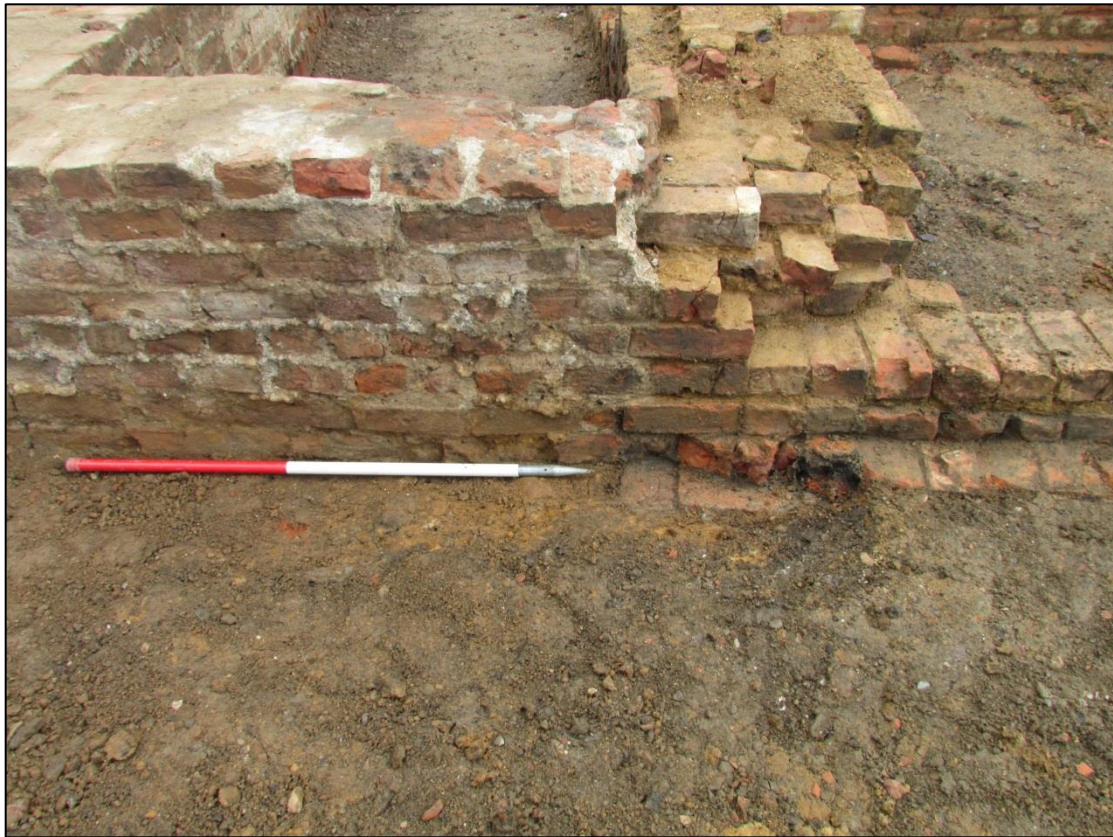
Fig. 26 Wall (097) is of one phase, however two different types of mortar are evident, suggesting that the construction process was carried out in specified stages
