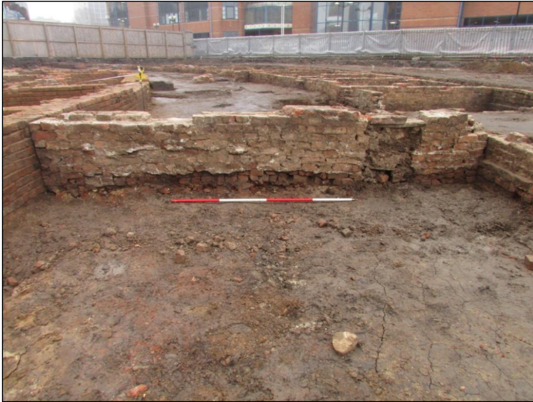
Fig. 16 Wall (074), showing cut [160] for later drain on the right and possible evidence for rebuild above deposit (161)
