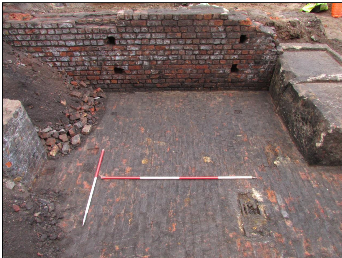
Fig. 24 A total of four slots within wall (042) and five within floor (041) were revealed in Railway Building 2, as shown
