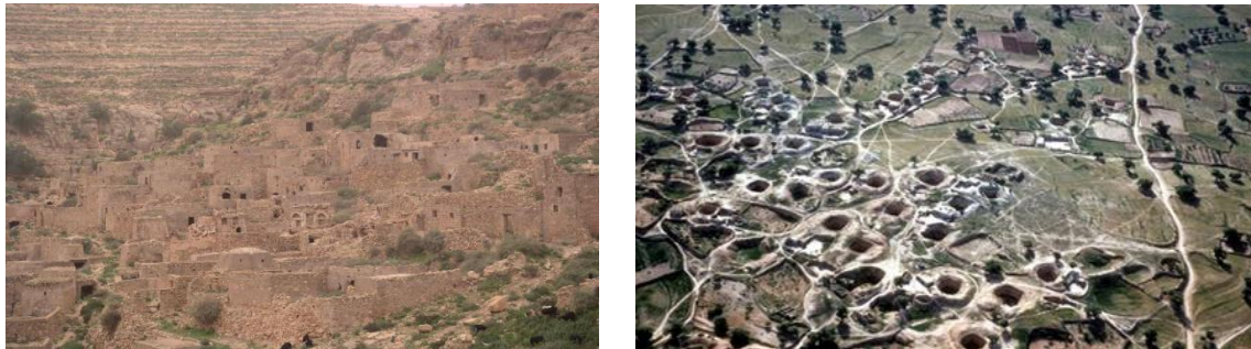
Figure 5: The compact grouping of under and above ground VD in NMR (author's photos)
