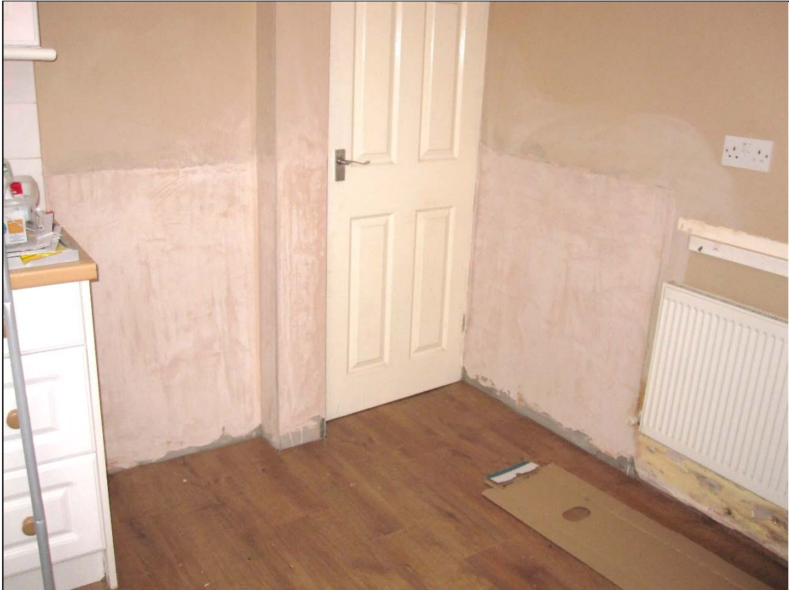
Figure 80: Panels B and C reverse side on completion of plasterwork reinstatement. Reverse side of Panel B (right side of door opening) and Panel C (left side of door opening) after the plaster finish coat had been applied to the low-permeability cement render backing coat.
