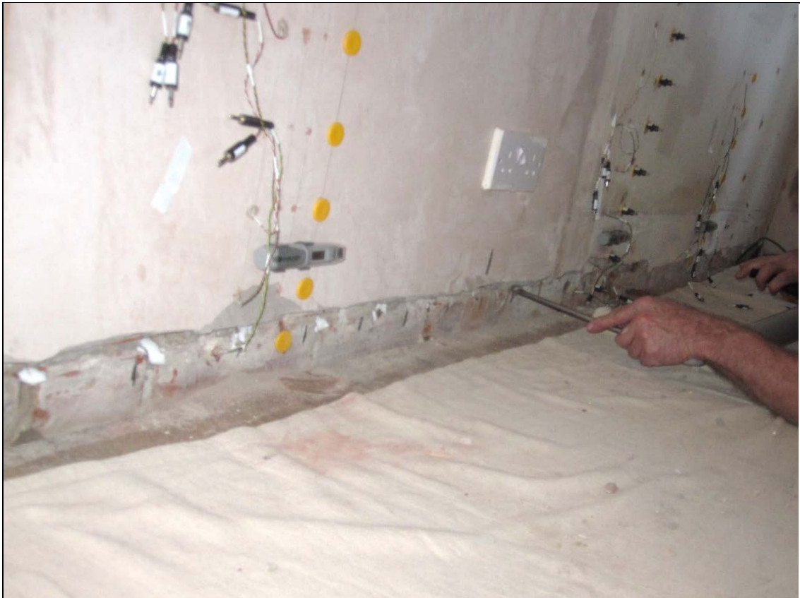
Figure 88: Panel C inserting damp proofing cream into pre-drilled holes.
