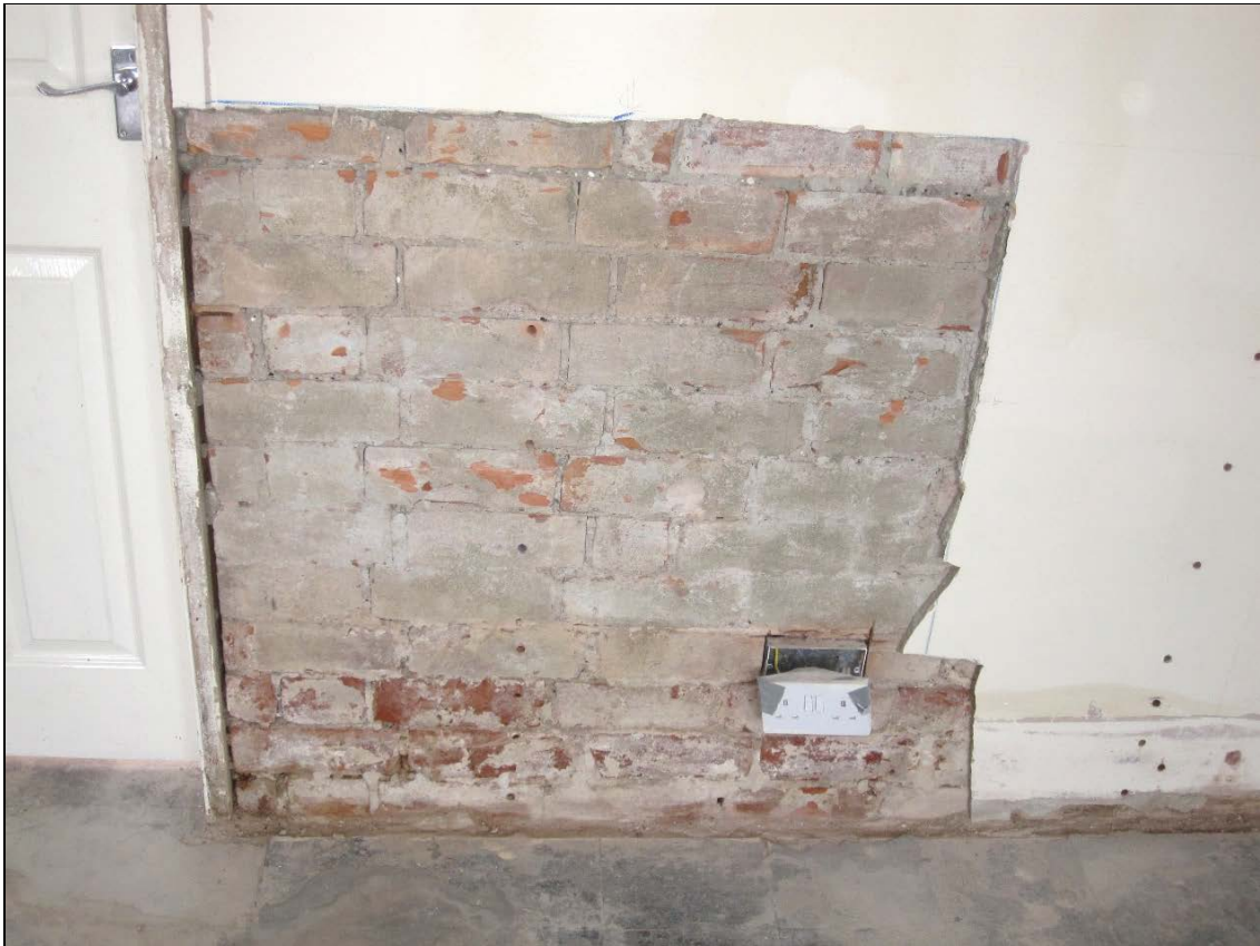
Figure 77: Panel C with existing plaster stripped.
