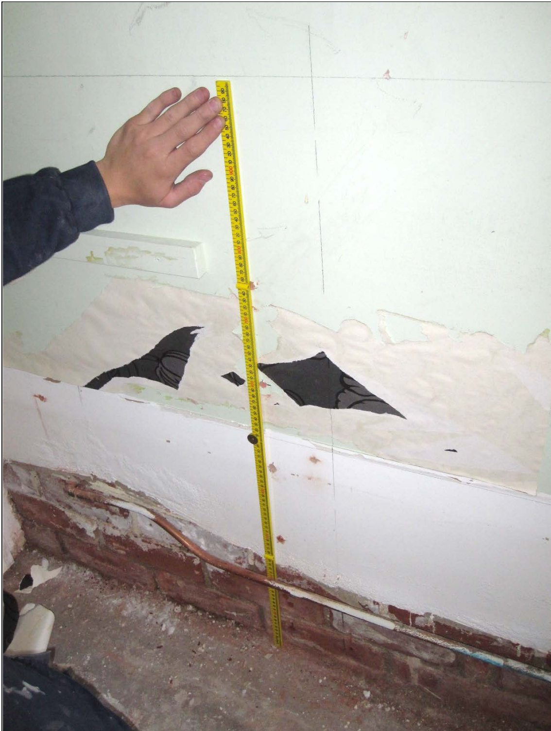
Figure 61: Panel A illustrating drilling pattern for samples required for Stage 2 moisture analysis.
