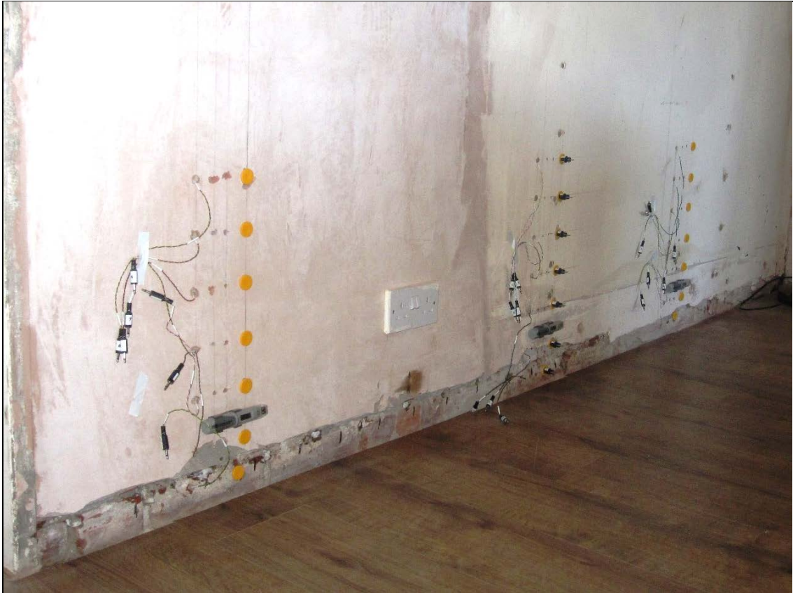
Figure 89: Panels C, D, and E: initial test panel set-up complete.
