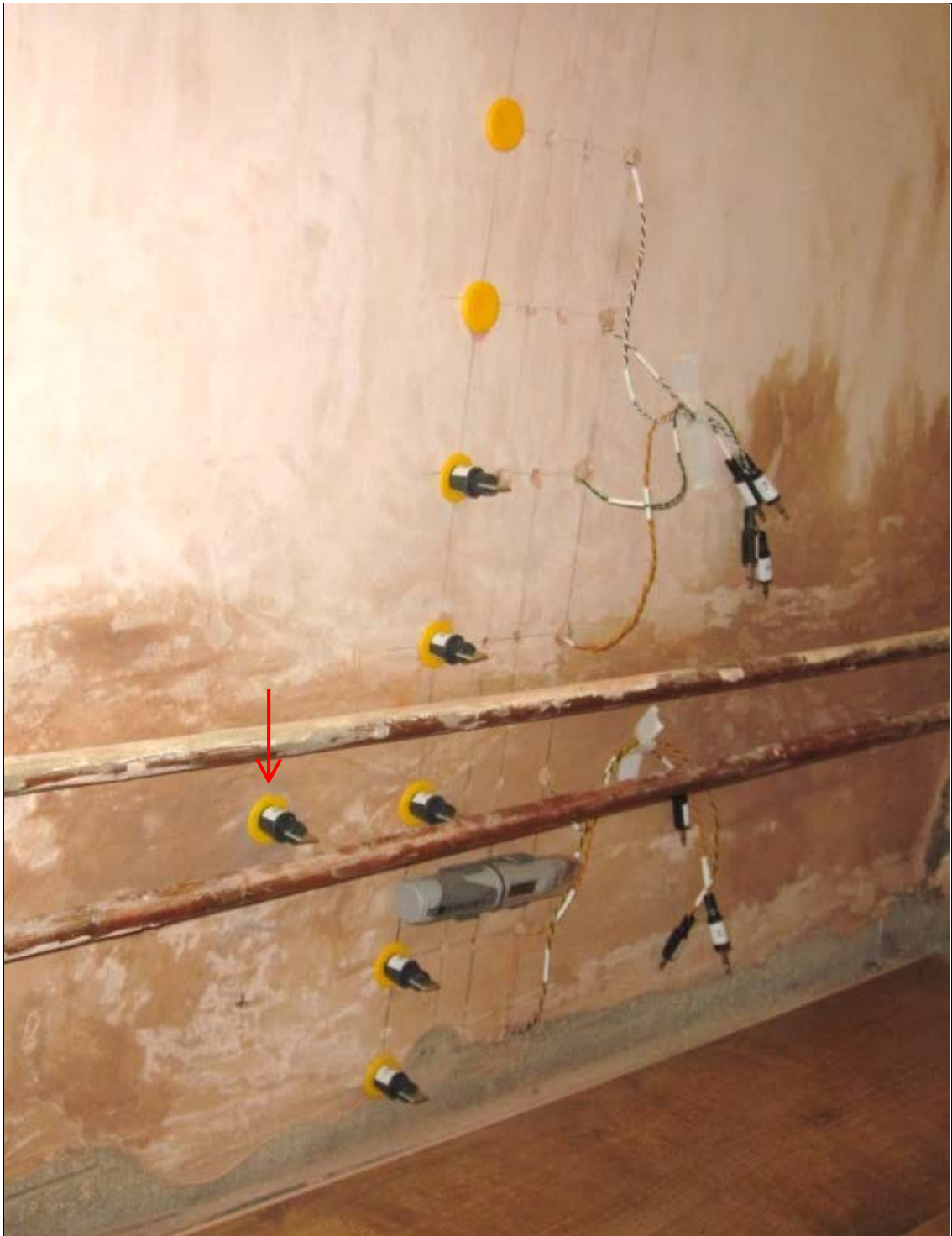
Figure 85: Panel B with additional Humidity Sleeve installed in row 3.
