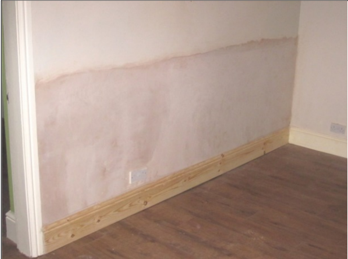
Figure 109: Test Panels C, D, and E following completion of reinstatement works.
