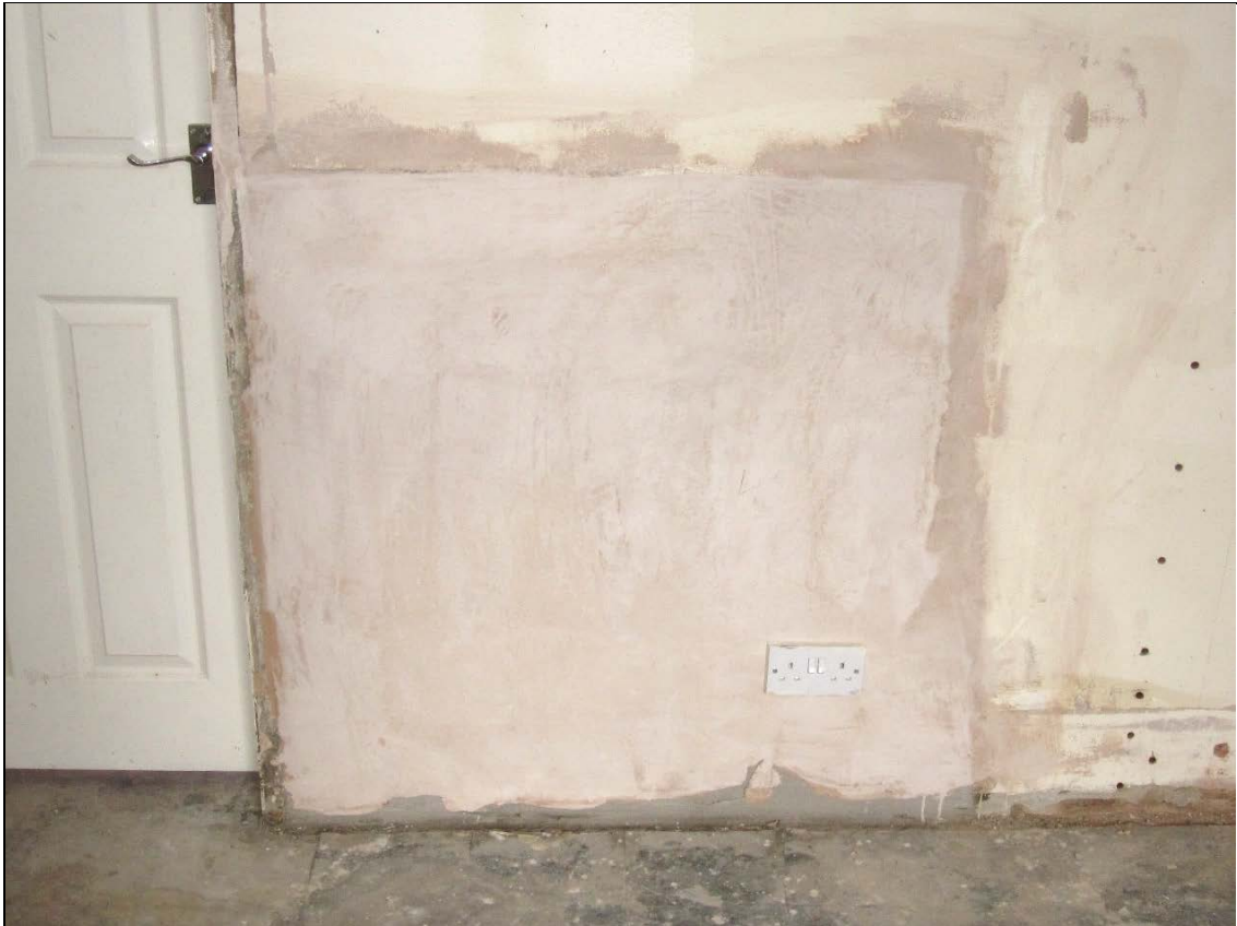
Figure 79: Panel C on completion of plasterwork reinstatement.
