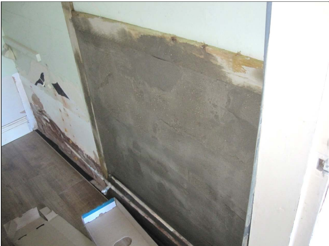
Figure 78: Panel B: low-permeability cement render applied.
