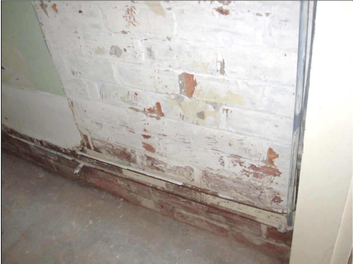
Figure 76: Panel B with existing plaster stripped.
