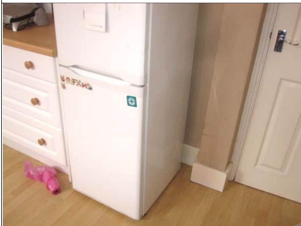
Figure 21: Kitchen front wall, nib wall to side of door. Damp staining extends to 250 mm above floor level.
