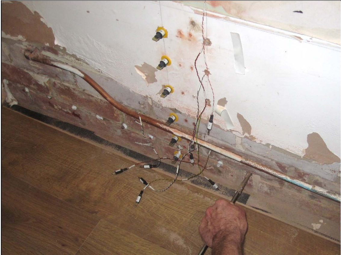
Figure 87: Panel A inserting damp proofing cream into pre-drilled holes.
