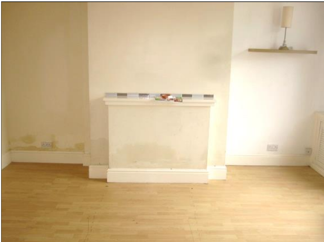
Figure 27: Living room fireplace and alcove walls.
