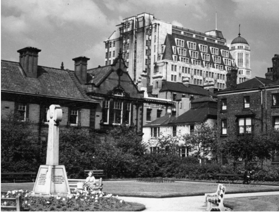
FIGURE 3 St John's Park, Manchester, 1931 © Courtesy of Manchester Libraries, Information and Archives
