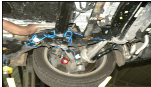
FIGURE 2.20: Physical installation of the accelerometers on the front axle. \circ : An accelerometer mounted on the wheel side.
