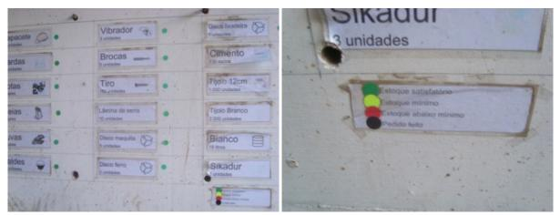
Figure 18-Material/consumables/hand tools stock control board on a construction site
