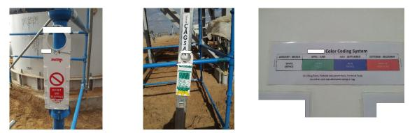
Figure 34-Colour-coded safety tagging (adopted from Tezel et al., 2013)
