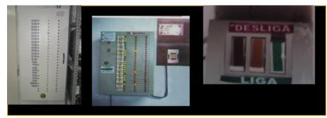
Figure 29-Andon in a high-rise building construction project
