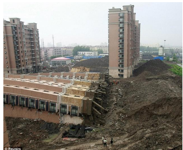
Fig. 2: Collapse of 13-Storey Building [4].
