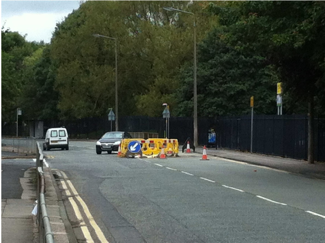
Figure A.11: Pictures showing Site 14
