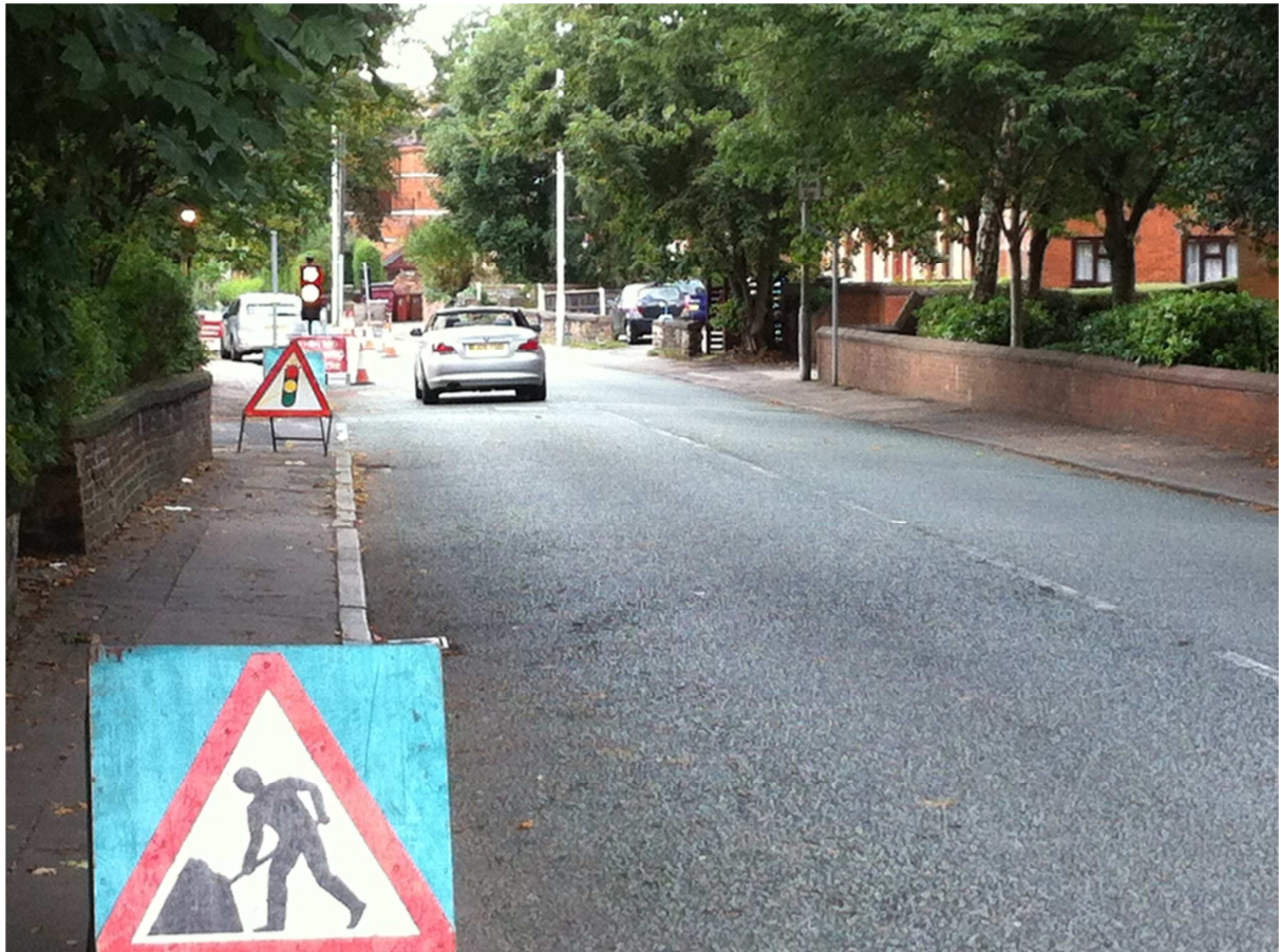
Figure A.15: Pictures showing Site 16
