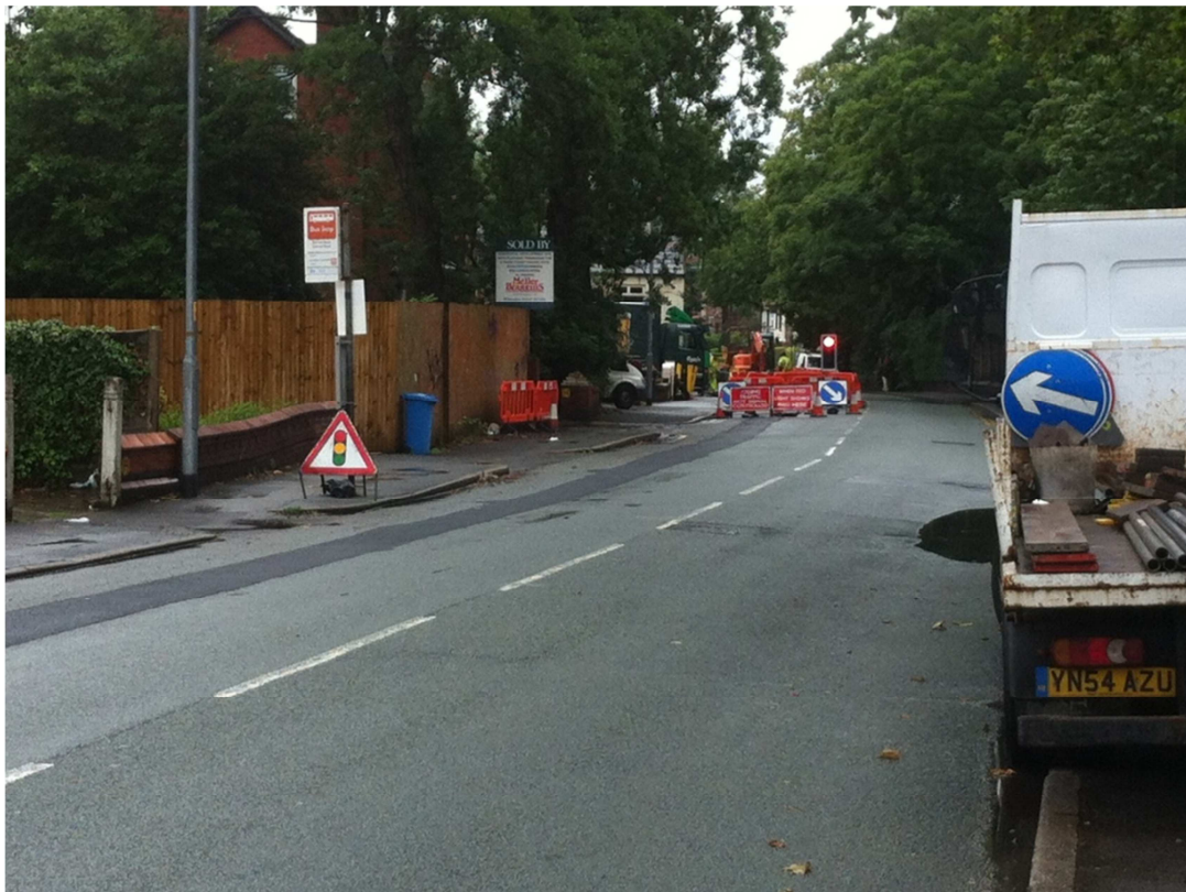
Figure A.4: Pictures showing Site 12
