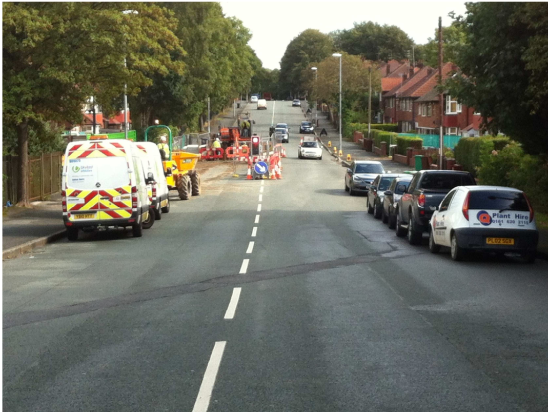
Figure A.21: Pictures showing Site 18
