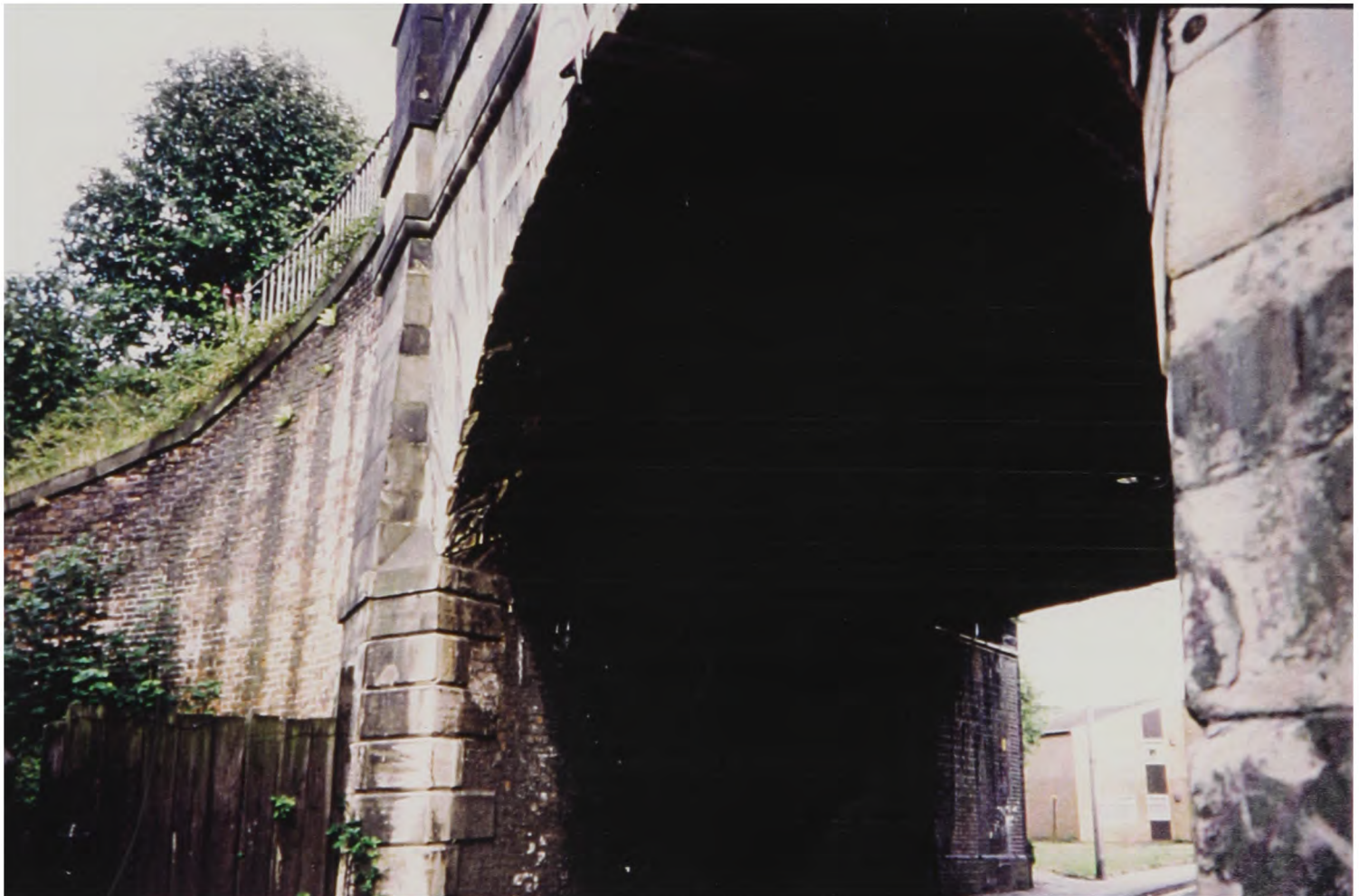
Plate 1.4 Edge detail adopted on skewed arch bridges
