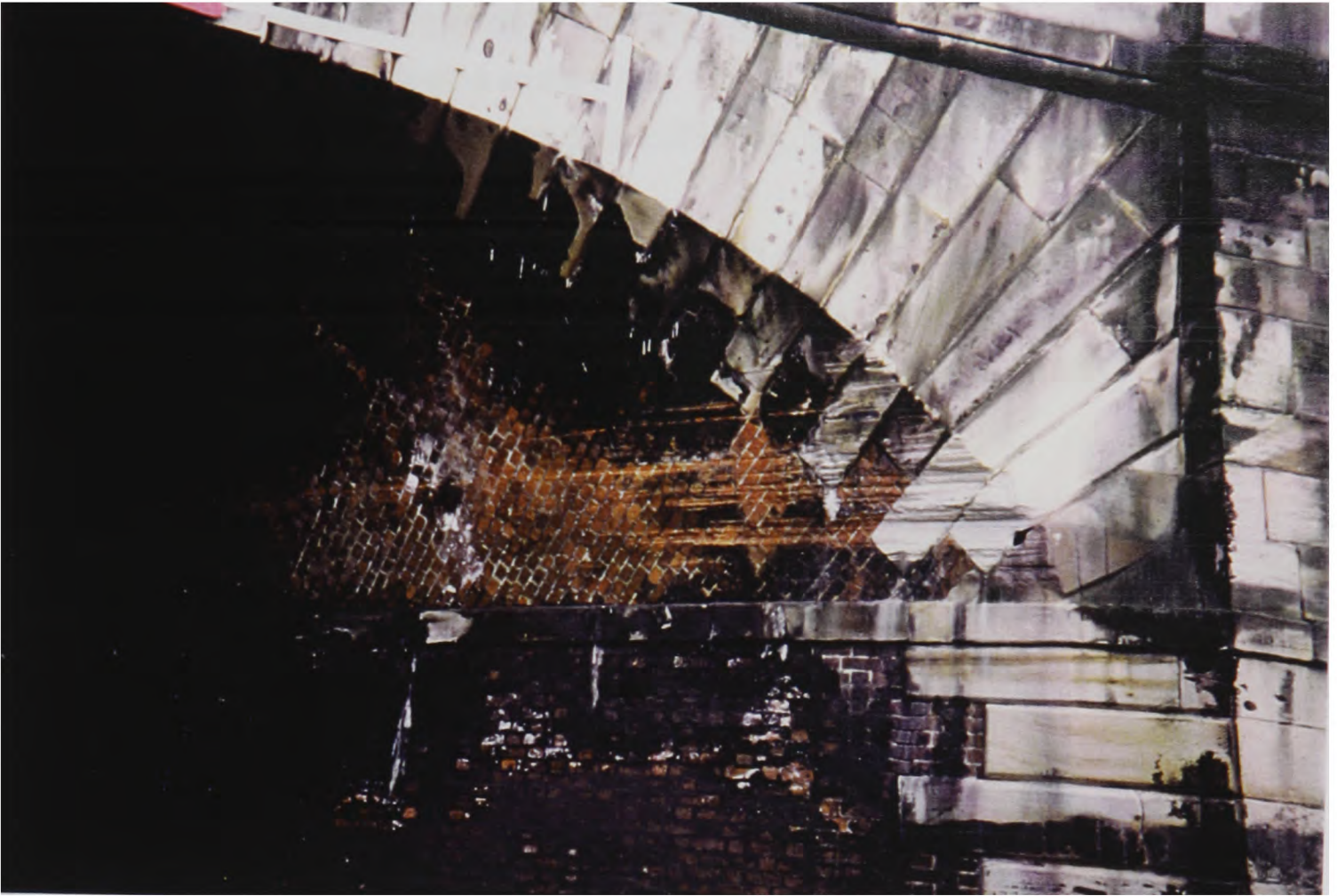
Plate 1.3 Edge detail adopted on skewed arch bridges
