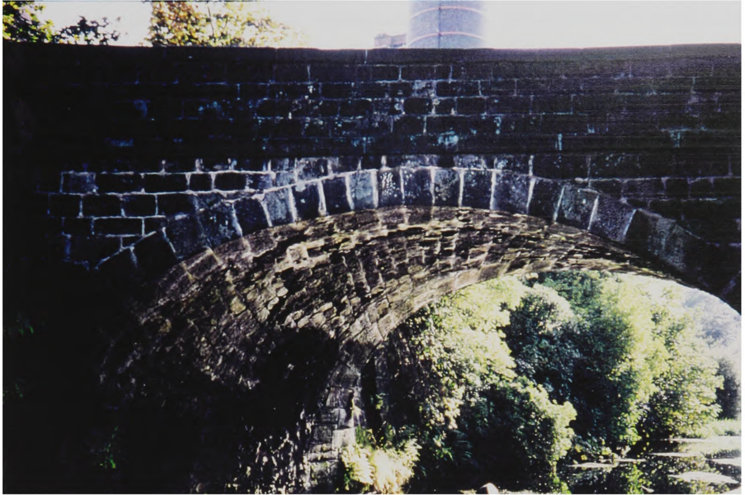
Plate 1.1 Jessop's Bridge: the first skewed arch
