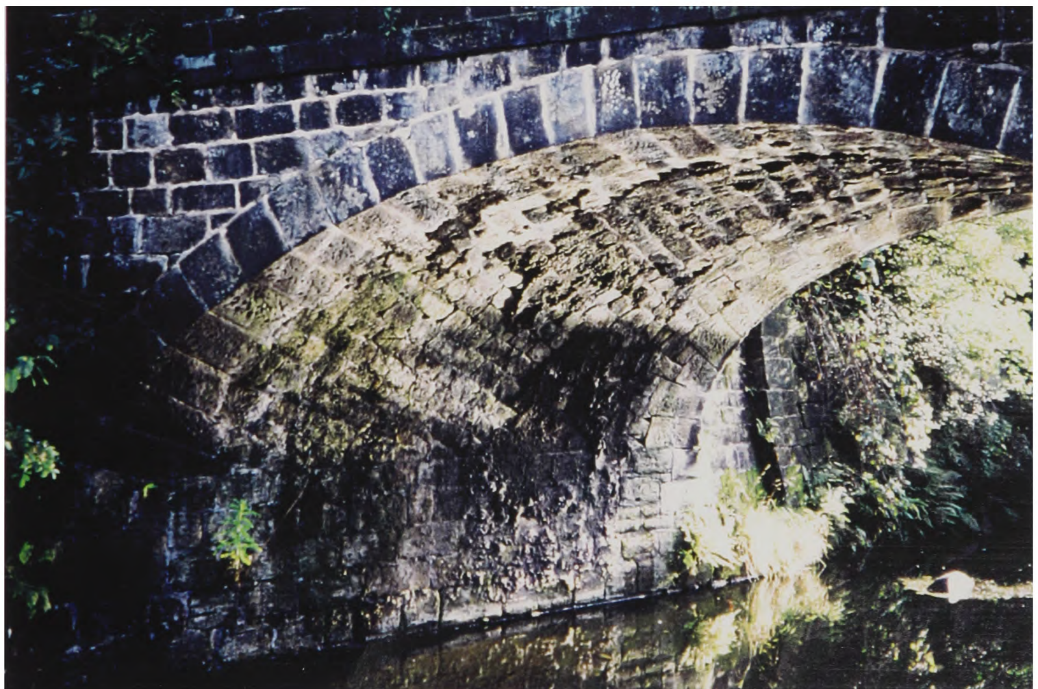
Plate 1.2 Jessop's Bridge: the first skewed arch
