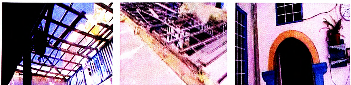
Figure 6. 46: The courtyard and the wood skeleton used to cover the courtyard when it is raining. This figure also shows the openings type
