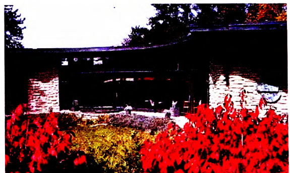
The north view
