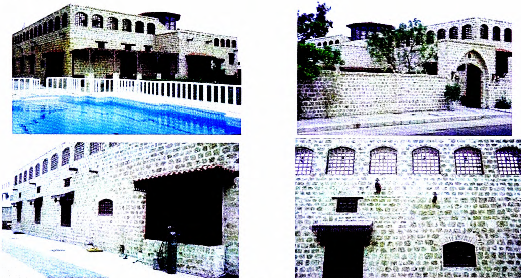
Elevations showing the use of local materials such as stone and the parapet wall with mashrabyia - wall detail with small windows that protected by shading device.
