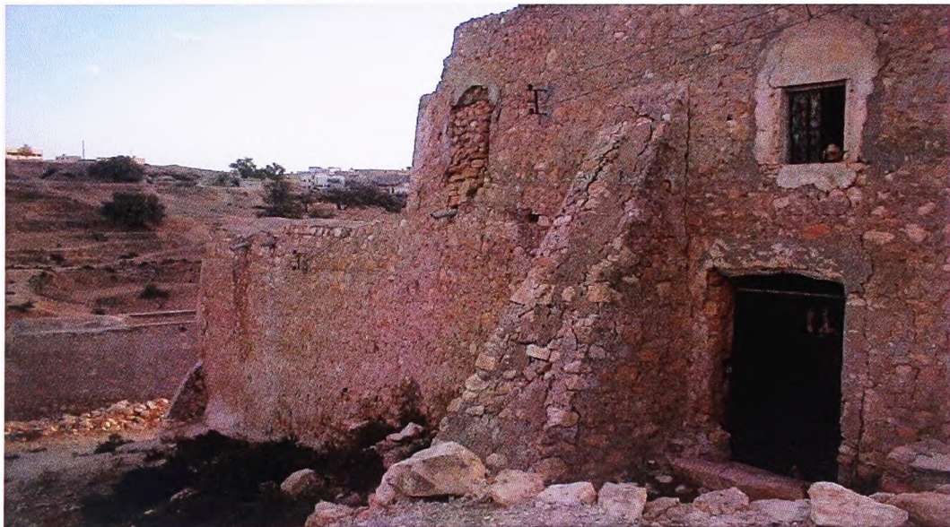
Figure 4.43 Figure 4. 43: Inclined walls supported the other walls from outside. Source: Madi (2005)
