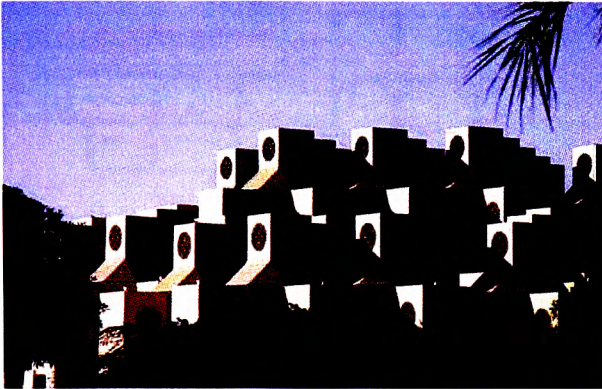
Figure 3. 54: Emphasizing natural ventilation by using wind towers in the education technology centre.
