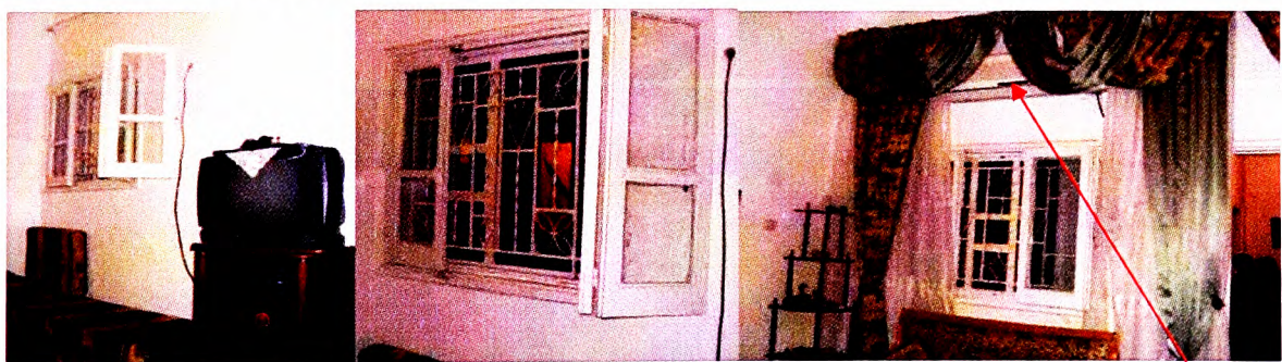
Figure 6.53: The window and the equipment in the living room and the position of the air conditioning located in the main hall.
