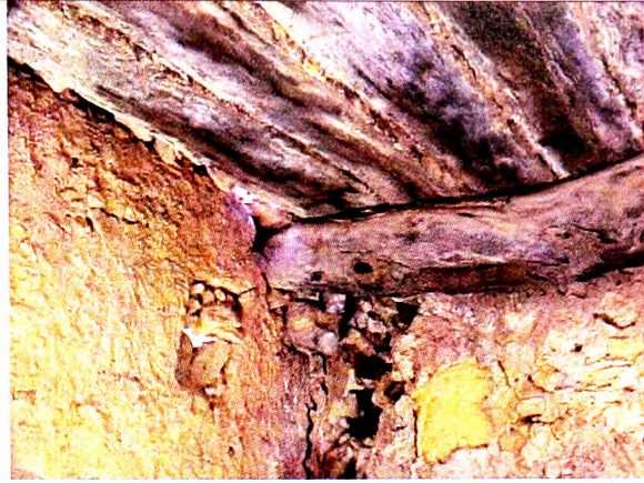
Figure 4. 45: Using palm-tree trunks and olive branches in flat roof.
