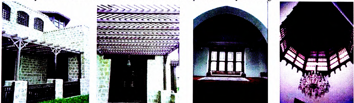
Using the entry porch to provide shade.
