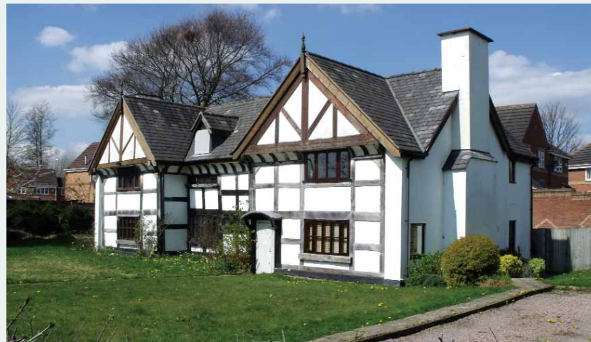
Fig 18: Kersall Cell, Salford. A cruck hall of c 1515 which was expanded in the later sixteenth century by the addition of two box-framed cross-wings.
