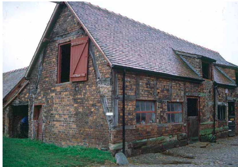
Fig 21: The Bent Old Farmhouse, a late medieval cruck-framed farmhouse replaced by a box-framed farmhouse around 1600. By the eighteenth century the old farmhouse was being used as barn and the wattle and daub walls were replaced by brick.
