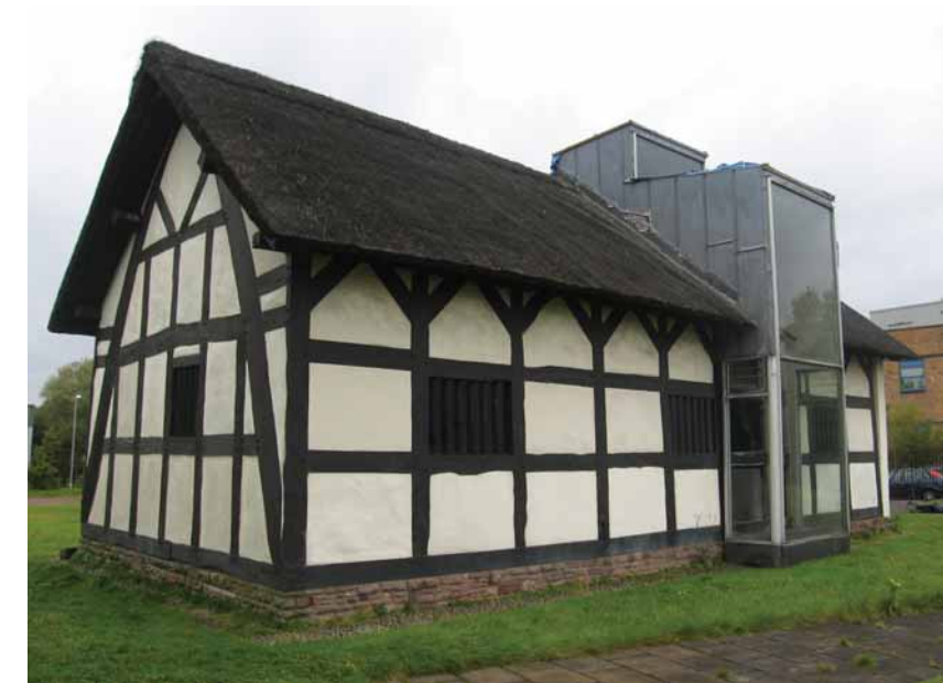
Fig 1: Newton Hall is a late medieval timber-framed cruck hall built by the Newton family.
