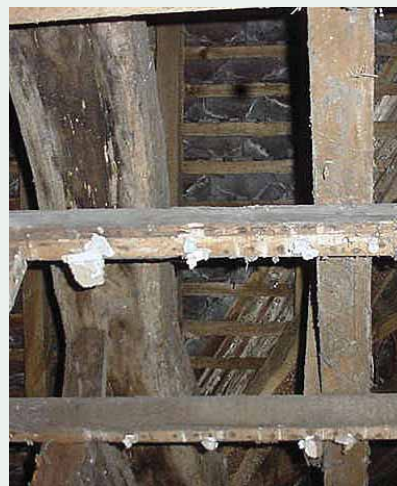
Fig 7: Re-used cruck blades in the roof of Paddock Lane Cottage, Warburton, rebuilt in 1737.
