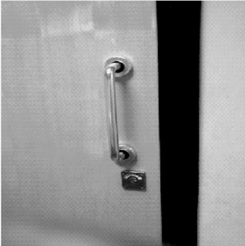
Fig 2: Same door with metal handle on the other side
