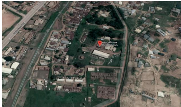
Figure 4:1 Aerial View of the case study Power Plant
