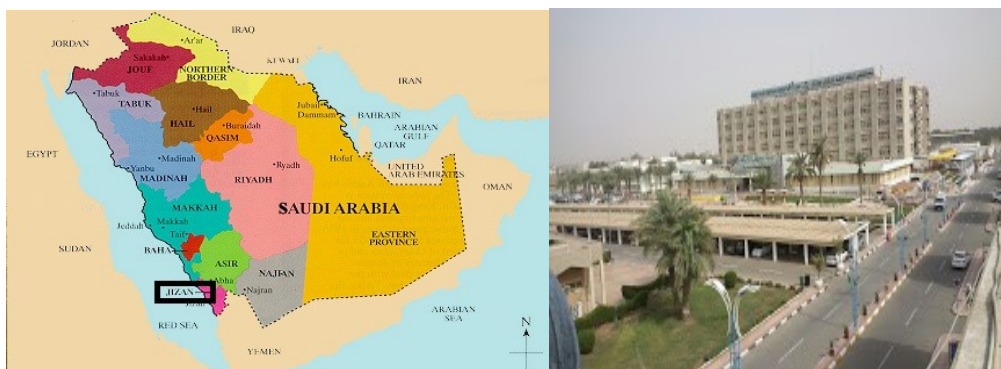
Figure 5.5 King Fahad Central Hospital – Jizan – KSA
