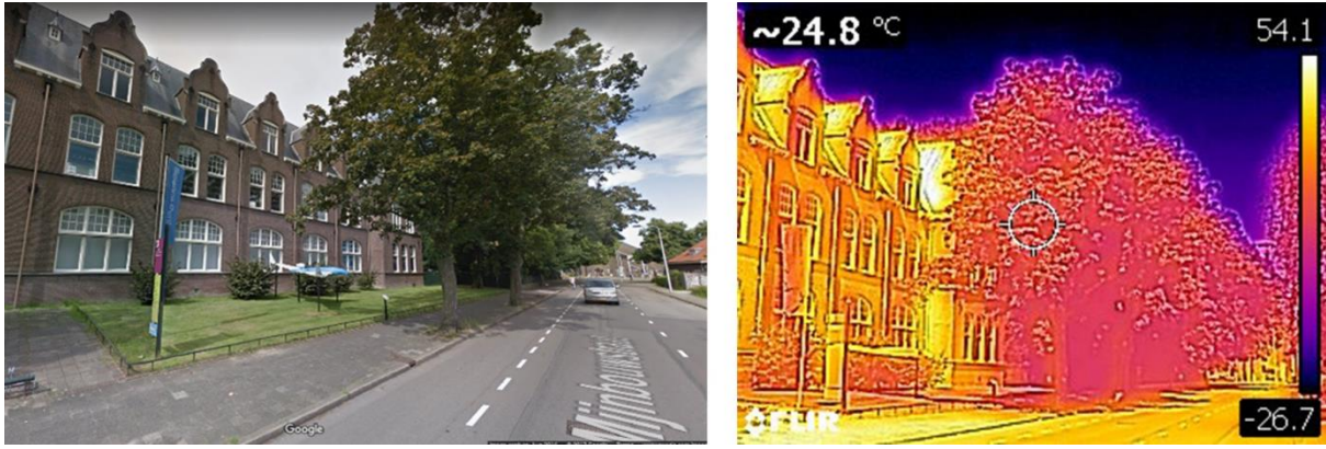
Figure 2: A view of the eastern façade of the Science Centre building (left); and the surface temperature of the façade. The emissivity was set to 0.90.
