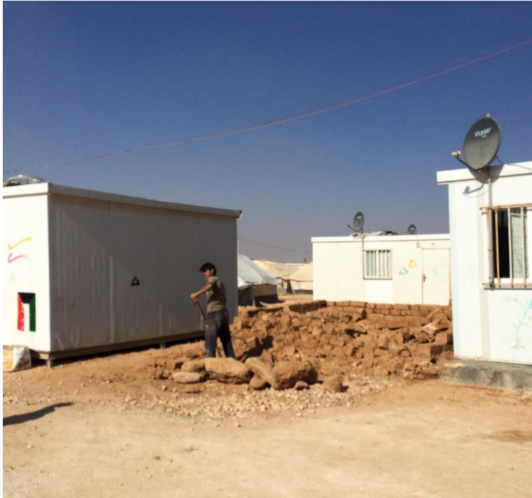
Figure 5.2: A shelter demolished by local government in the Al Za'atari camp
