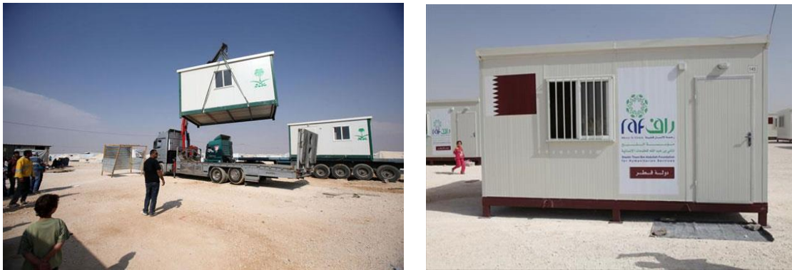
Figure 2.13: Examples of prefabricated caravans in the Al Za'atari (Source: www.google.jo )
