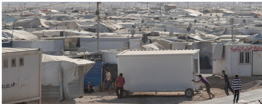
Figure 2.12: Prefabricated shelters in the Al Za'atari camp (Source: www.google.jo)
