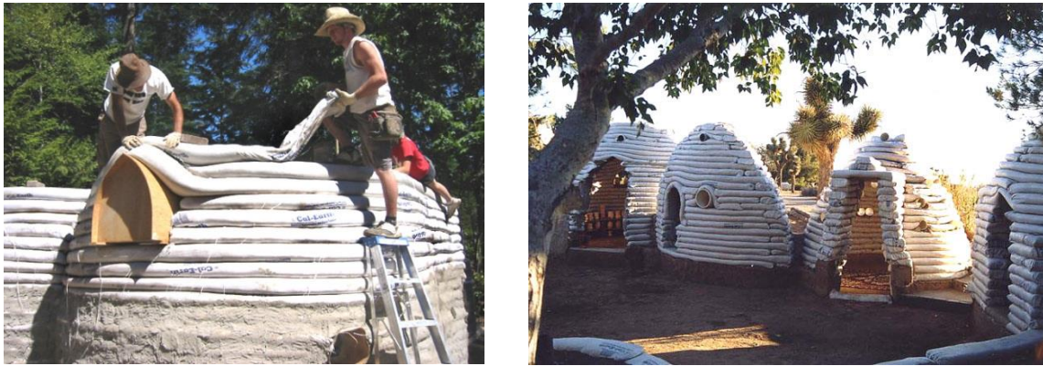
Figure 2.17: Sandbag shelter in Iran (Source: www.earthbagbuilding.com )
