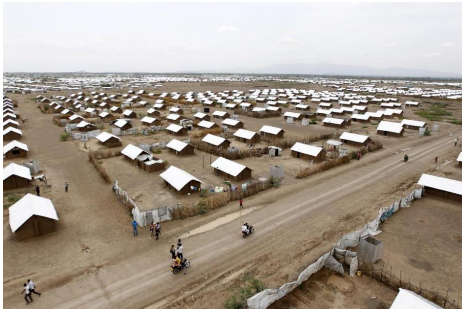
Figure 2.2: Constructed houses at the Kakuma refugee camp (Source: www.reuters.com)
