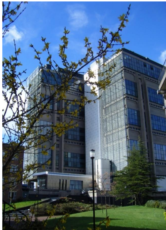
Figure 11. The Grade 2 listed Muirhead Tower, built in 1963, University of Birmingham, March 2014.
