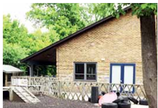
Good: abundant sun heat but with external shading devices, e.g. canopy (top), overhangs (bottom)
