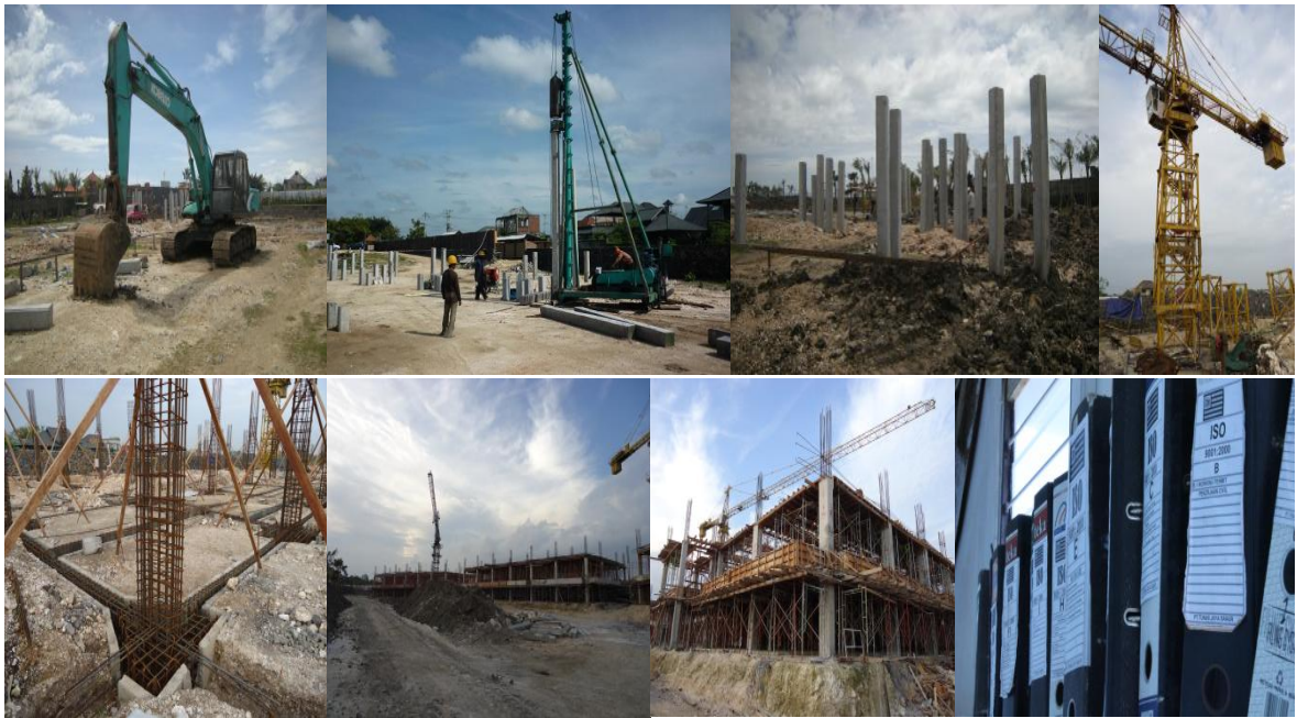
Figure 4-7: Mobilisation and Substructure Activities
